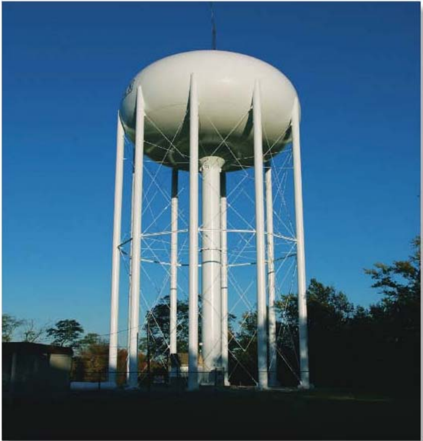
The columns used to support this water tank are braced at their mid-height in order to reduce their chance of buckling.
