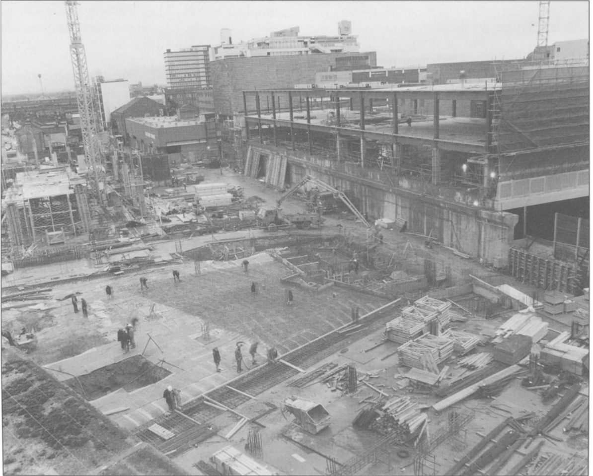
Figure 7.7 The Exchange Shopping Centre, Ilford, under construction (Source: Norwich Union)
