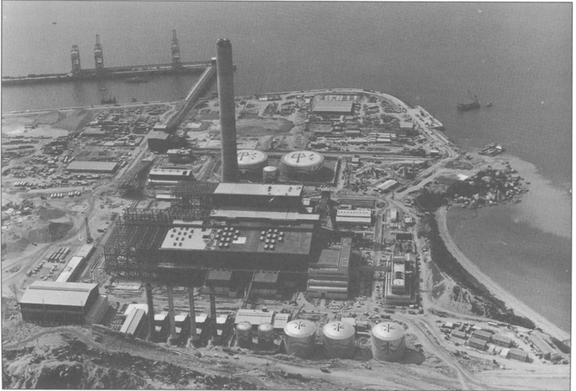
Figure 8.34 Castle Peak 'A' Power Station, Hong Kong (Source: L.G. Mouchel & Partners)
