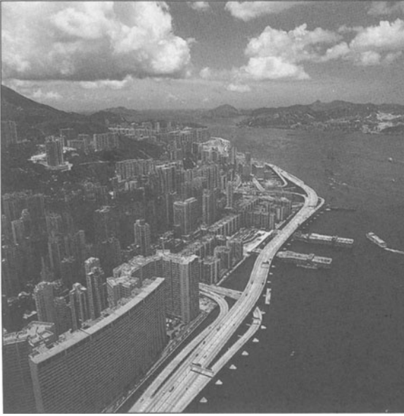
Figure 3.7 Island East Corridor, Quarry Bay, Hong Kong (Source: Hong Kong Territory Development Department)
