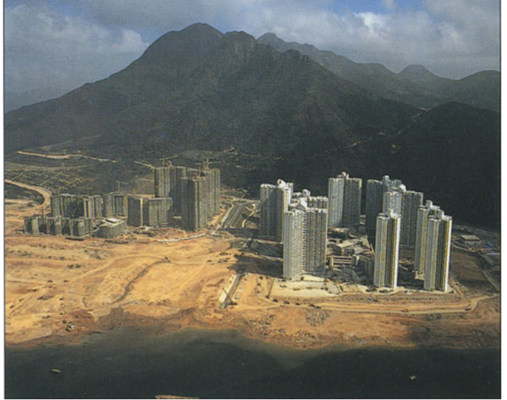
35 Sea reclamation for Ma On Shan extension, Sha Tin New Town, Hong Kong (Source: Territory Development Department, Hong Kong)
