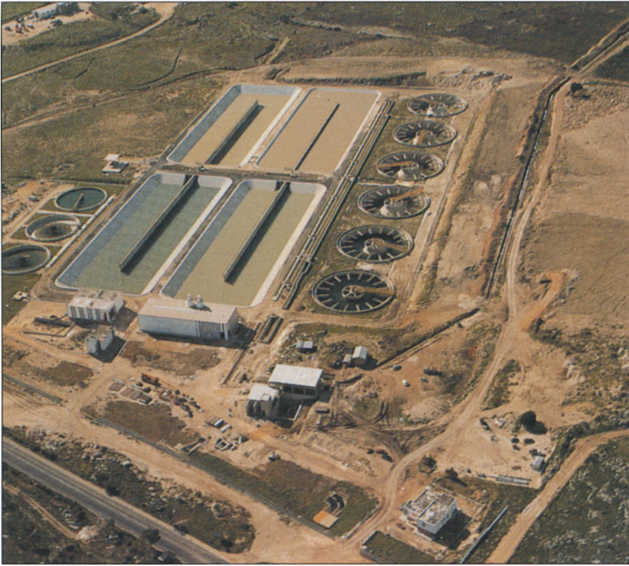
16 Syracuse water treatment works, Sicily (Source: Watson Hawksley)
