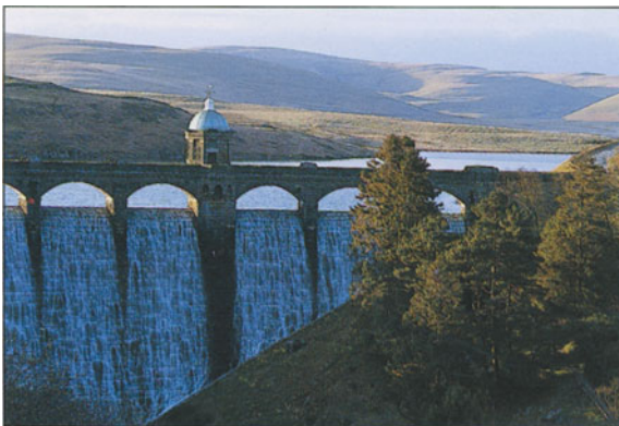
14 Elan Valley (Craig Goch) Reservoir (Source: Severn Trent Water)
