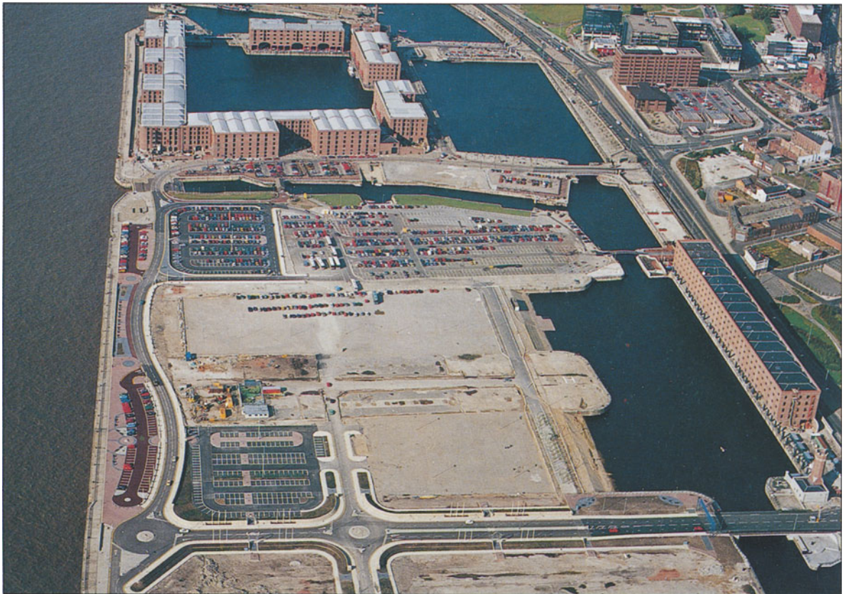
26 Albert Dock and Wapping Warehouse, Liverpool, after renovation (Source: Merseyside Development Corporation)
