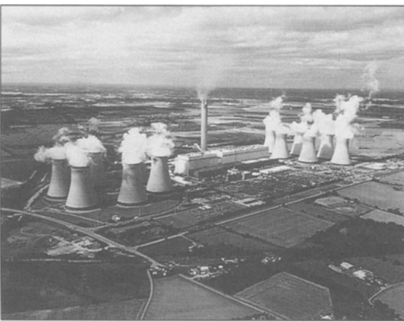
Figure 8.32 Drax Power Station (Source: Ove Arup & Partners)
