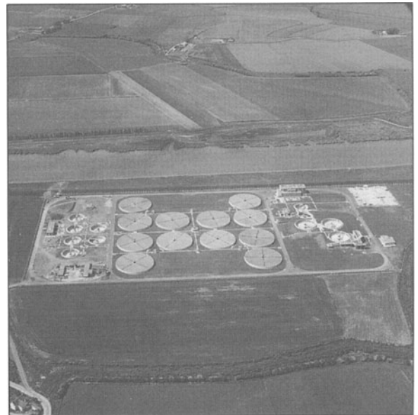
Figure 4.22 Boston sewage treatment works, Lincolnshire (Source: Binnie & Partners)
