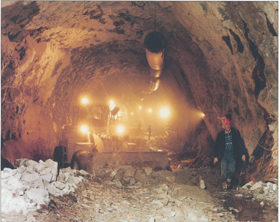
9 A55: Penmaenbach Tunnel (Source: Travers Morgan)
