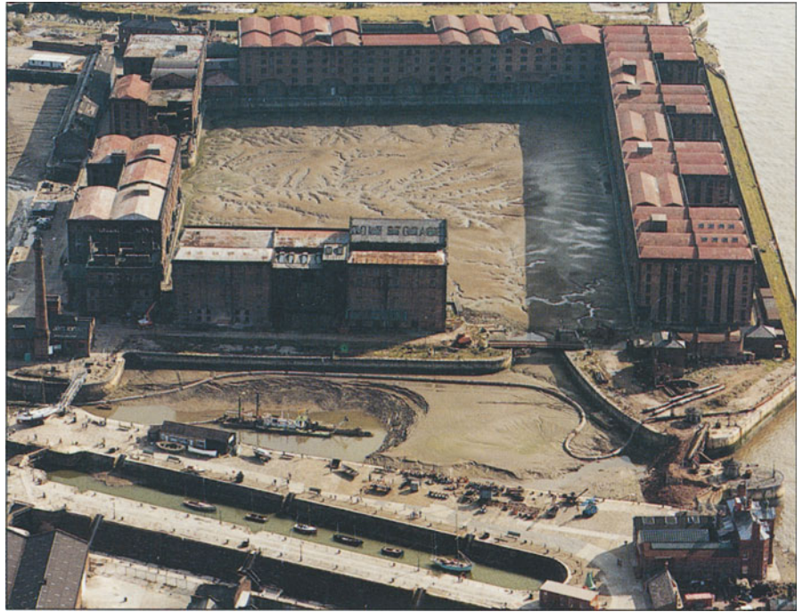
25 Albert Dock, Liverpool, before restoration (Source: Merseyside Development Corporation)
