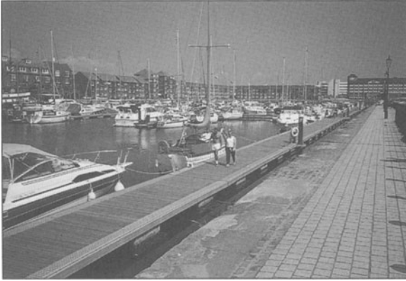
Figure 7.15 Swansea Maritime Quarter, main dock basin and surrounding buildings (Source: Swansea City Council)
