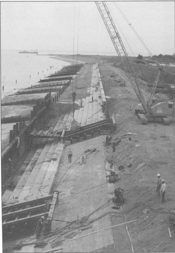
Figure 8.7 Sea defence work under construction, Felixstowe (Source: W.A. Dawson Ltd)
