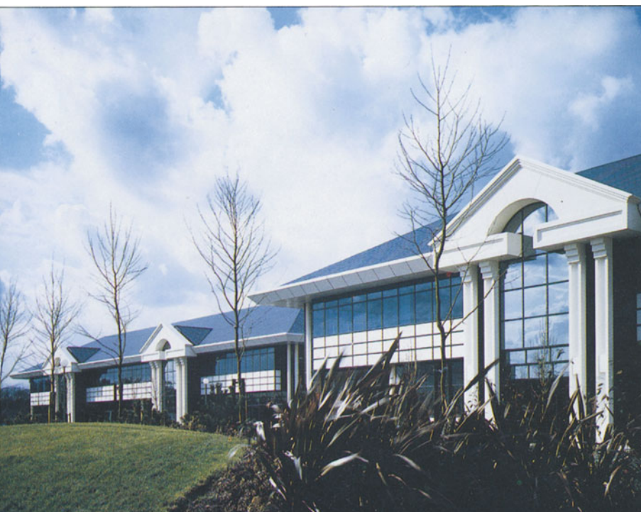
24 Watchmoor Business Park, Camberley, landscaped buildings (Source: London & Metropolitan)
