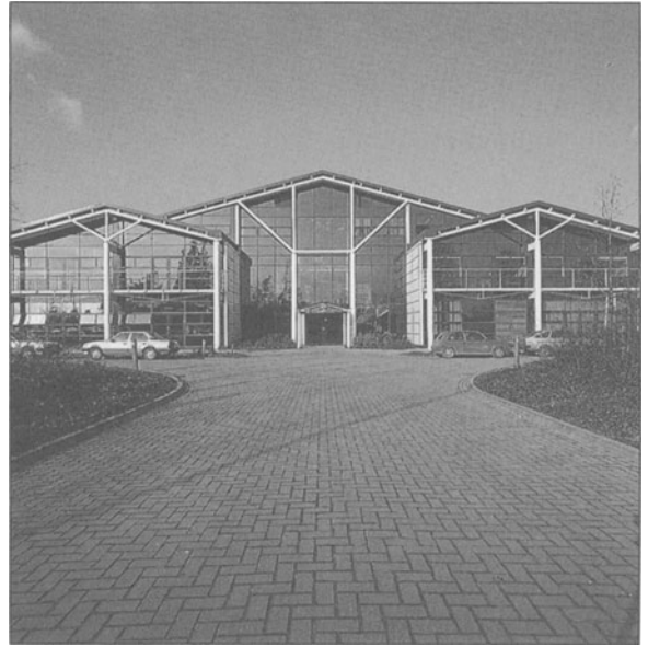
Figure 7.12 St John's Innovation Centre, Cambridge (Source: Shepherd Construction Ltd)
