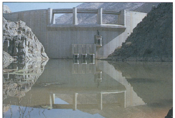
15 Mudhiq Dam, Saudi Arabia, in operation (Source: Binnie & Partners)
