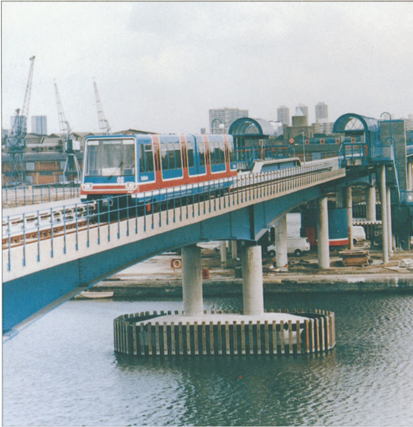
1 London Docklands Light Railway (Source: W. S. Atkins, Consultants Ltd)
