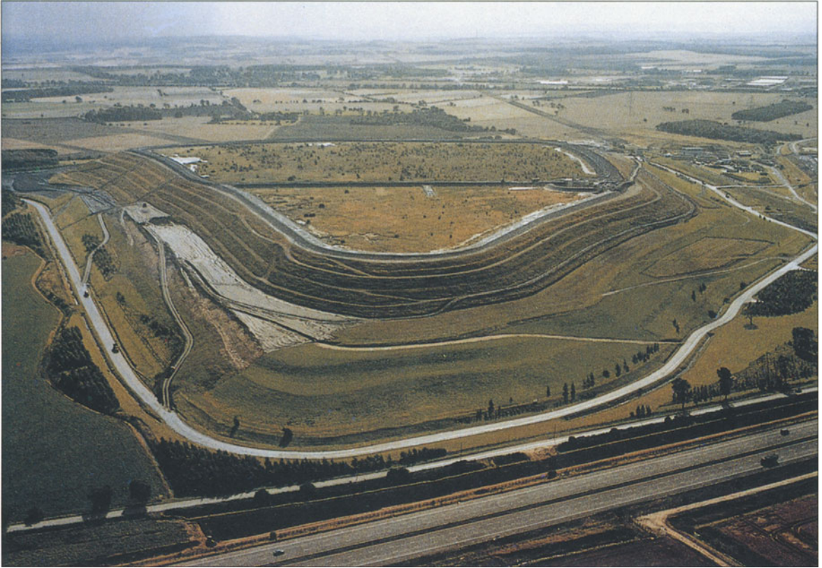
41 Gale Common, ash disposal from power stations (Source: Rendel Palmer & Tritton)
