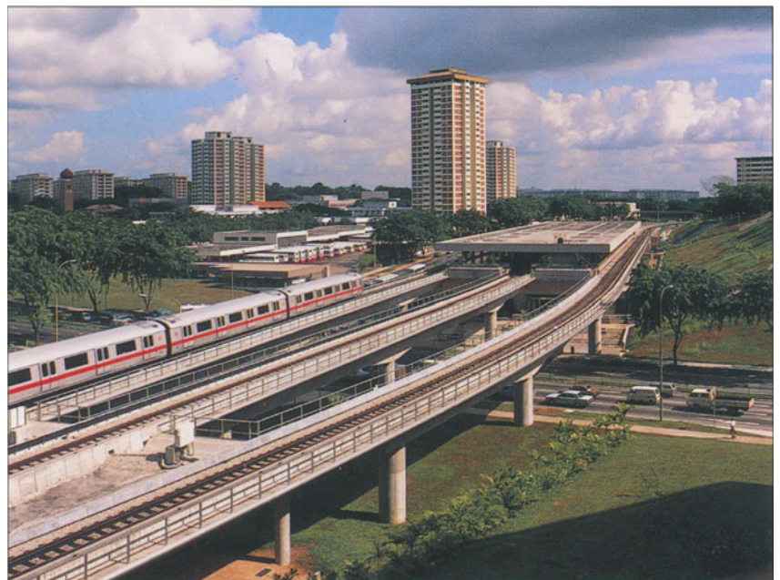
2 Singapore Mass Rapid Transit Train and Ang Mo Kio Station (Source: Sir W. Halcrow & Partners Ltd)
