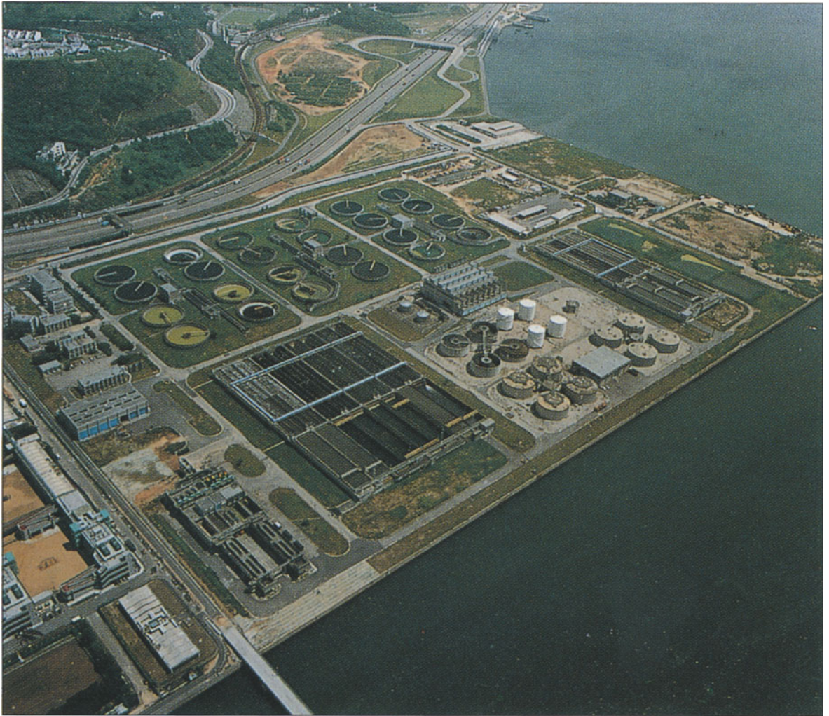
13 Sha Tin sewage treatment works, Hong Kong (Source: Watson Hawksley)
