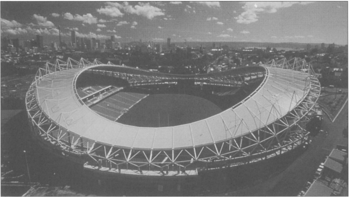
Figure 8.27 Sydney Football Stadium (Source: Ove Arup & Partners)
