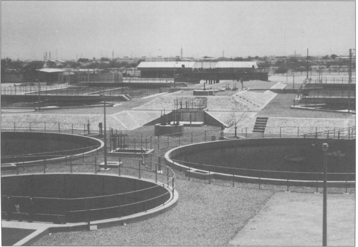
Figure 4.26 MAM sewage plant, Oman (Source: W.S. Atkins)
