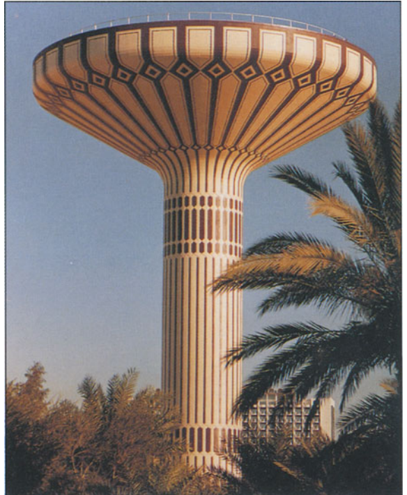
18 Dubai water tower, Jumeirah, United Arab Emirates (Source: Watson Hawksley)
