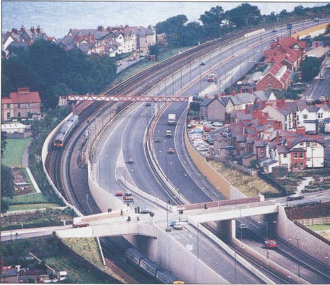
8 A55: Rhos Interchange (Source: Travers Morgan)
