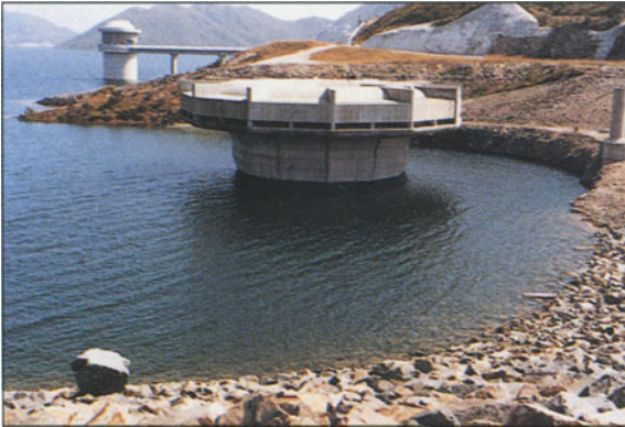
17 High Island Dam and Reservoir, Hong Kong (Source: Binnie & Partners)
