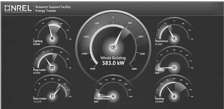
Energy Dashboard Highlighting Current Demand and Various End Uses (Sub Metered) Source: nrel.gov
