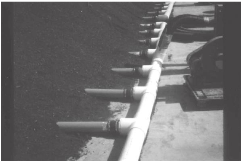
FIGURE 7.15 Aboveground perforated pipe assembly system, showing manifold and blowers.
