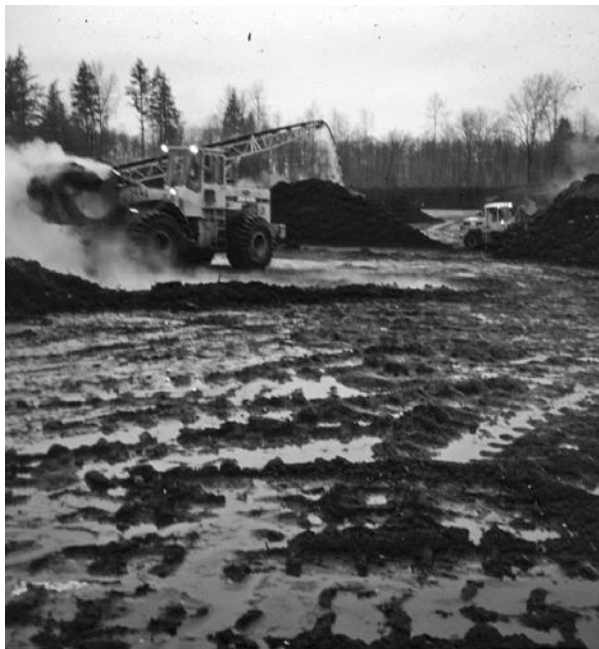
FIGURE 14.4 Runoff and leachate on a composting pad.
