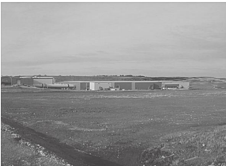
FIGURE 3.2 Edmonton, Canada, municipal solid waste and biosolids composting facility. The rotating drums are in the front of the composting building.
