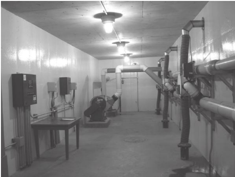
FIGURE 6.13 Fan room for the aerated bins in Granby, Canada. (Courtesy of ECS, Seattle, Washington.)
