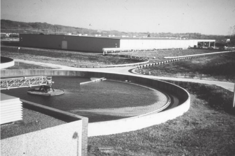
FIGURE 6.7 An enclosed ASP facility in Davenport, Iowa. The large pipe along the wall is the air handling system for the biofilter.
