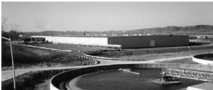
FIGURE 7.2 Davenport biosolids composting facility. Adjacent to the facility is the biofilter for odor control.
