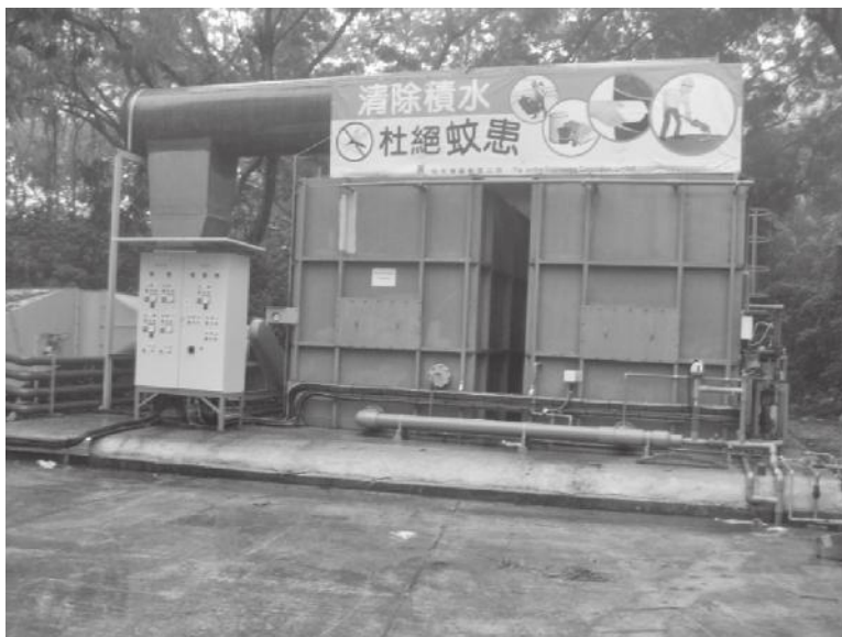
FIGURE 11.10 A vendor-supplied biofilter at a composting facility in Hong Kong.
