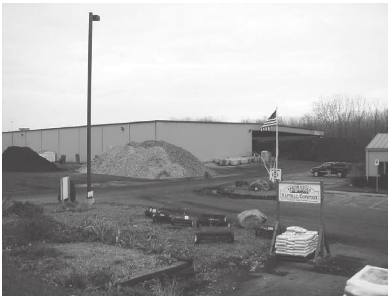
FIGURE 3.1 Davenport, Iowa, biosolids and yard waste composting facility. Yard waste to be used as a bulking agent is chipped on site. In the foreground, bags of the finished product are available for sale.
