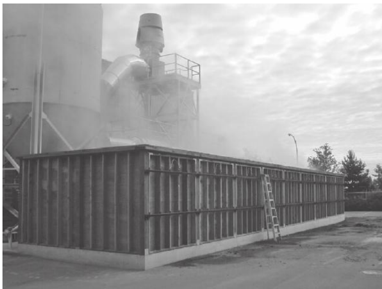
FIGURE 11.9 Biofilter designed by the author at a Victoria, Canada, wastewater treatment plant during smoke testing.
