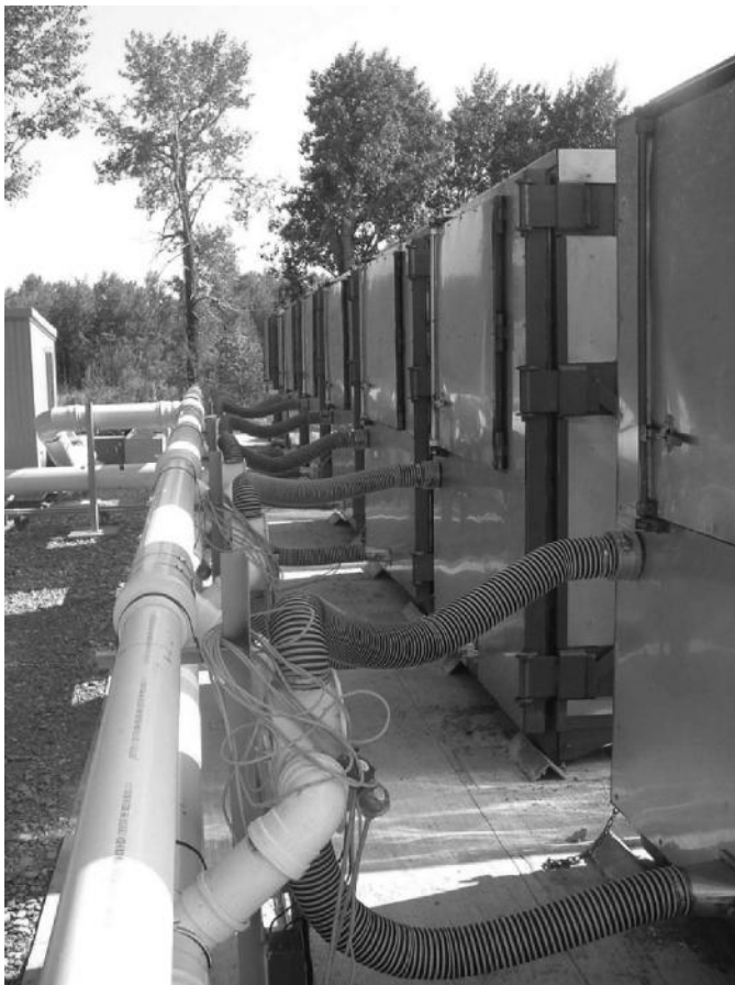
FIGURE 6.16 Aeration system for portable composting bins. (Courtesy of ECS, Seattle, Washington.)
