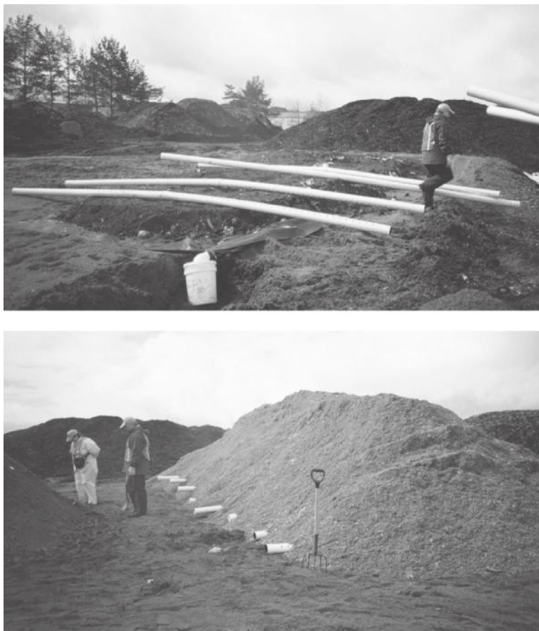
FIGURE 6.2 Passive aeration pile or windrow under construction and in use.
