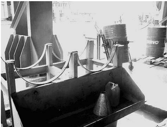
Figure 12.7 Oil handling—poor practices
