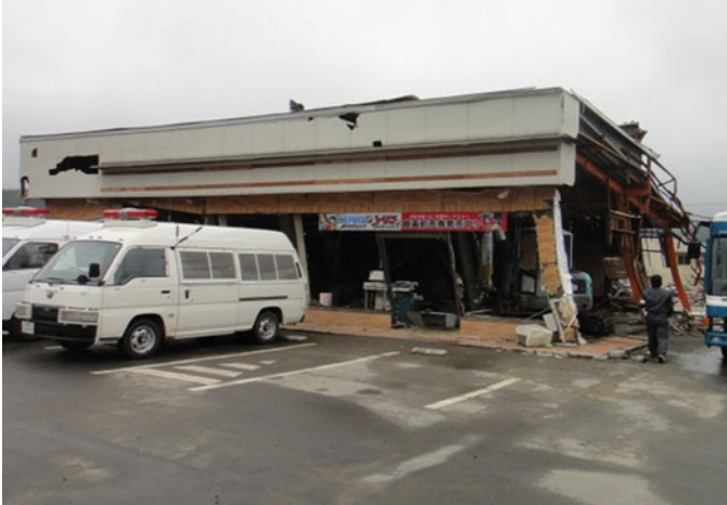
Fig. 8.106 Store E: external view
