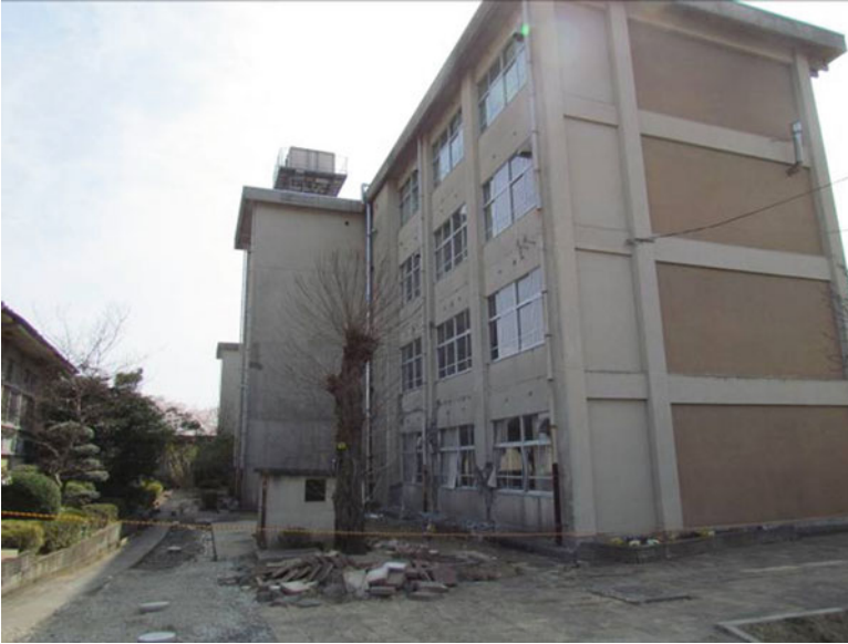
Fig. 4.40 West side view of Building “A”
