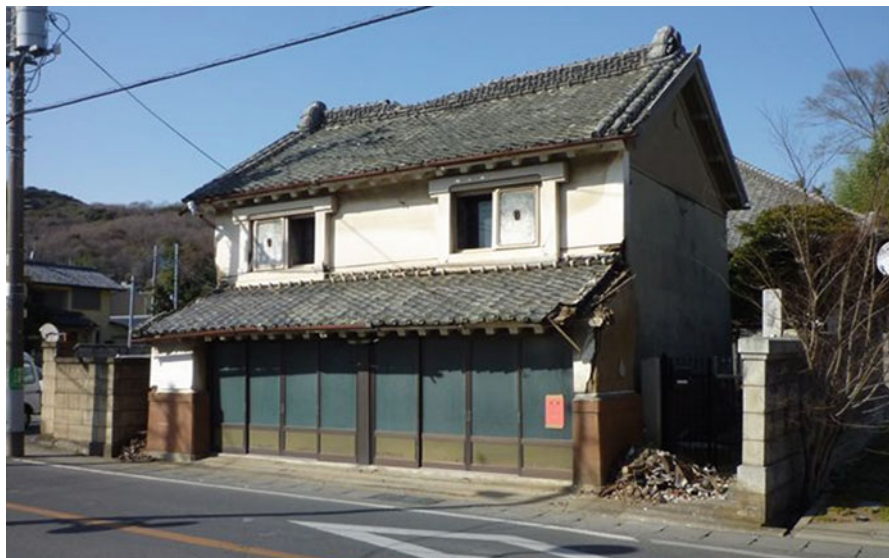
Fig. 3.9 Damage to storehouse with heavy clay walls in Tsukuba
