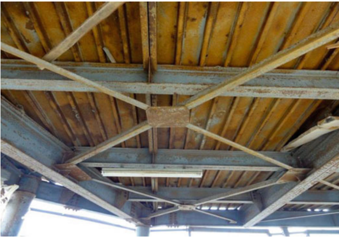
Fig. 8.99 Warehouse D: roof bracing
