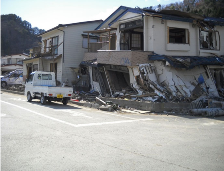
Fig. 2.81 A wooden house destroyed by tsunami with 3.2 m inundation height
