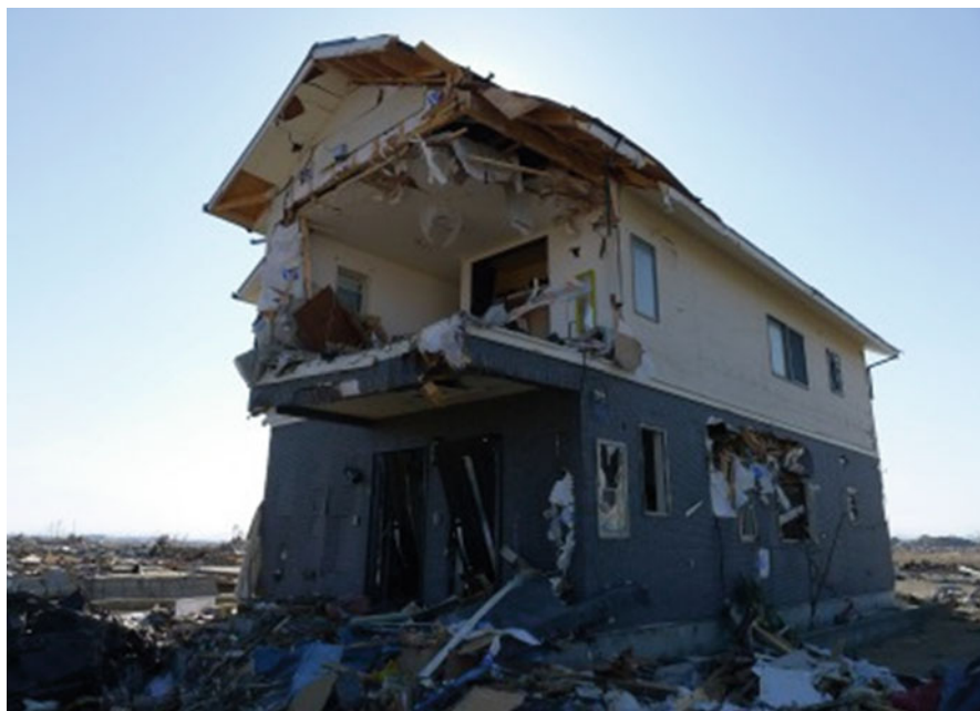
Fig. 3.24 Wood building escaping complete devastation
