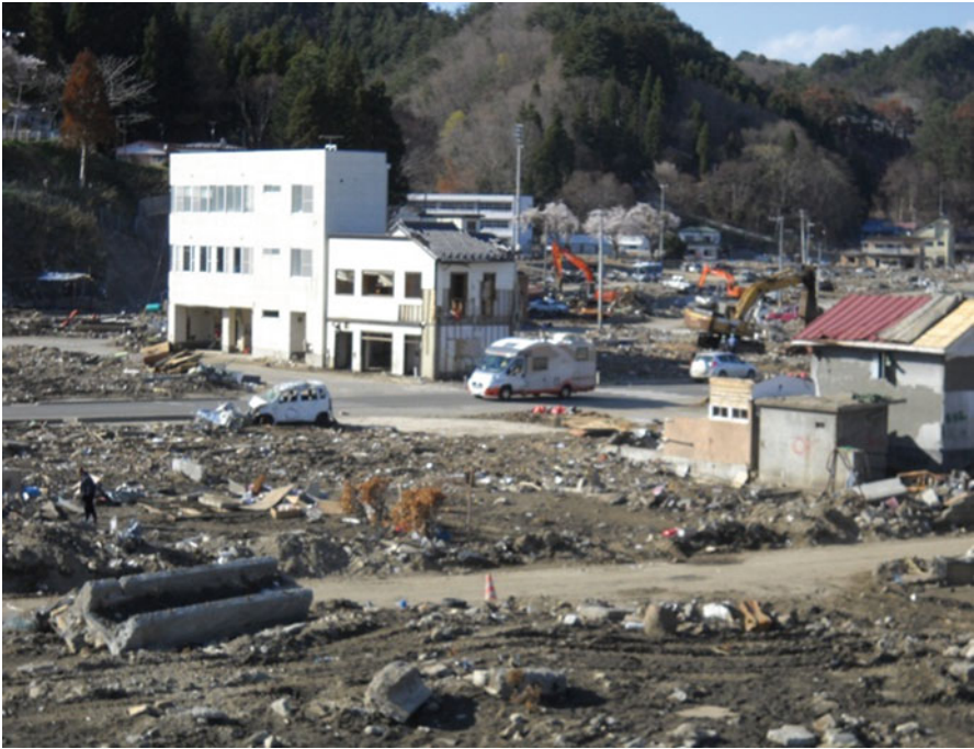
Fig. 2.79 2-storied and 3-storied RC buildings in the western end area of Taro-Cho
