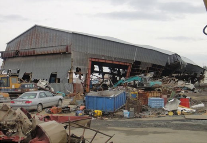
Fig. 8.119 Factory F: external view
