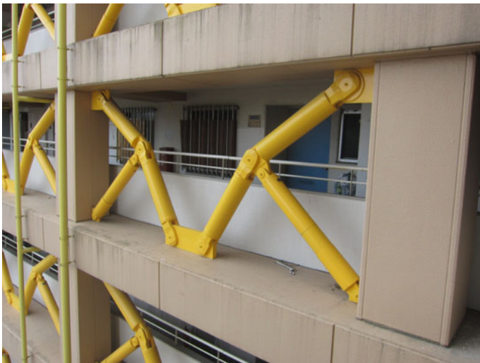
Fig. 4.71 Oil damper brace with toggle amplification mechanism
