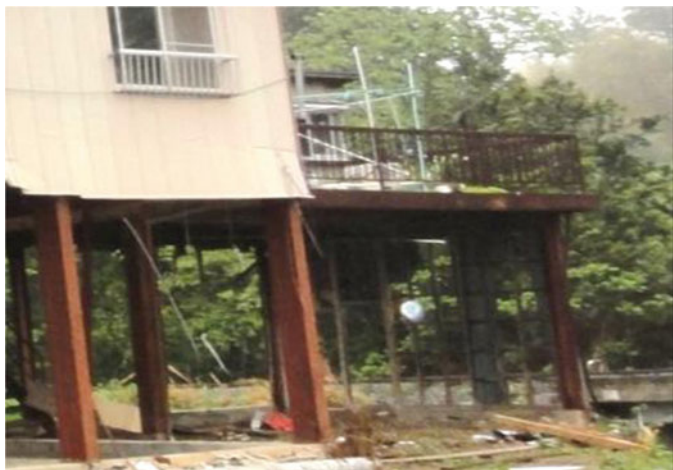
Fig. 8.100 Residence A: external view
