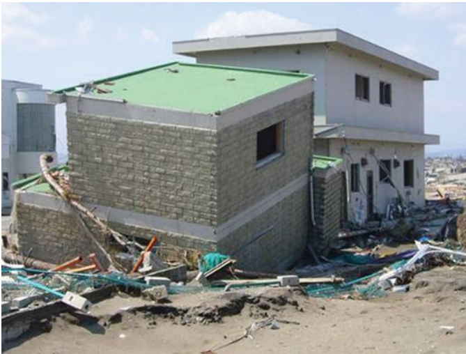
Fig. 7.2 Damaged two-story reinforced hollow concrete masonry houses
