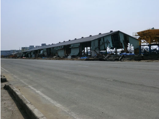
Fig. 8.49 Port facility A: external view
