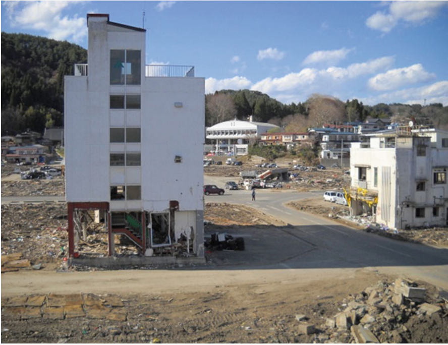
Fig. 2.77 A steel-made 5-storied building in the central area of Taro-Cho that remained after tsunami
