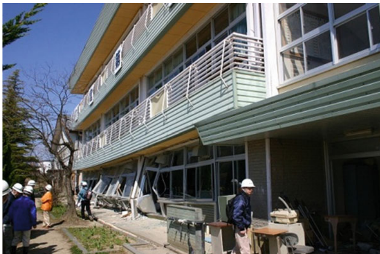
Fig. 4.27 Southern view of south building
