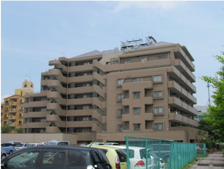
Fig. 5.13 Overall view of the apartment building K1
