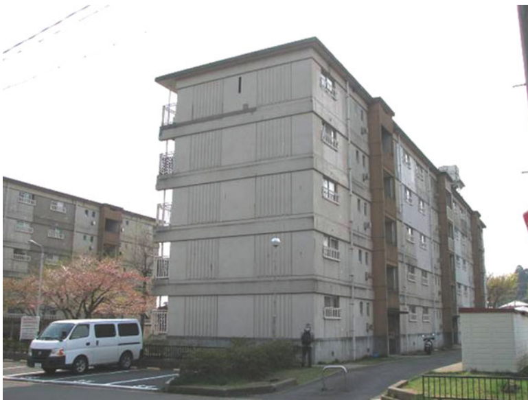
Fig. 6.25 Building D in Natori city
