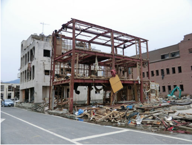
Fig. 8.63 Building E: external view
