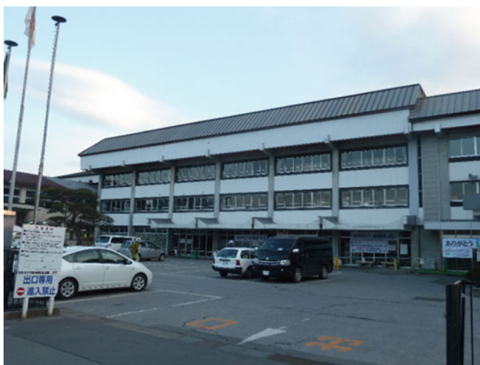
Fig. 4.50 Overall view of the building
