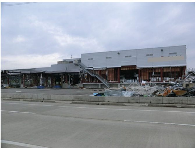
Fig. 8.145 Factory I: external view
