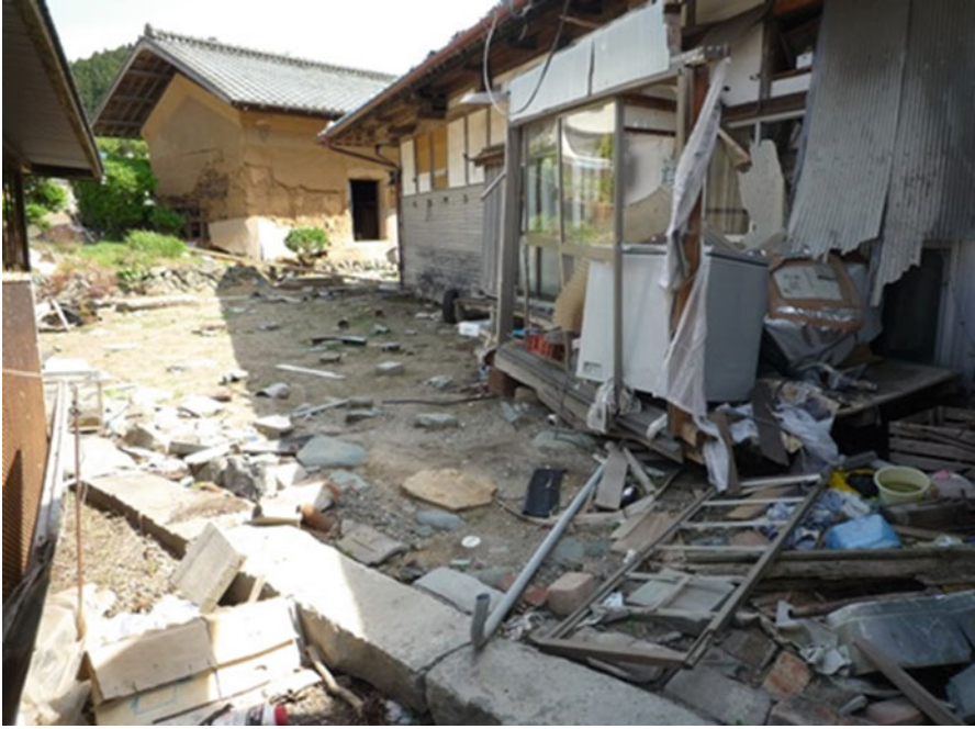
Fig. 3.47 Survived and rotated old house
