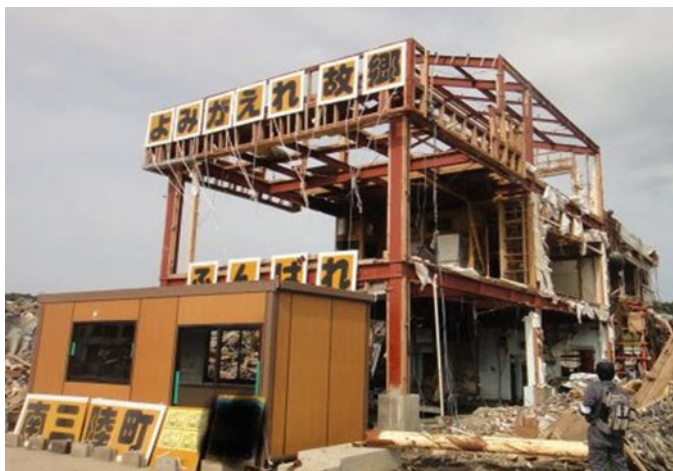
Fig. 8.88 Store B: external view
