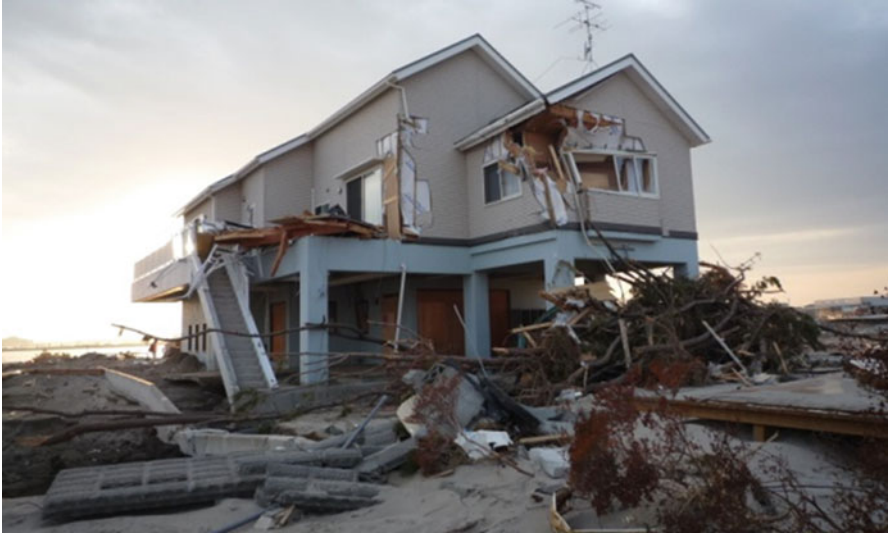
Fig. 3.36 Composite structure consisting of RC on the first floor and wood construction on the second floor
