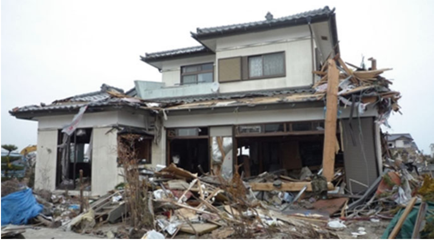
Fig. 3.28 Wood house remaining without the protection of the forest (location (J))
