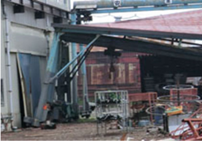
Fig. 8.148 Factory J: leaning columns
