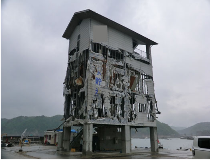
Fig. 8.151 Ice making factory A: exterior view
