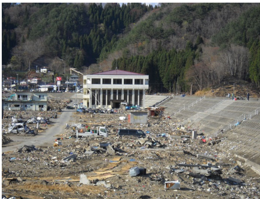
Fig. 2.74 North-side view from the seawall top
