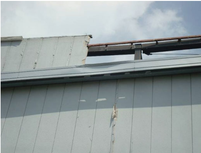
Fig. 9.44 Damaged parapet
