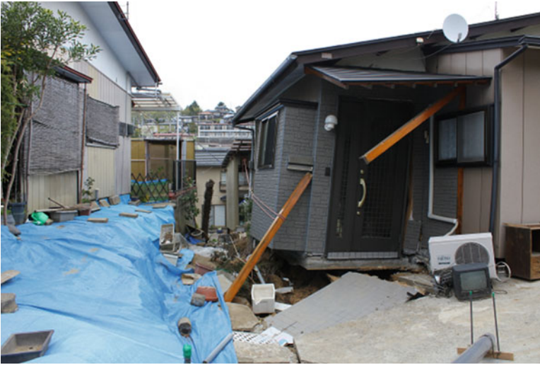
Fig. 10.27 Damage to a house
