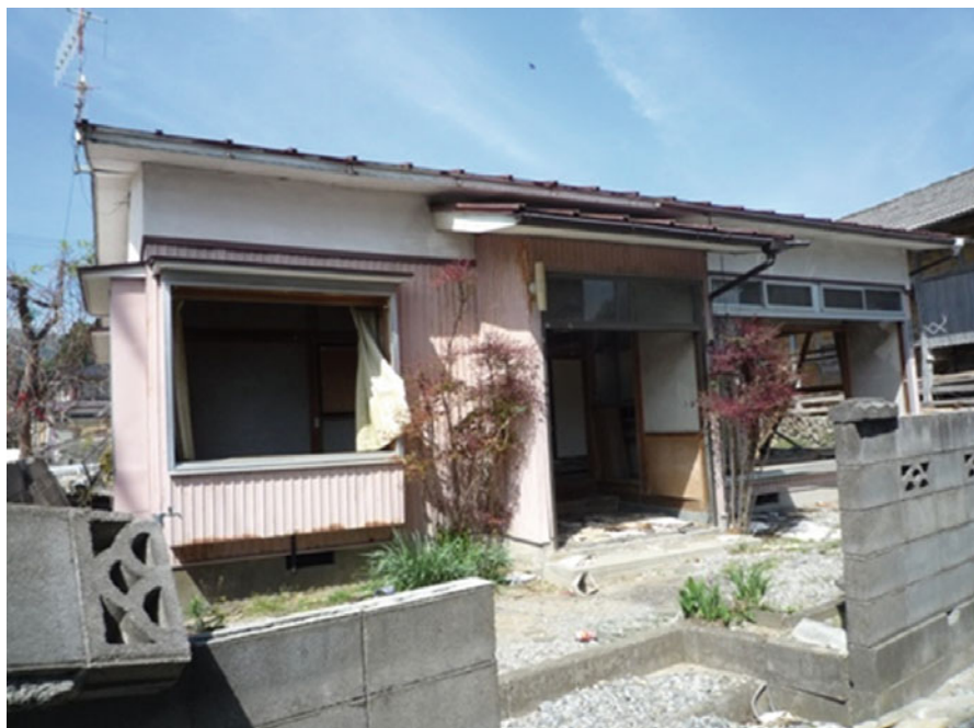
Fig. 3.45 Survived house in spite of minor structural specifications
