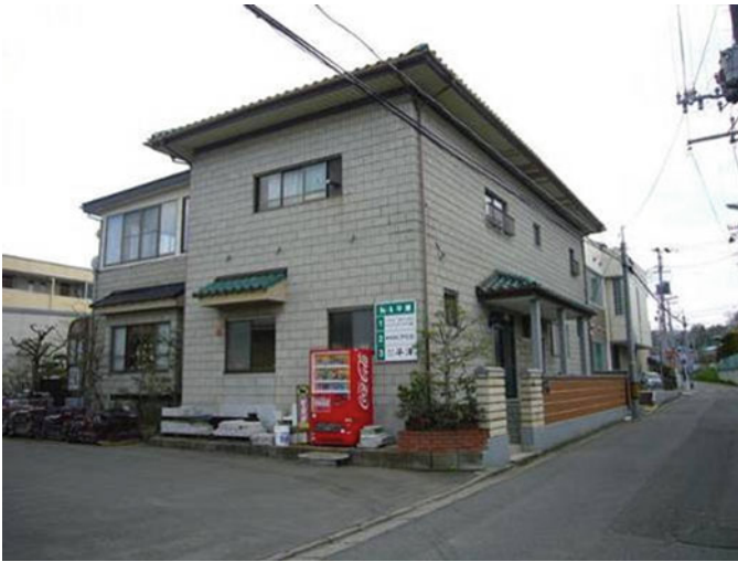
Fig. 7.6 A reinforced fully grouted concrete masonry house without any damage
