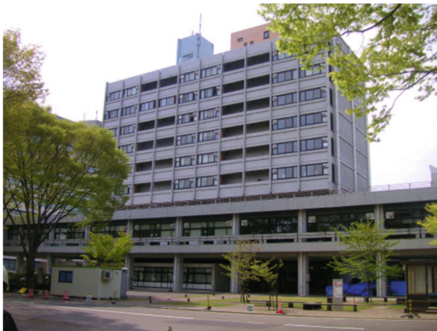
Fig. 5.26 Overall view of University T-2 building
