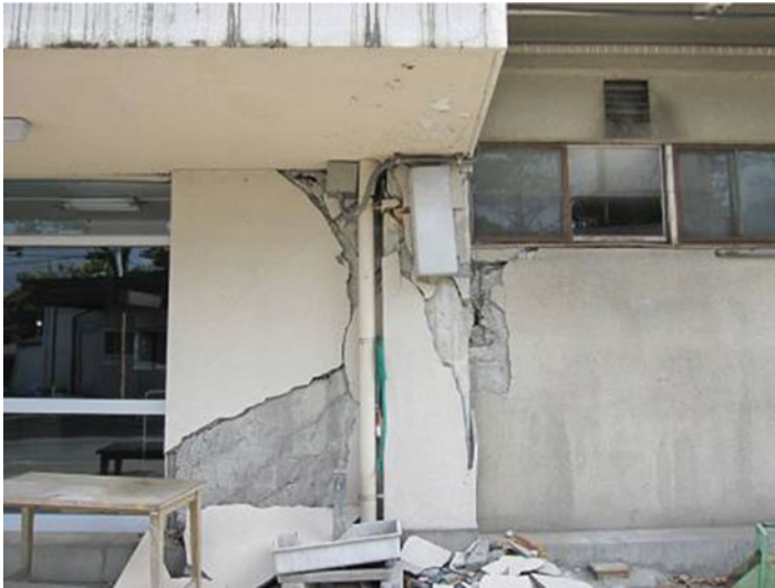
Fig. 4.61 Column with wing wall
