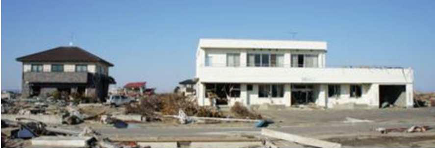
Fig. 3.22 Wood house remained downstream of RC building
