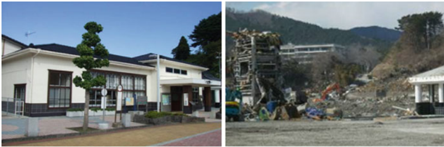
Fig. 1.10 Onagawa station before and after tsunami
