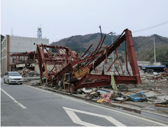
Fig. 8.61 Building D: external view
