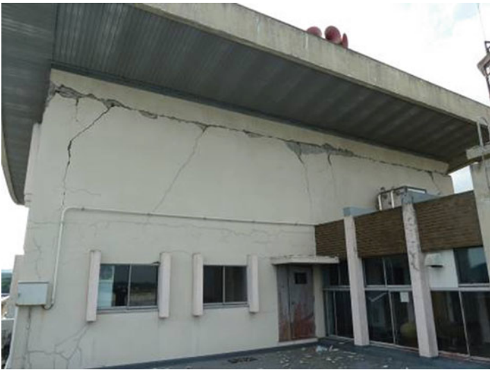
Fig. 4.63 Wall in the third story
