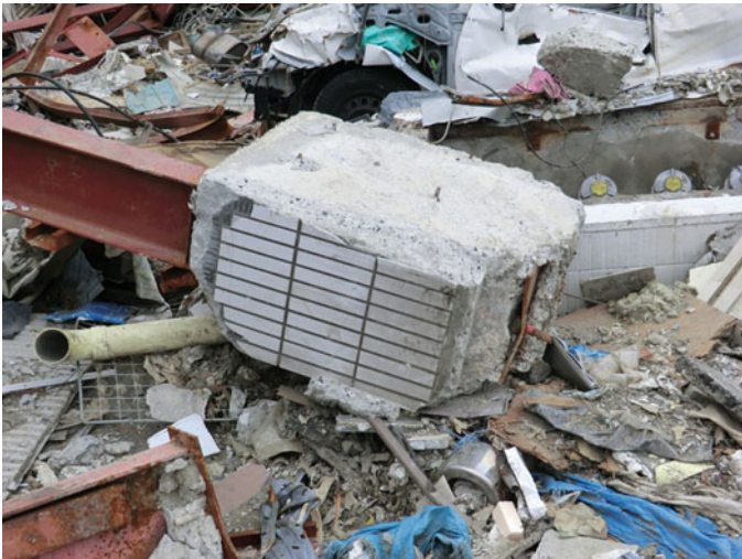
Fig. 8.68 Building F: column base
