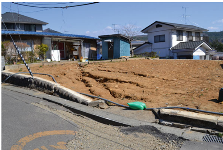
Fig. 10.23 Large cracks
