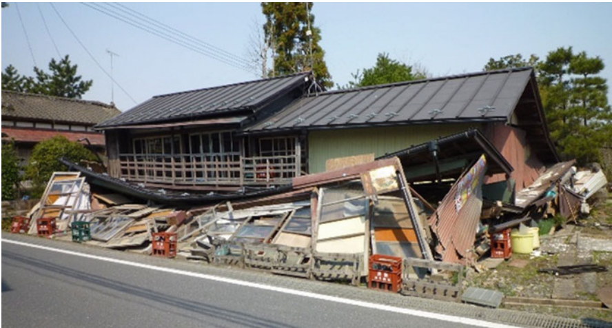
Fig. 3.3 Collapse of wood house with store attached in Misato
