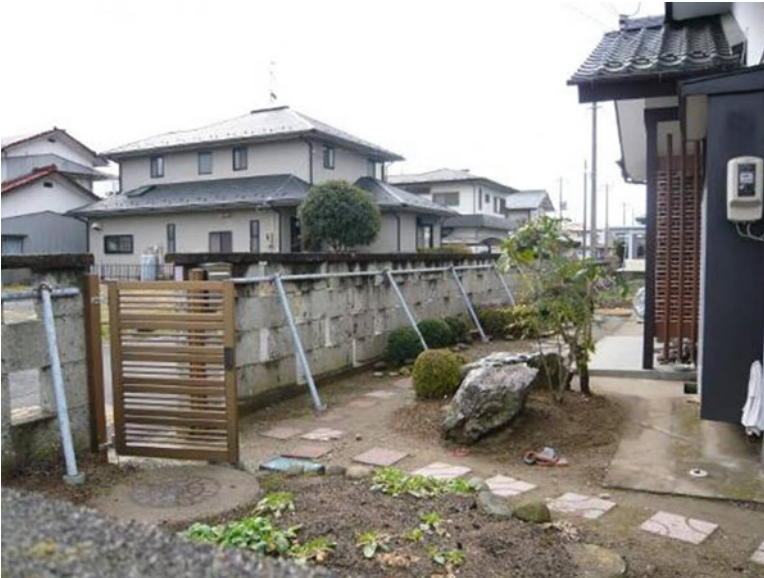
Fig. 7.22 Stone masonry garden wall retrofitted with steel structure
