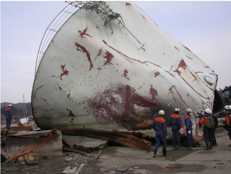
Fig. 1.7 Oil tank collapsed by tsunami
