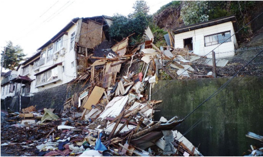
Fig. 3.17 Collapse of hotel due to landslide in Sendai-city
