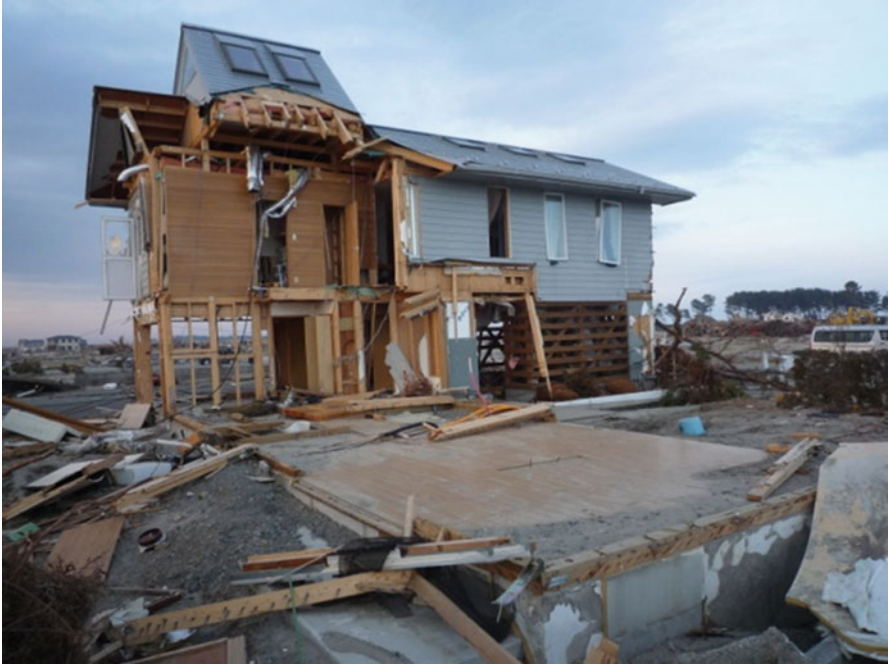
Fig. 3.34 A portion of a wood house washed away
