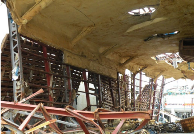
Fig. 8.71 Warehouse A: inside view
