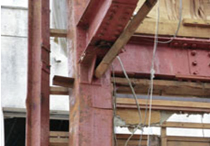
Fig. 8.65 Building E: beam-to-column connections at corner column
