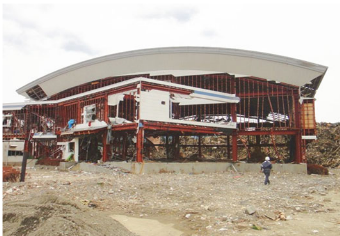
Fig. 8.132 Gymnasium C: external view
