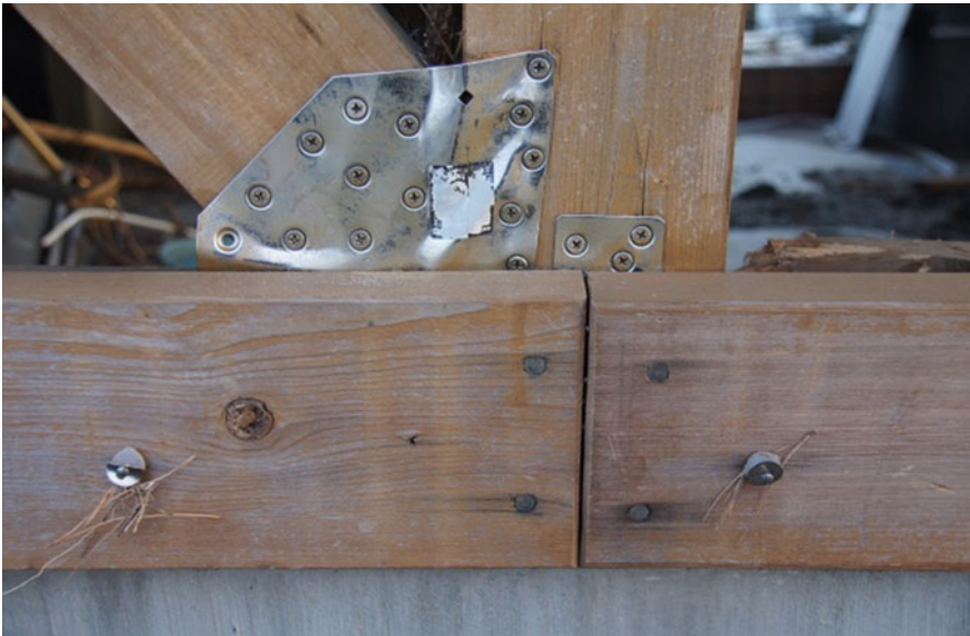
Fig. 3.35 Fastener of joint in the house of Fig. 3.34
