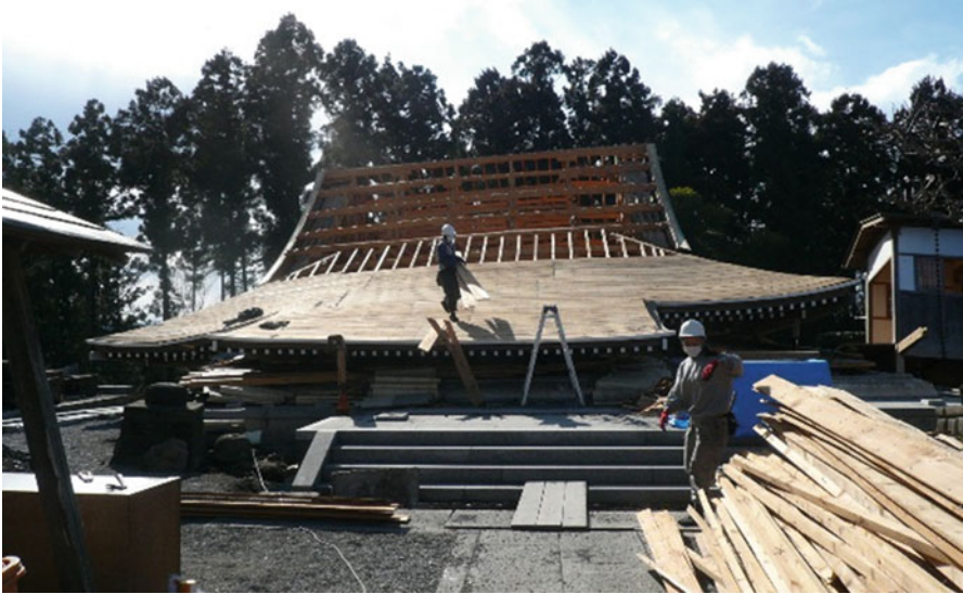
Fig. 3.14 Collapse of the main building of temple in Takanezawa
