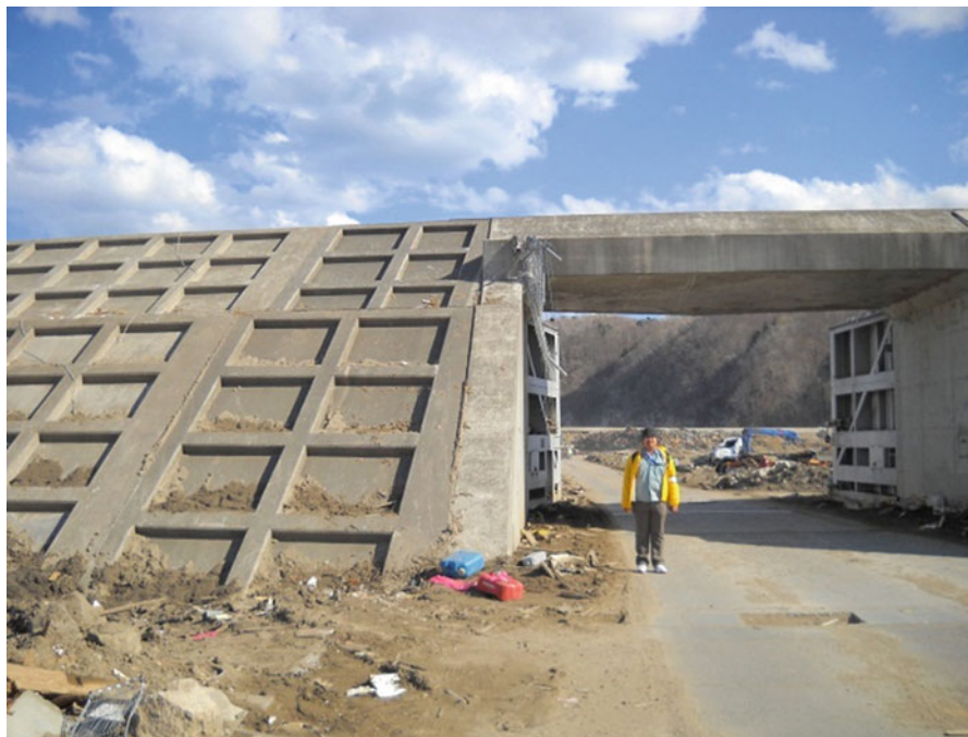
Fig. 2.75 A huge seawall in Taro-Cho, 10 m high from the sea level
