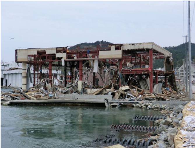
Fig. 8.59 Building C: external view
