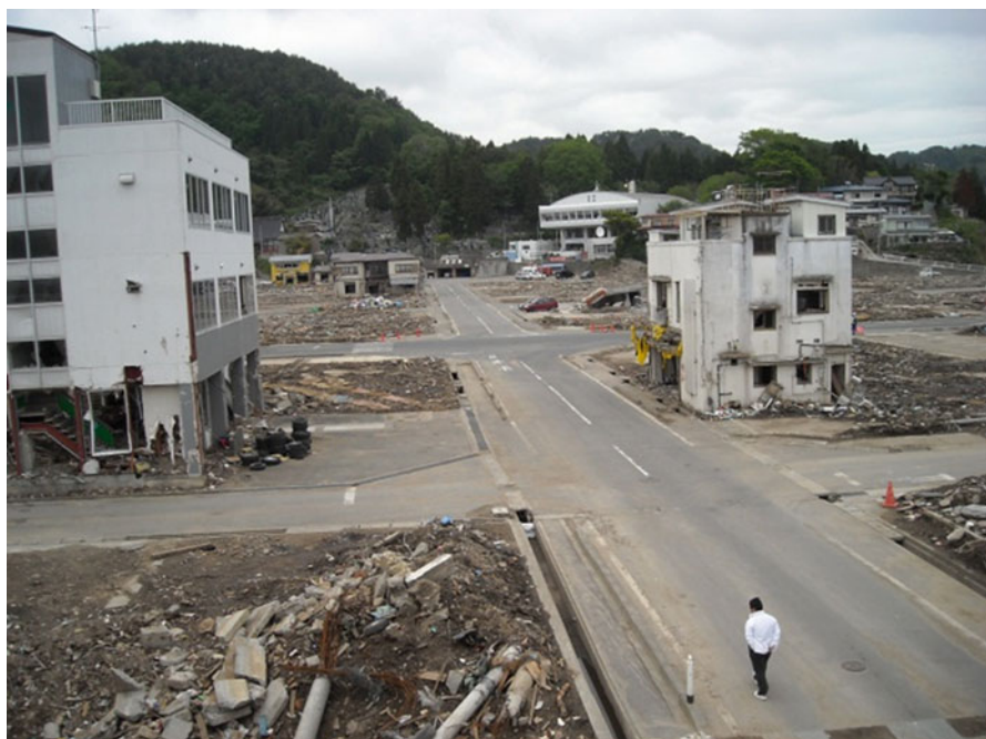
Fig. 2.76 Reinforced concrete buildings and steel-made buildings that remained after tsunami
