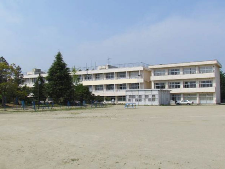
Fig. 4.35 South side view of the building
