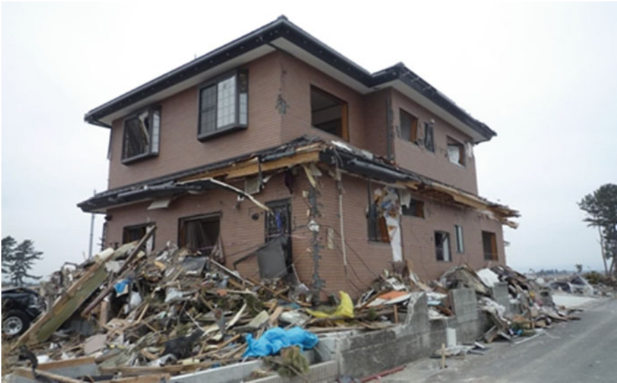
Fig. 3.29 Japanese conventional post and beam house remaining (location (K))
