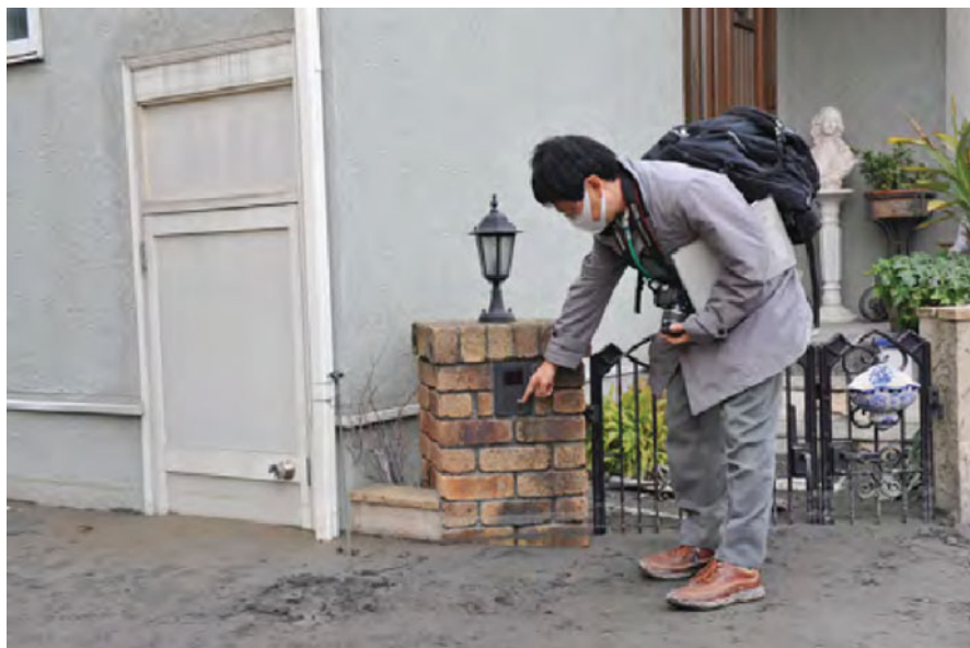
Fig. 10.8 Large building settlement
