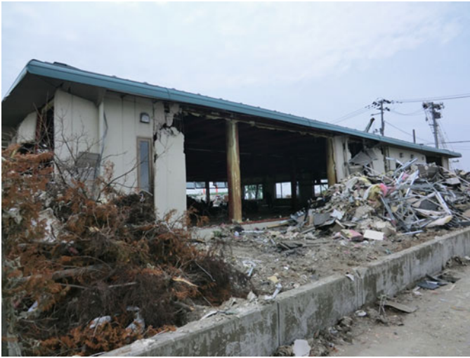
Fig. 8.45 Office building A: external view
