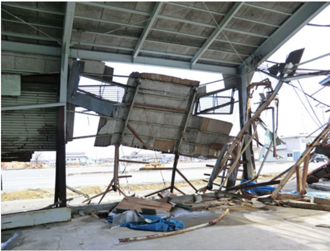
Fig. 8.50 Port facility A: inside view
