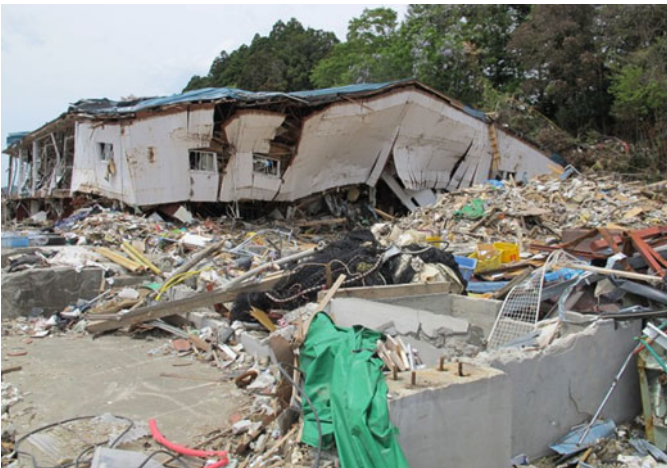
Fig. 8.131 High-school gymnasium B: building displaced by 20 m
