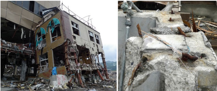
Fig. 8.137 Office building: anchor bolts fractured; building leaning on next building
