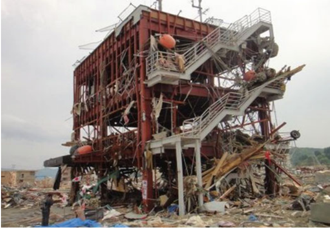
Fig. 8.84 Office building F: external view
