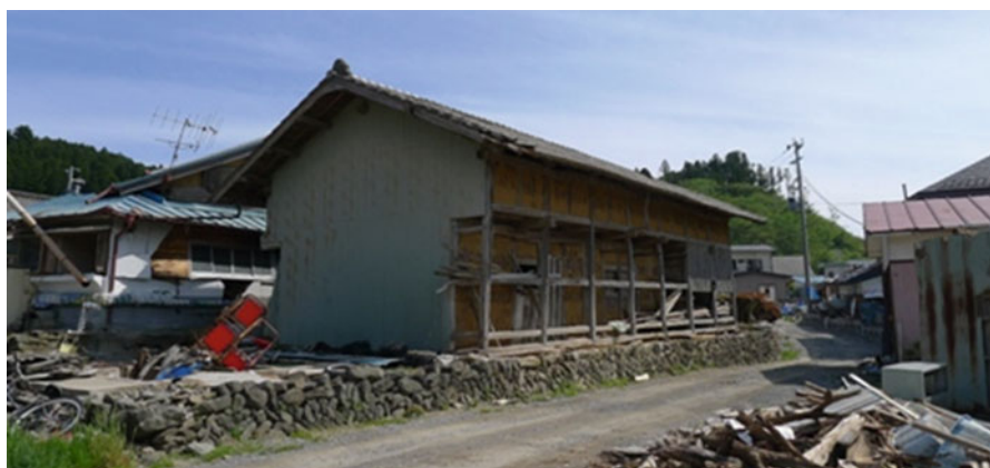
Fig. 3.46 Survived warehouse in spite of minor structural specifications
