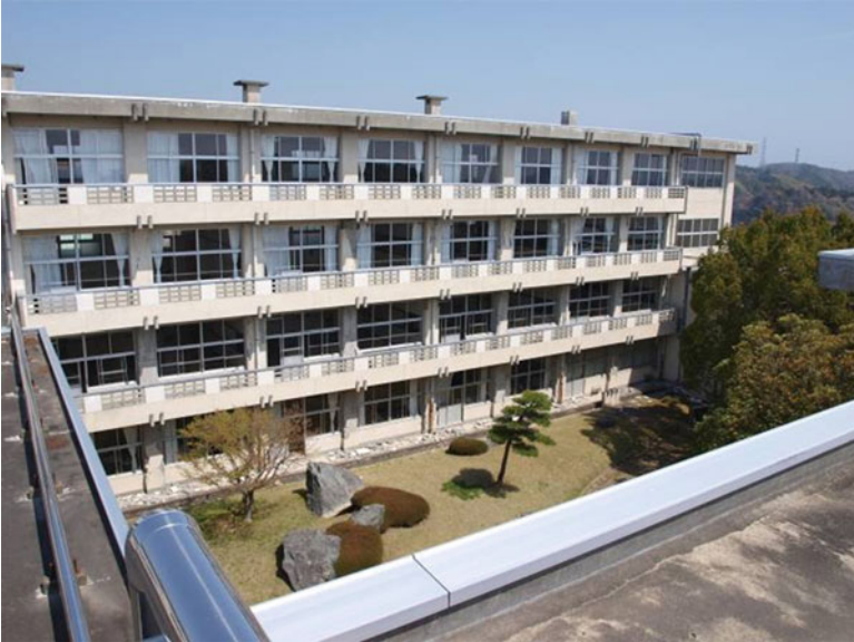
Fig. 4.38 Overview of Building “A”
