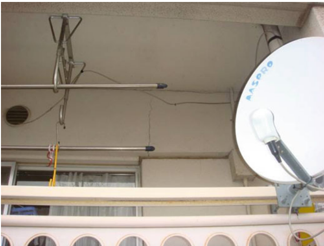
Fig. 6.29 Crack in second floor beam of Building D
