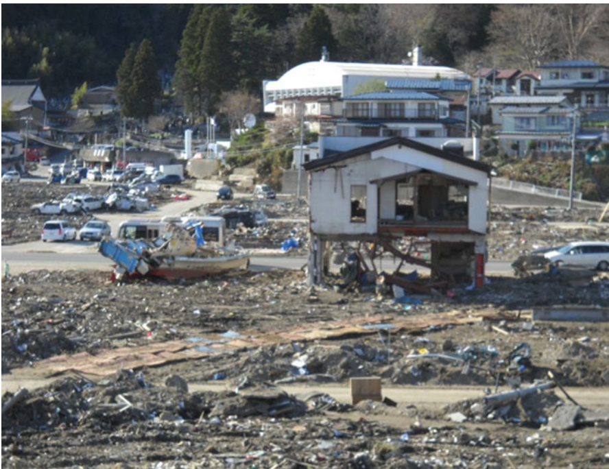
Fig. 2.78 A steel-made 2-storied building in the central area of Taro-Cho that remained after tsunami
