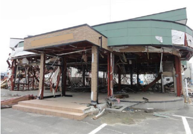
Fig. 8.102 Store D: external view
