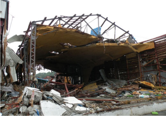
Fig. 8.69 Warehouse A: external view
