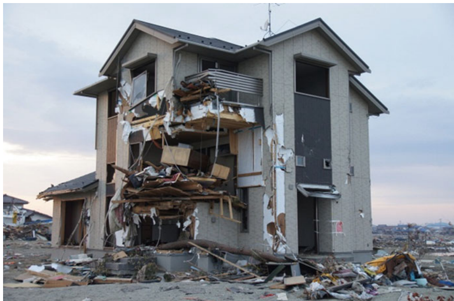
Fig. 3.38 Three-story wood house remaining
