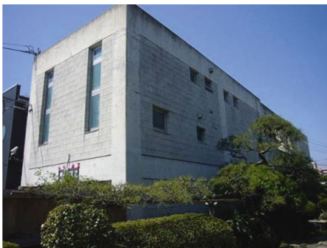
Fig. 7.8 Undamaged RC building with concrete masonry nonbearing walls
