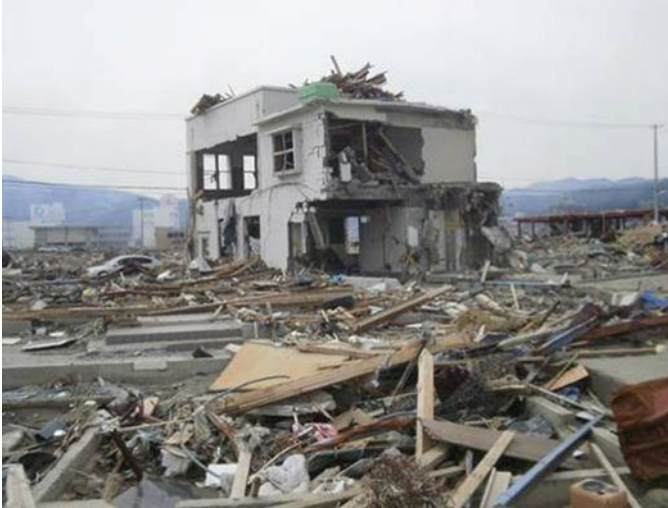
Fig. 7.9 Damaged RC building with nonbearing concrete masonry walls
