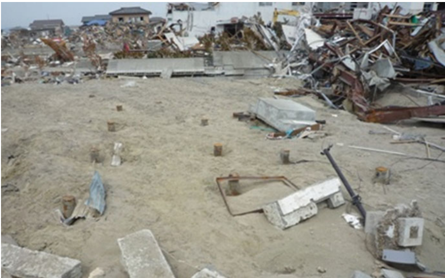
Fig. 3.27 Steel pile left of the original position in Fig. 3.26
