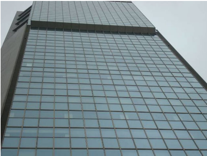
Fig. 9.31 Glass curtain wall without damage
