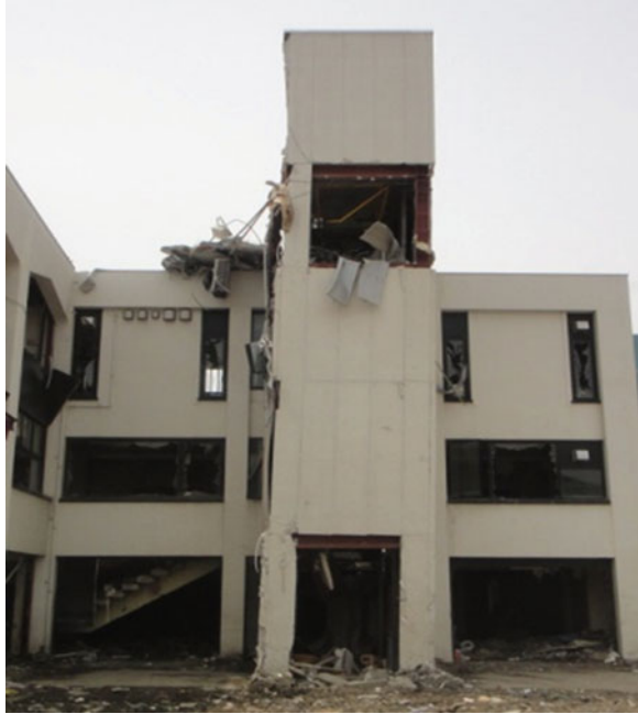
Fig. 8.121 Office building G: external view
