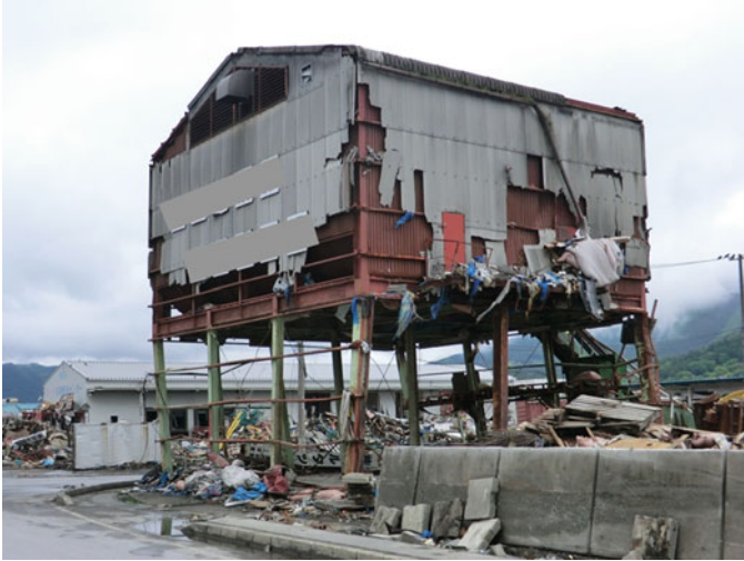
Fig. 8.155 Factory K: external view
