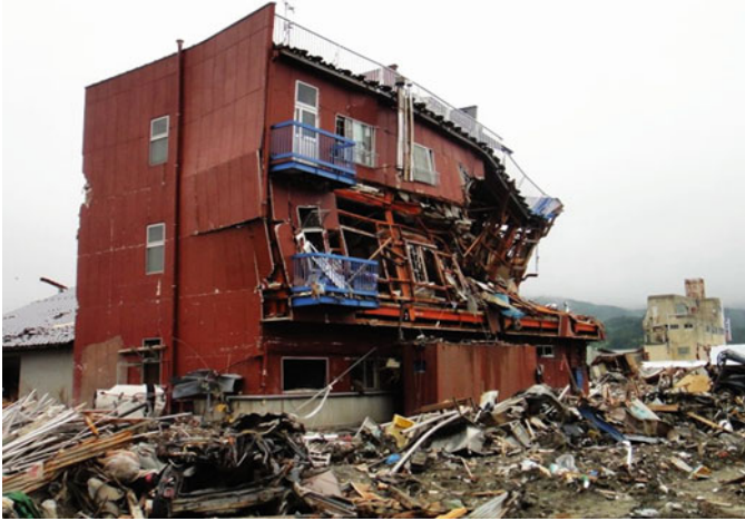
Fig. 8.104 Traditional hotel A: external view
