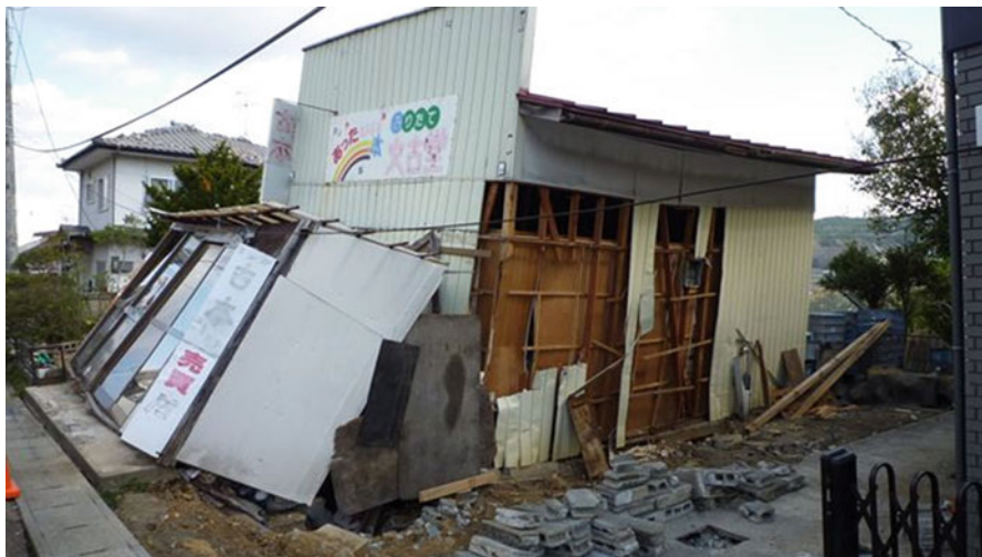
Fig. 3.19 Severe damage to a house due to landslide in Sendai-city
