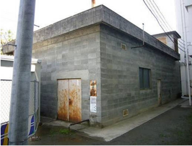
Fig. 7.1 A reinforced hollow concrete masonry building without any damage
