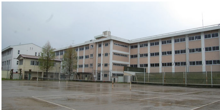
Fig. 4.43 Northern side view of the building No. 3
