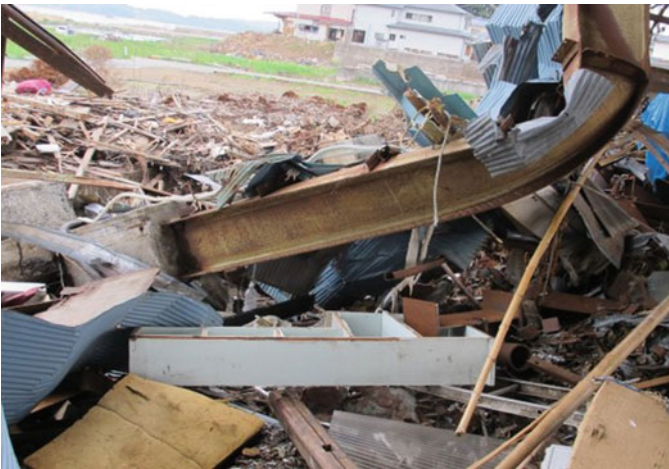
Fig. 8.120 Factory F: collapsed column
