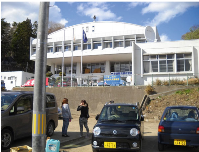
Fig. 2.72 Taro-Cho town office (3-storied RC building on high ground, not affected)
