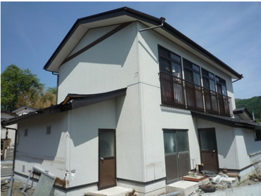
Fig. 3.42 Wood house without damage with over 7 m wave depth
