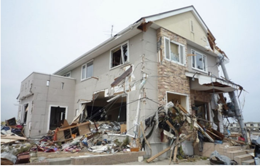
Fig. 3.30 One of few light frame construction houses remaining (location (L))
