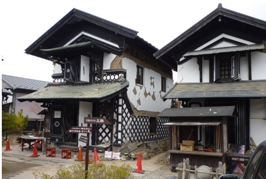
Fig. 3.7 Damage to older storehouses in Osaki
