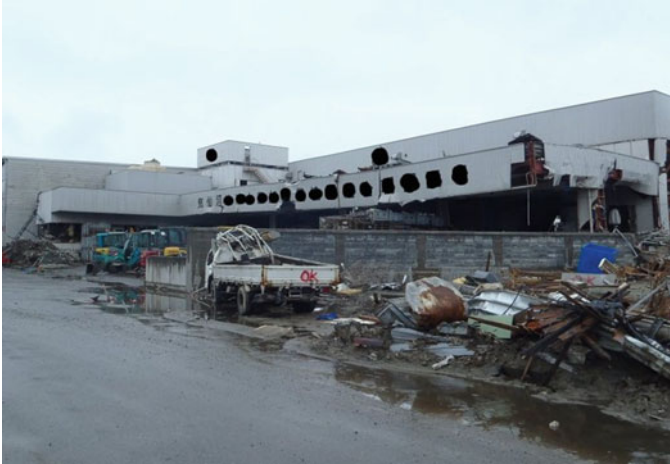
Fig. 8.110 Factory B: external view
