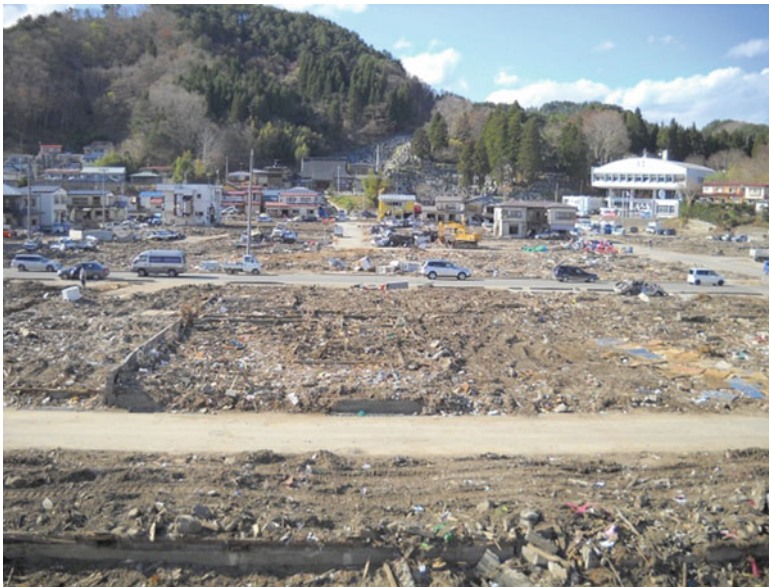
Fig. 2.71 Overview of Taro-Cho central area from the seawall top
