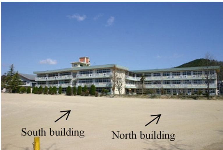
Fig. 4.26 South-east panoramic view of south building and north building
