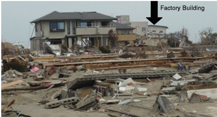
Fig. 3.32 Wood houses moved away from downstream of the factory building (location (P))
