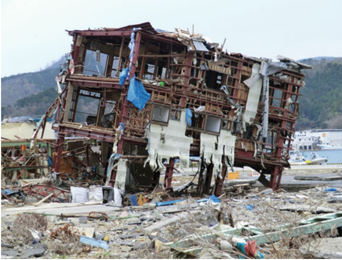
Fig. 8.55 Building A: external view showing large tilt
