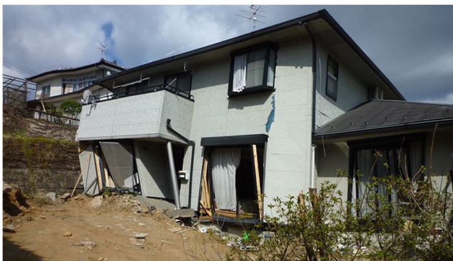
Fig. 3.20 Severe damage to a house due to landslide in Sendai-city
