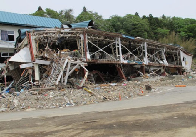
Fig. 8.130 High-school gymnasium B: external view of collapsed building
