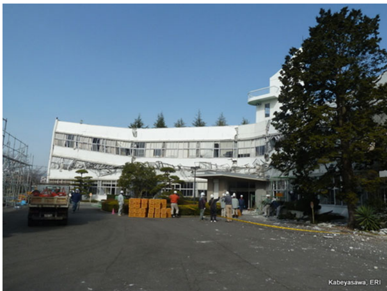
Fig. 4.20 South overview of west wing
