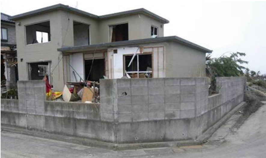
Fig. 7.20 Undamaged concrete masonry garden wall by tsunami wave
