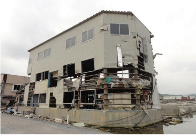
Fig. 8.98 Warehouse D: external view
