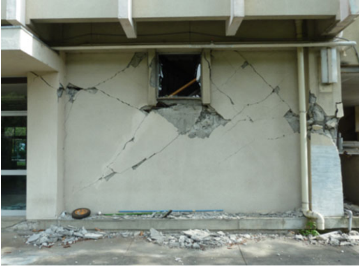
Fig. 4.62 Wall in the first story
