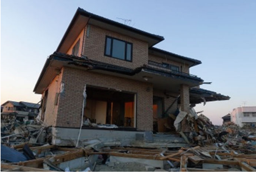
Fig. 3.26 Wood house moved away with foundation
