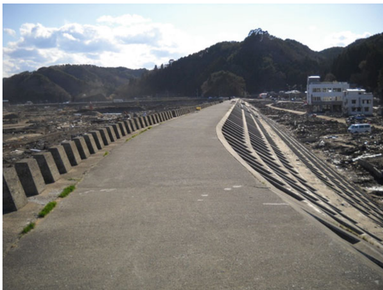
Fig. 2.73 South-side view from the seawall top
