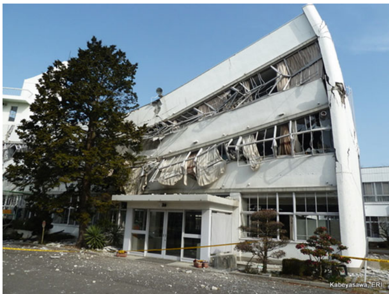
Fig. 4.21 South overview of east wing
