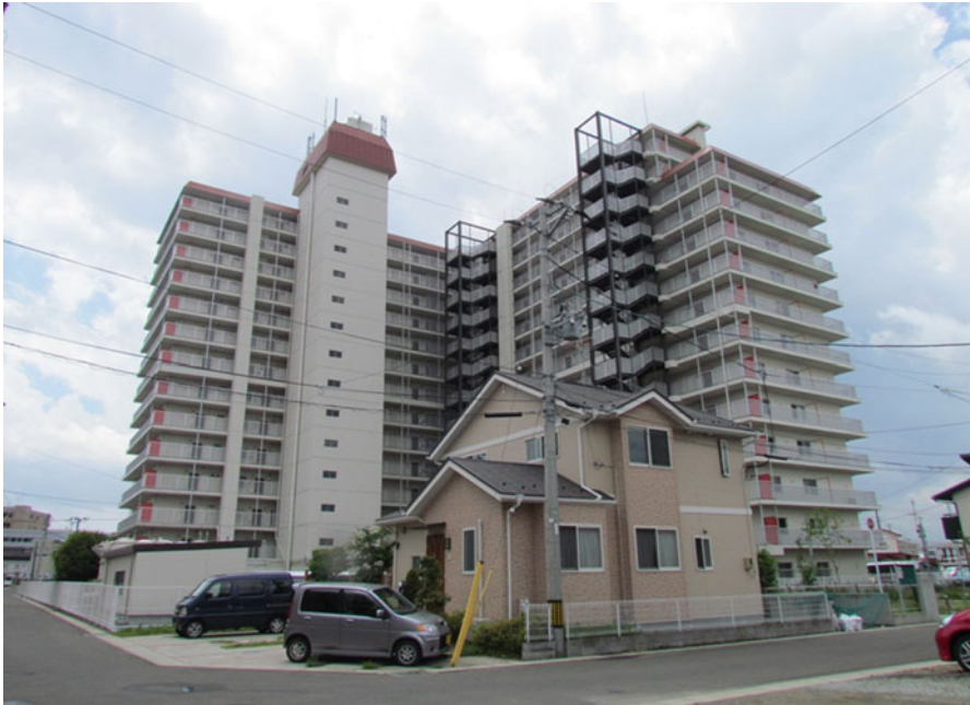
Fig. 5.3 Southside view of the apartment building S1
