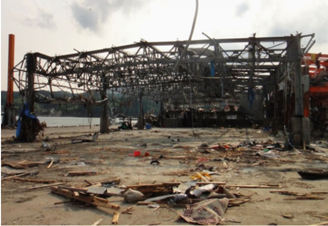
Fig. 8.91 Factory A: external view
