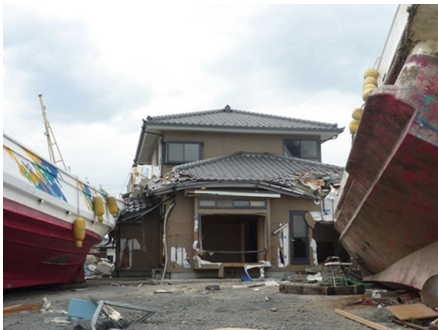
Fig. 3.39 Wood house remaining even after collision with ship
