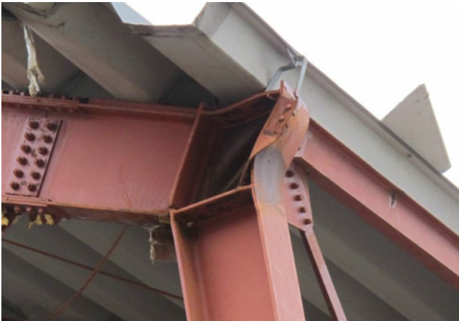
Fig. 8.129 Factory G: large deformation of column panel zone
