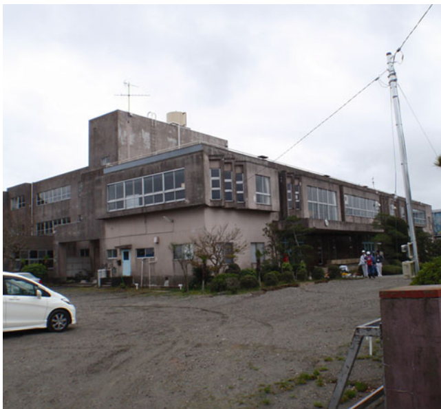
Fig. 4.45 Overall view of school buildings
