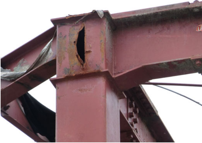
Fig. 8.67 Building F: beam-to-column connection
