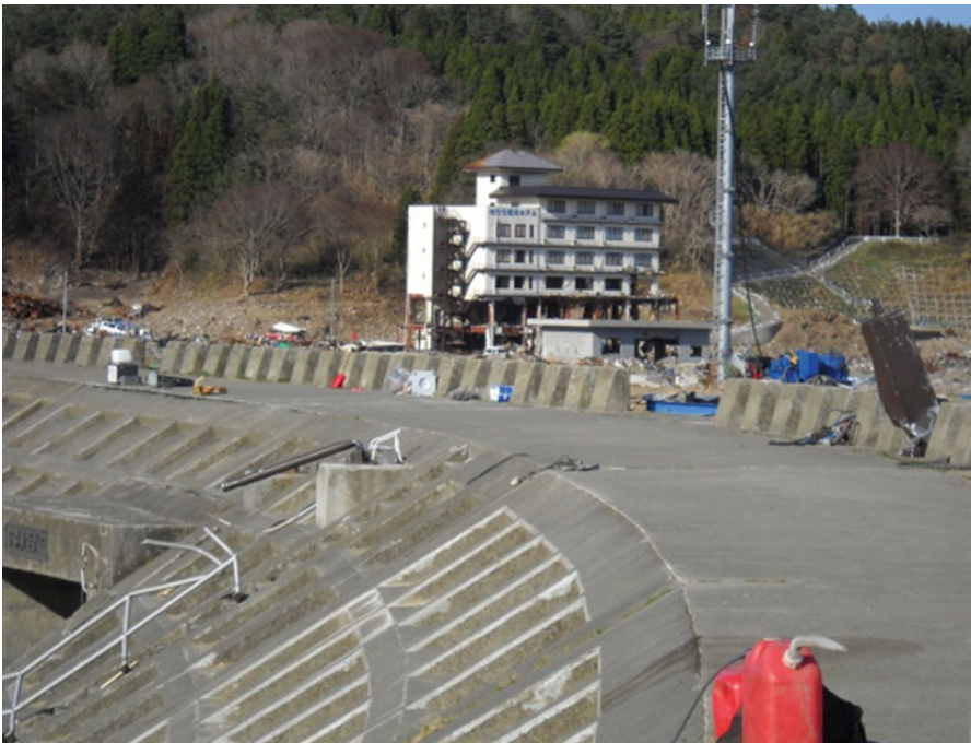
Fig. 2.80 A steel-made 5-storied hotel in the southern end area of Taro-Cho
