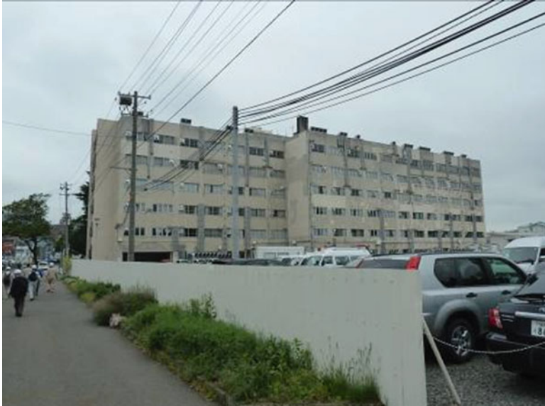
Fig. 4.52 Overview of the building
