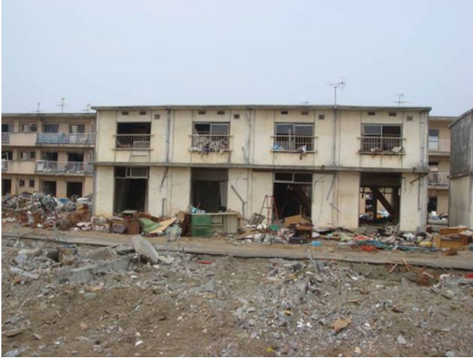
Fig. 6.37 Mass production type public apartment building in Natori city damaged by tsunami
