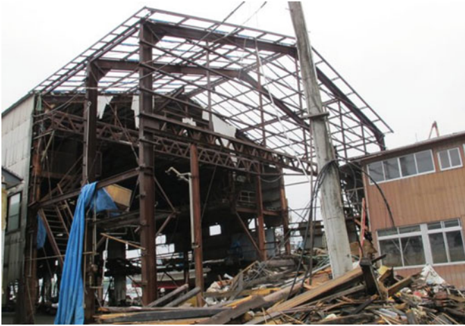
Fig. 8.115 Factory D: external view
