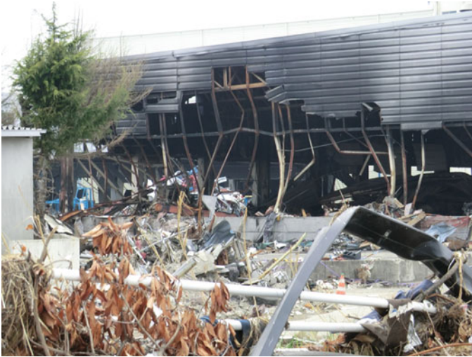
Fig. 8.162 Same building shown in Fig. 8.161 (Miyagino, Sendai)
