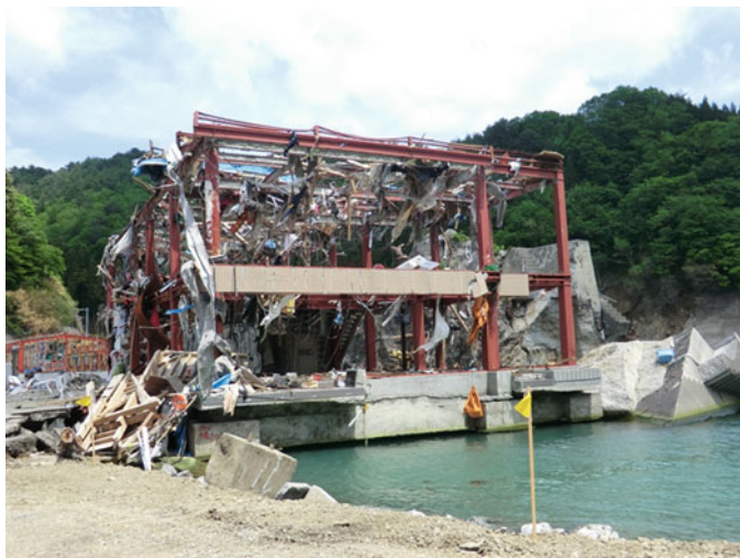
Fig. 8.153 Office building H: external view
