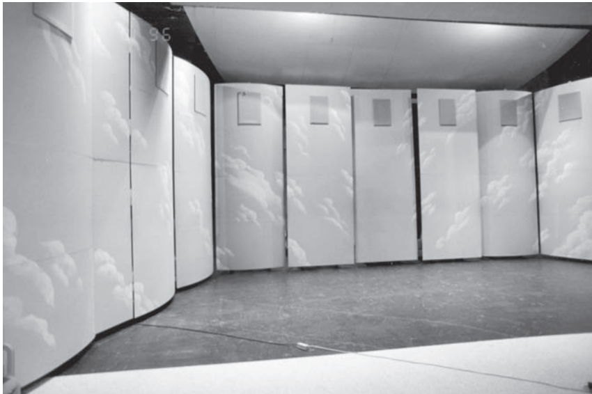
Figure 6.10 Using an electronic reverberation enhancement system one can achieve high flexibility in room acoustic conditions. The photo shows an active system for control of acoustics on a stage using loudspeakers integrated into a stage shell to achieve a proper blend of early reflections and local reverberation. Installation in Motala Community Center, Sweden. (Photo by Mendel Kleiner.)
