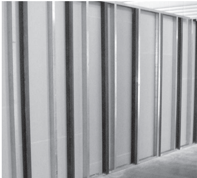
Figure 10.7 A double-panel drywall under construction showing the back of one panel and the steel studs, waiting for glass wool filling and the second panel to be installed.
