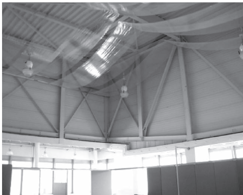
Figure 7.15 Microperforated foils can be successfully employed as translucent sound absorbers. (Microsorber photo courtesy of KAEFER, Germany)
