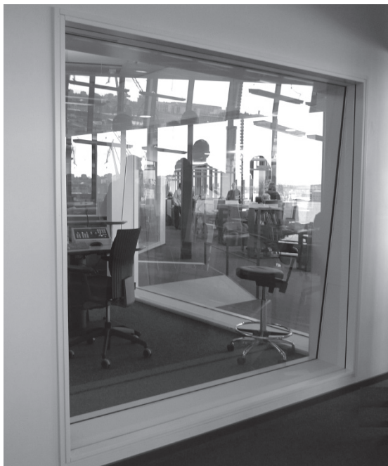
Figure 10.11 Example of a window between a recording studio and a control room that uses offset (non-parallel) glass panes and sound-absorptive material at the interior air space edges. (Photo by Mendel Kleiner.)
