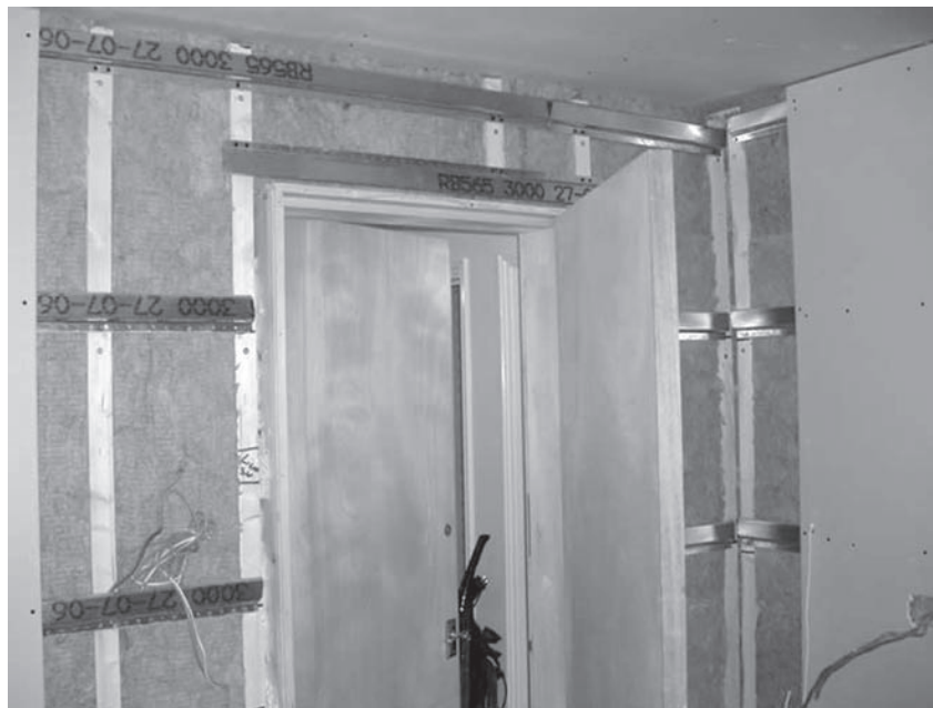
Figure 10.10 A resilient layer being added to a room to improve the sound isolation (photo by Alex Hill, Soundservice, UK).
