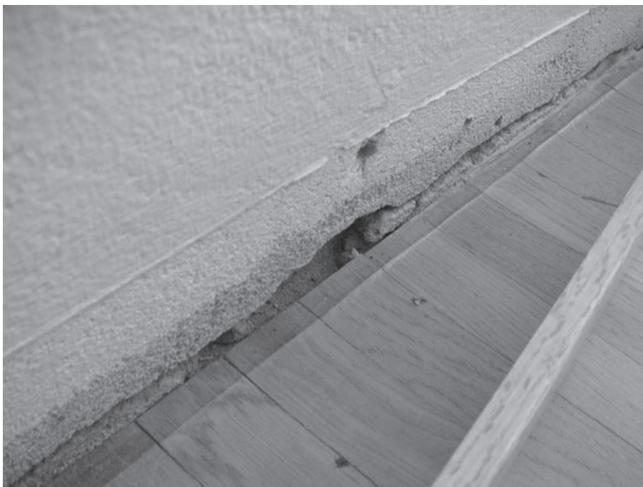
Figure 10.13 A major leak, between a lightweight concrete wall and the floor, that was hidden by wood trim. (Photo by Mendel Kleiner.)
