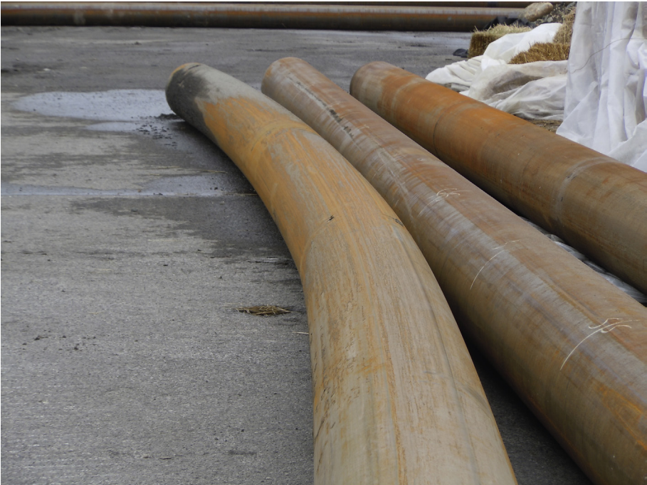
Plate 25.1 Bent piles identified and removed.
