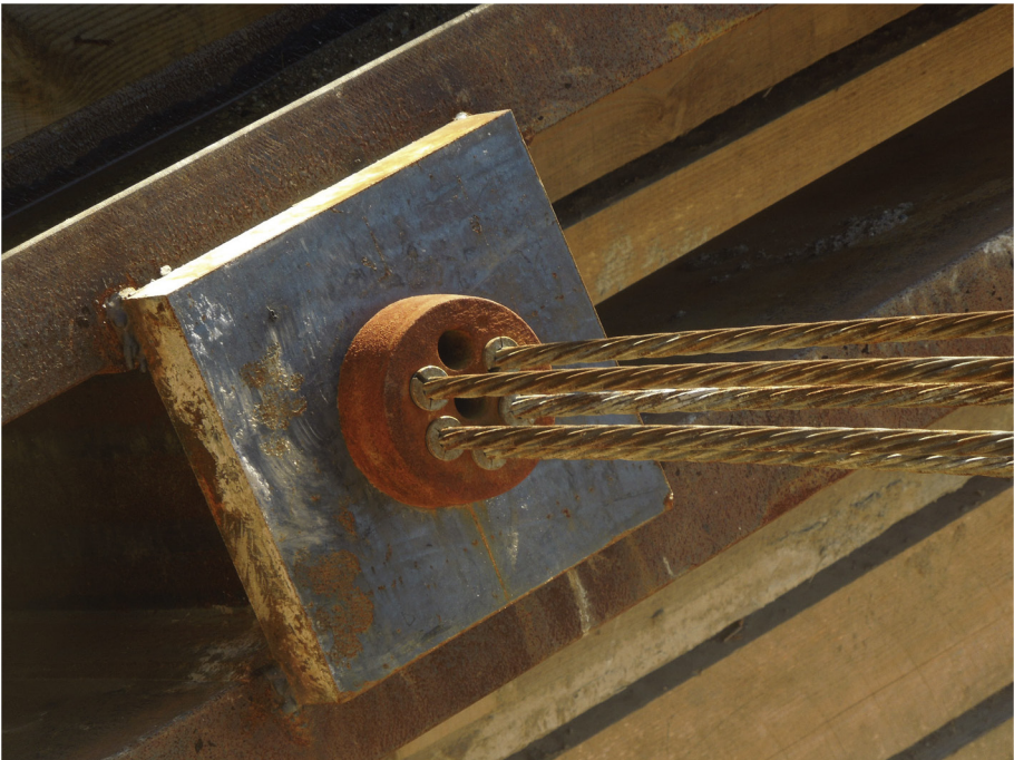
Plate 8.4 Soil anchor.
