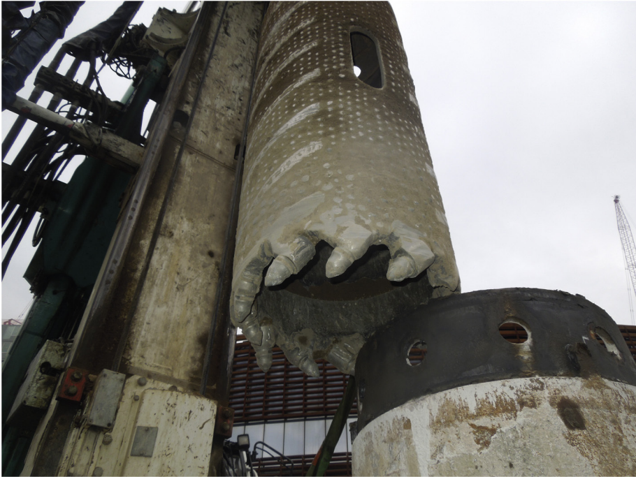
Plate 6.1 Special rock cutting cutter head (these can cut through boulders).
