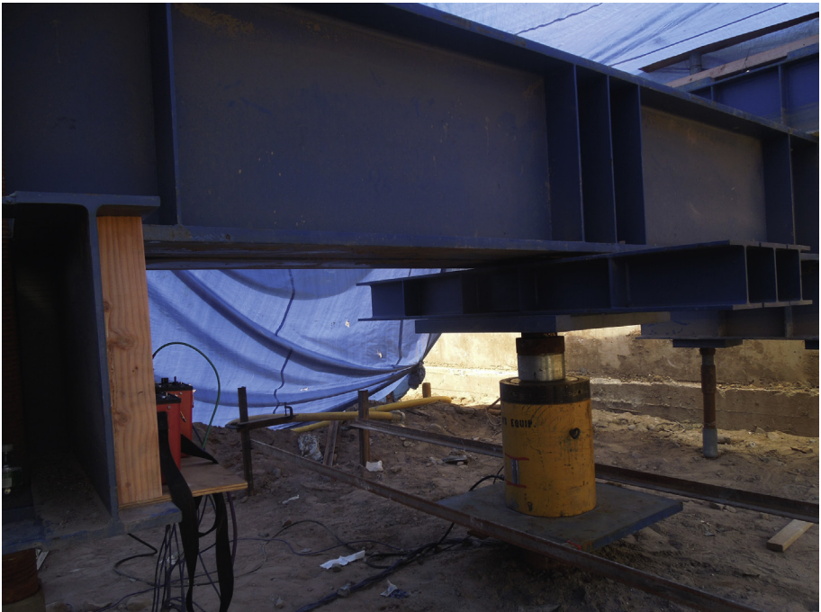
Plate 24.1 Pile load test.
