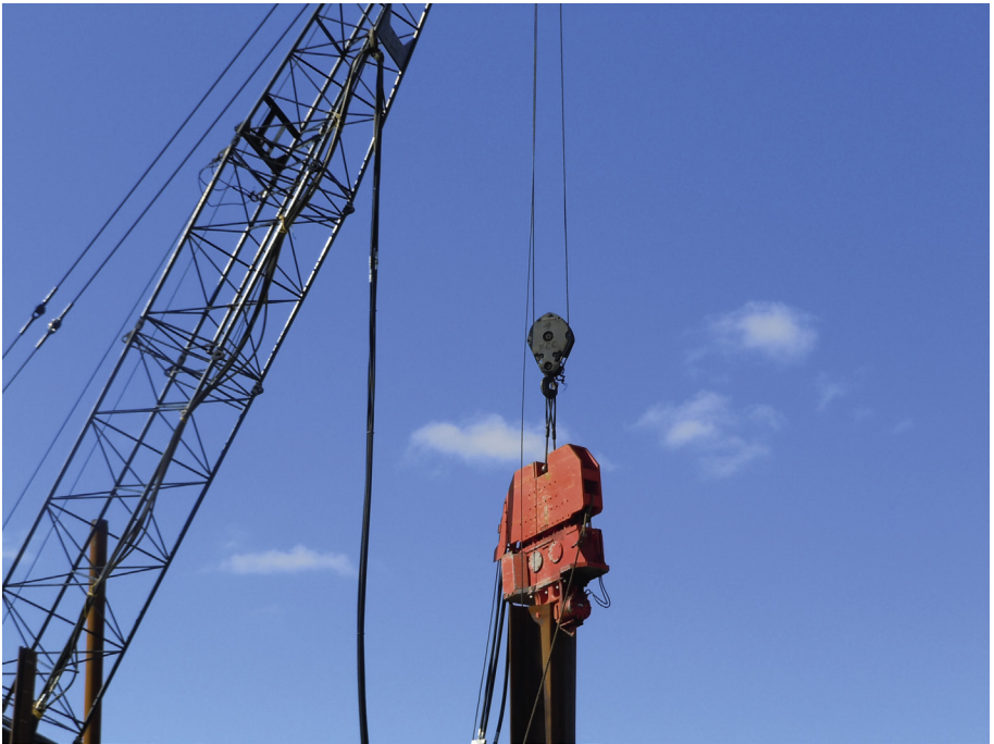
Plate 22.2 Vibratory hammer attached to a pile.
