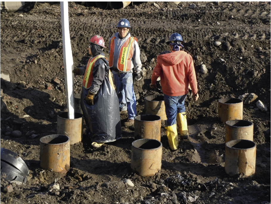
Plate 22.5 Piles cutoff to proper height.
