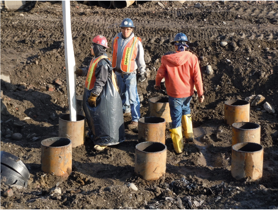
Plate 5.1 Pipe piles after installation.
