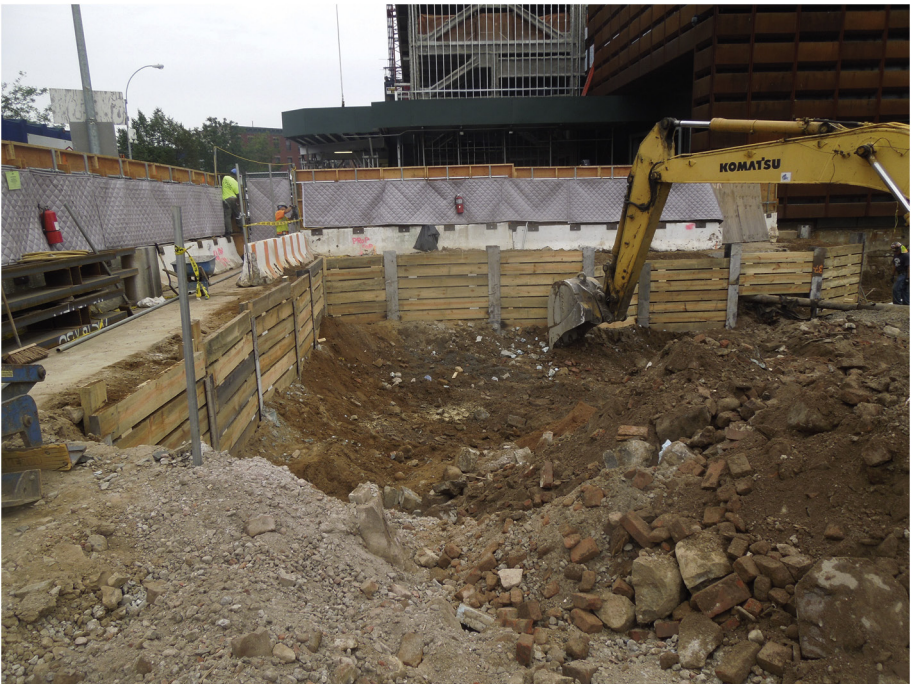
Plate 8.2 Excavation after installation of first set of lagging.
