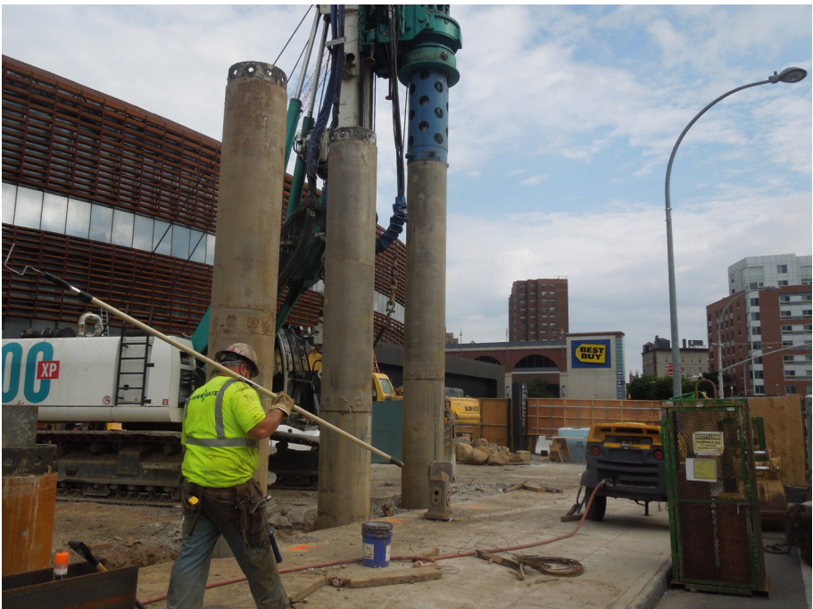
Plate 5.4 Casings are pushed into the ground.
