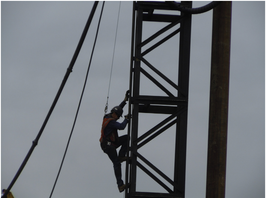
Plate 22.3 Pile lead and a pile shown here. Pile is on the right-hand side of the photo.
