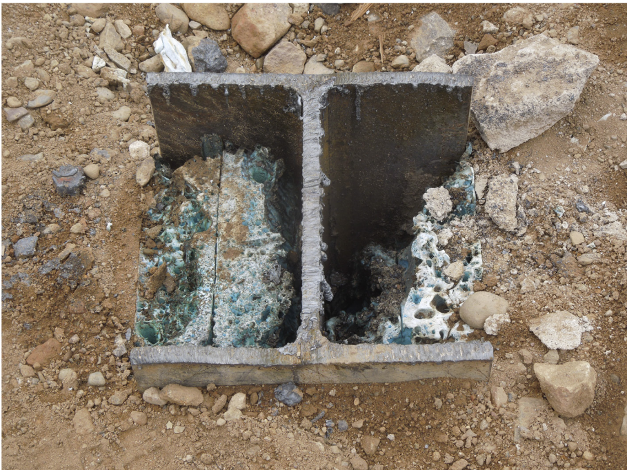
Plate 6.2 H-Pile installed in the ground.
