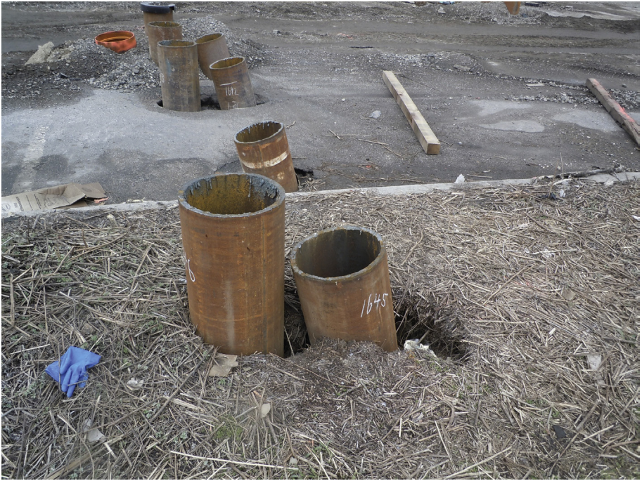
Plate 20.1 Batter piles.
