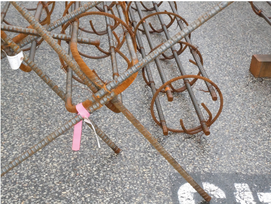
Plate 5.5 Rebar cages.
