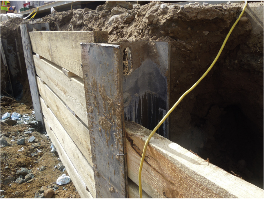
Plate 8.1 Timber laggings are installed between H-sections.
