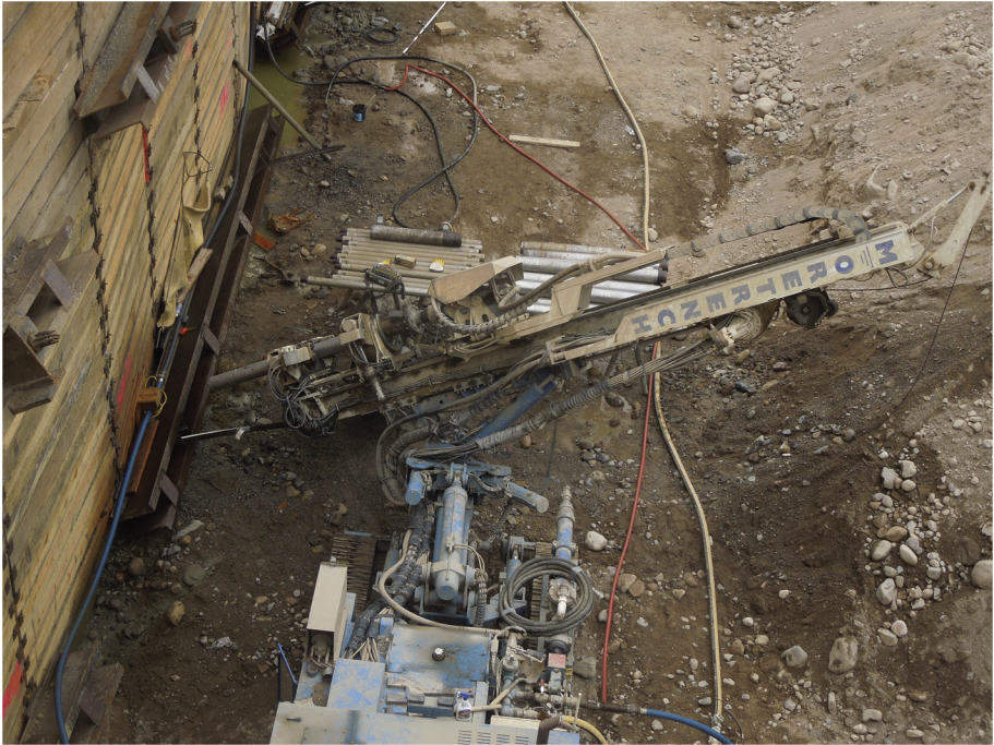
Plate 8.5 Soil anchor rig.
