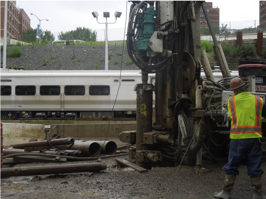
Plate 1.2 Mud rotary drill rig.
