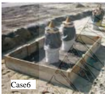
Photo. 1: Construction of subsurface ground improvement
