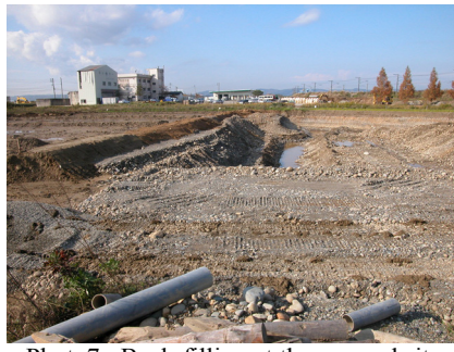
Photo 7: Back-filling at the scraped site
