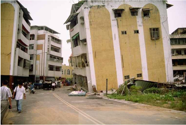
(a) 5- and 6-story buildings with foundation failures (photograph by R. B. Seed)
