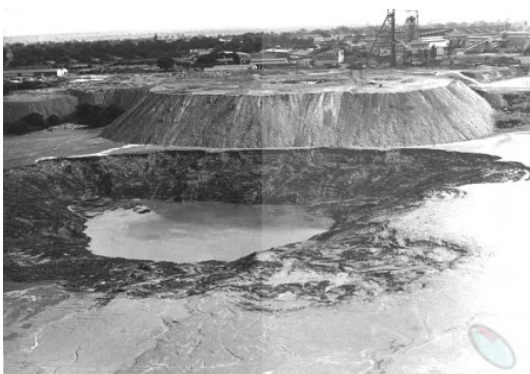
Fig. 3: Photograph of 1970 Mufulira sink hole (from [9])
