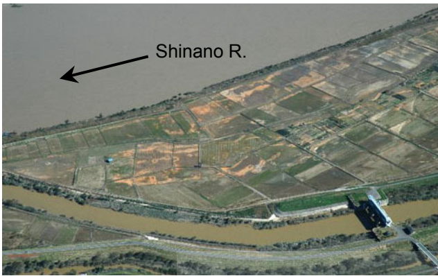
Photo 3: Aerial view of paddy field after the earthquake. Many sand boils, white threads in the photo, were observed on the field.
