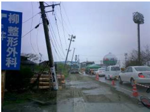
Photo 4: Tilt of electric poles and deformation of the road were found in many places where sand boiling was observed in the nearby paddy field.
