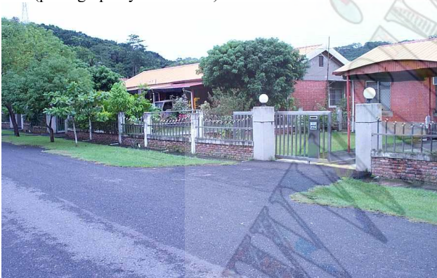
(c) 1-story buildings without evident ground failure or building settlement
