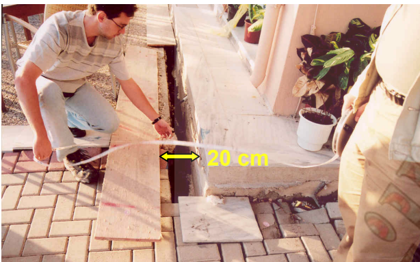
Fig. 5 : Settlement and displacement of quaywall and backfill soil in the areas “b” and “c”
