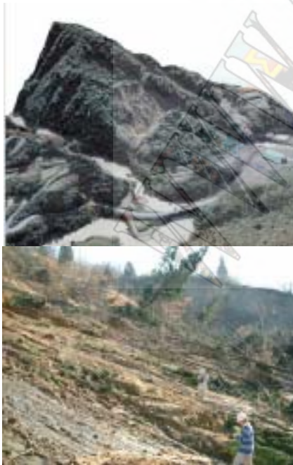
Fig.10 Aerial view of slope failure (top) and slip plane behind soil block (bottom) at Higashi-Takezawa.
