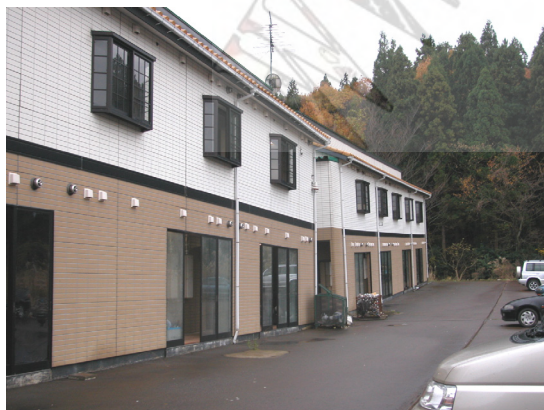
Photo 12: Residential houses suffered differential settlement at Point C in Figure 9
