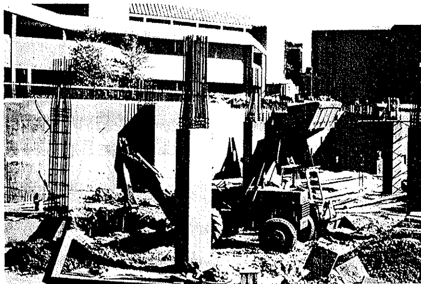
Reinforced concrete tied columns under construction; Kurt F. Wendt Engineering Library, University of Wisconsin, Madison, WI. (Photos by C. G. Salmon.)
