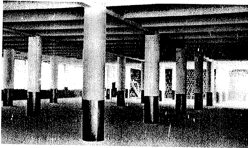
Monolithic slab-beam-girder system; Liggett and Myers Tobacco Company, Richmond, VA. (Courtesy of Portland Cement Association.)
