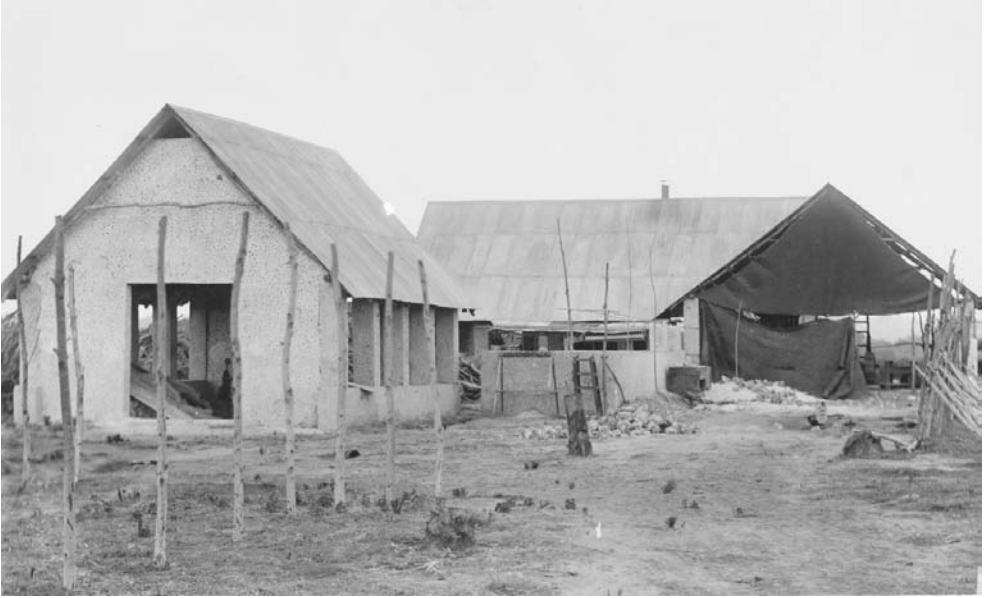
'A house for my machines under construction'
