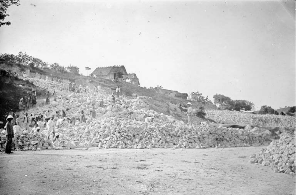
No text and no date. On the shore coral stone. See description of mortar making in chapter 6
