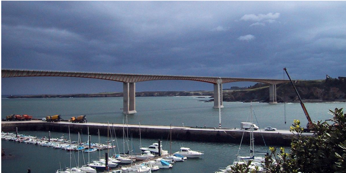
Fig. 2-10: Los Santos Bridge (Corres et al., 2008). Existing bridge comprising three 150,00 m spans, built by the cantilever method in the 1980's. The bridge deck was widened from 12,0 to 24,0 m by reinforcing the existing box cross section and using new ideas and materials in order to minimize the impact of the additional loads.
