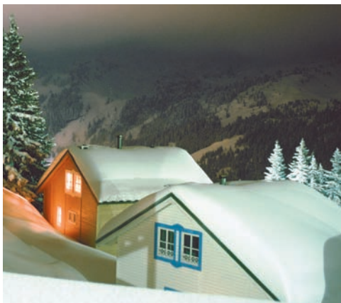
Photo 5.3 The roofs of the buildings shown must be able to support not only the total weight of the snow but also the nonsymmetric distributed loads resulting from drifting of the snow.
