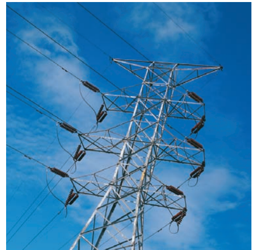
Photo 6.4 Three-dimensional or space trusses are used for broadcast and power transmission line towers, roof framing, and spacecraft applications, such as components of the International Space Station .
