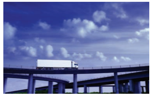
Photo 7.2 The internal forces in the beams of the overpass shown vary as the truck crosses the overpass.
