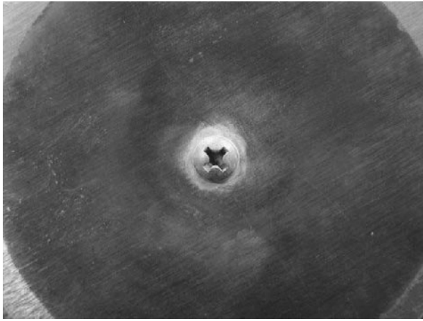
FIGURE 27.12 Galvanic corrosion where a large anode area is in contact with a small cathode area.
