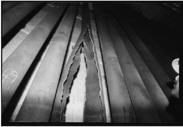
FIGURE 2.9 A close-up of the top portion of the reformer tube crack extending into the second segment from the bottom across a butt weld.
