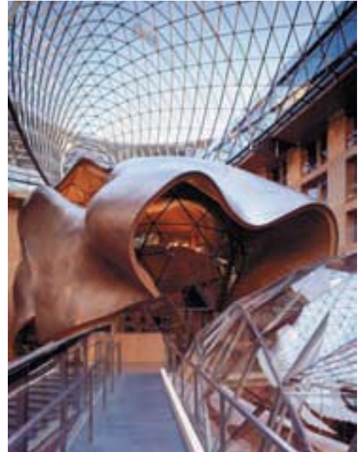
DG Bank, Berlin, Germany. Architect: Gehry
