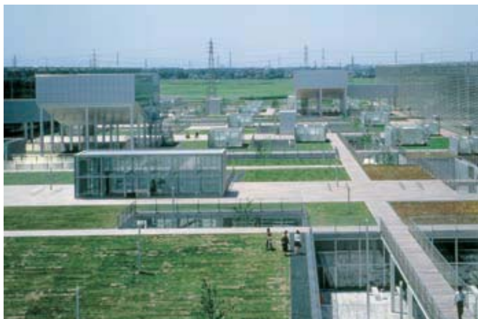
Prefectural University, Tokyo, Japan. Architect: Riken Yamamoto and Field Shop.
