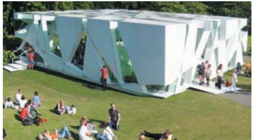
Pavilion, London. Architect:Toyo Ito & Associates
