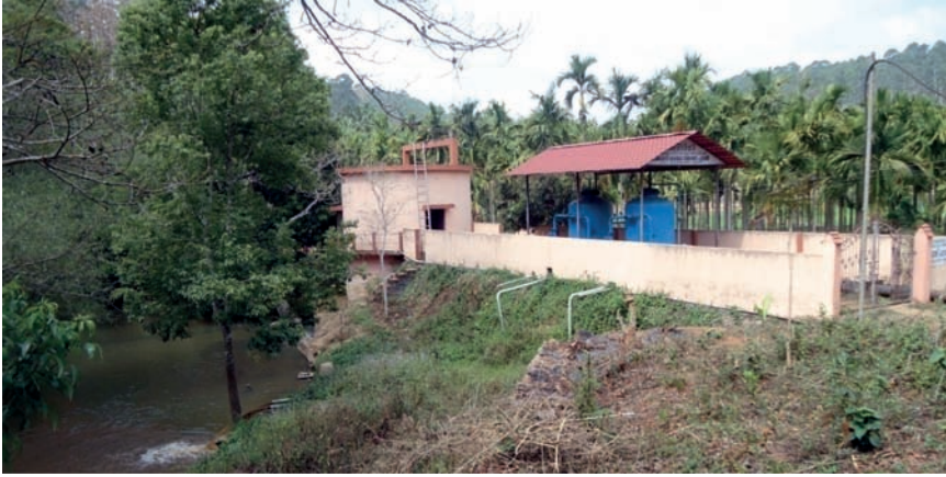
Plate 16 Village water purification plant
