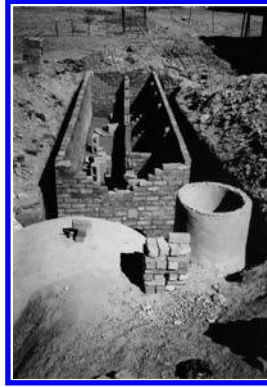
Figure 17.3. DEWATS construction in Maseru.
