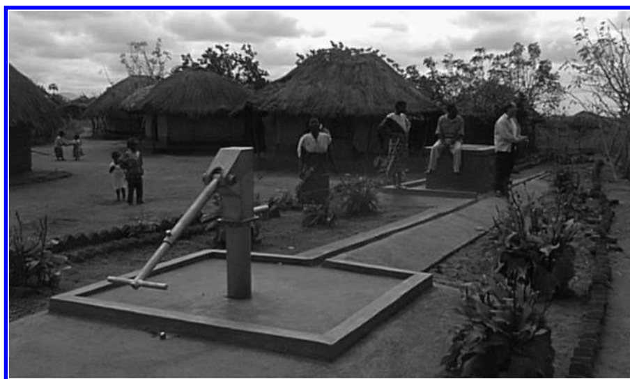
Figure 4.4. A typical wellhead protection layout in Malawi.
