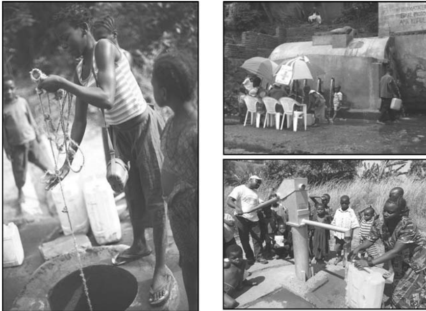
Figure 15.6. Pictures showing some means of Rural Water supply in D.R. Congo. A: Left hand, a Borehole in Nduruma; B: Upper right hand, from a captured spring in Kadutu (South Kivu), in volcanic aquifer exposed to anthropogenic pollution due to household located in the recharge and protection area of the spring; C: A communal water pump (Indian model) in Lulimba (South Kivu).
