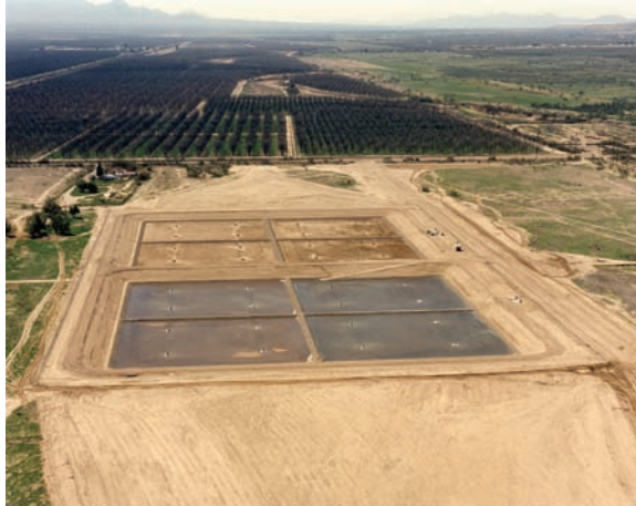
Plate 3 Pima Road recharge basin near Tucson, Arizona. (Courtesy of Central Arizona Project)
