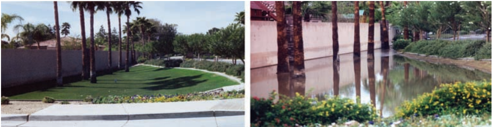
Plate 8 Example of small neighbourhood detention basin in Scottsdale, Arizona (photo by L.W. Mays)
