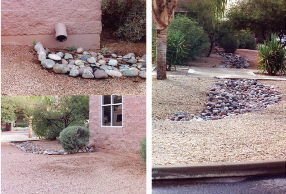
Plate 7 Showing rooftop drainage flowing into infiltration bed (photos by L.W. Mays)
