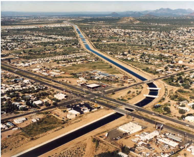
Plate 6 Central Arizona Project aqueduct through residential area in Scottsdale, Arizona (US Bureau of Reclamation)
