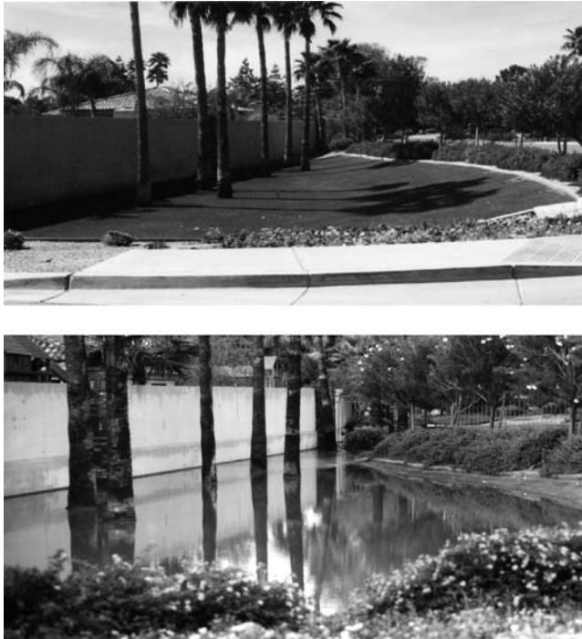
Figure 4.3 Example of small neighbourhood detention basin in Scottsdale, Arizona (photo by L.W. Mays) (See also colour plate 8)
