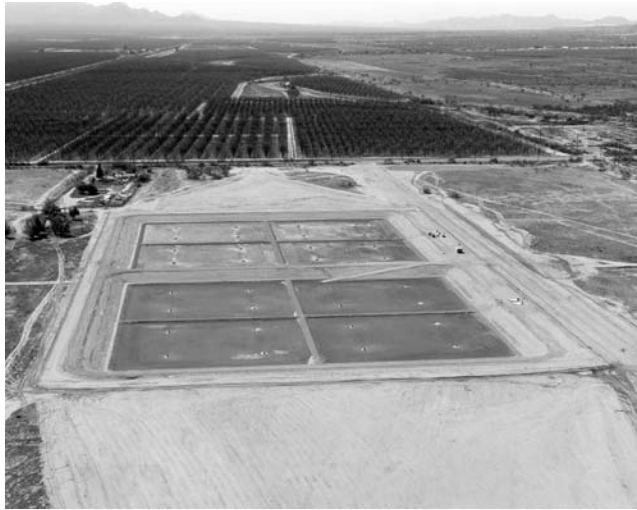
Figure 3.8 Pima Road recharge basin near Tucson, Arizona (See also colour plate 3)
