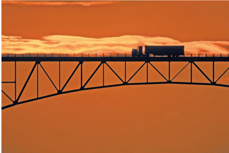
Photo 8.1 This bridge truss consists of two-force members that may be in tension or in compression.
