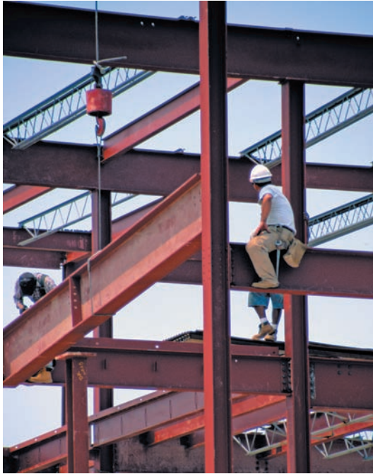
Photo 11.3 Wide-flange steel beams form the frame of many buildings.
