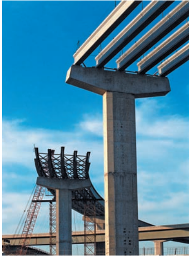
Photo 15.1 A different function M(x) is required in each portion of the cantilever arms.
