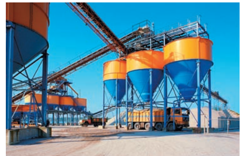
Photo 5.2 The storage tanks shown are all bodies of revolution. Thus, their surface areas and volumes can be determined using the theorems of Pappus-Guldinus.
