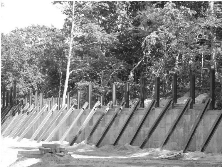
Figure 1.17 Retaining structure installed against in-place embankment shoring. Shoring braces are removed after wall has cured and reached full strength.
