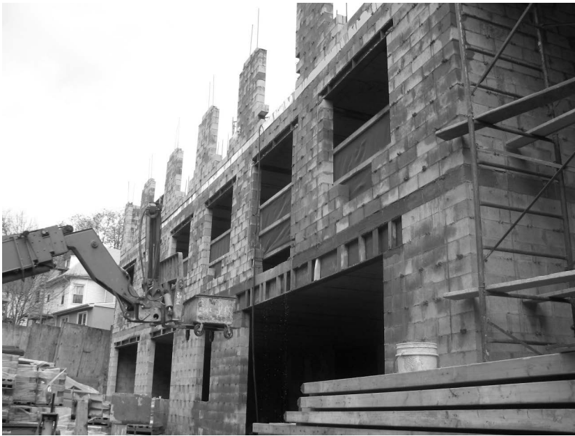
Figure 5.12 Segmented masonry shear walls with building irregularity.
