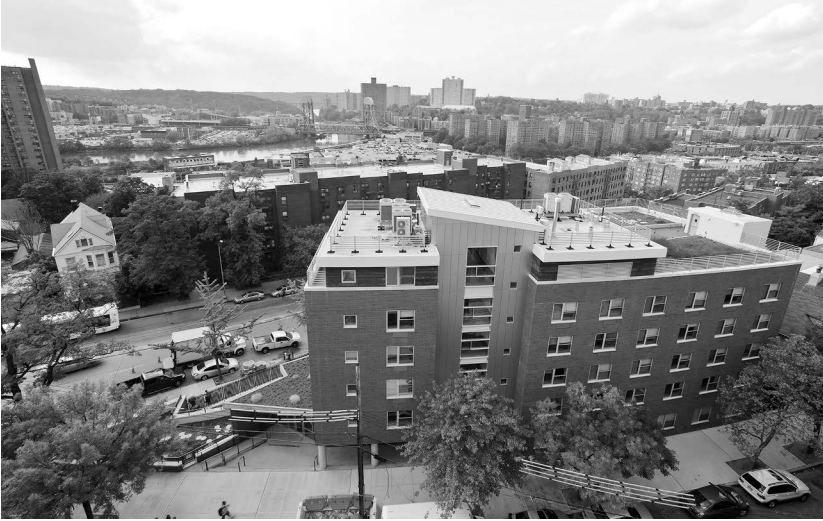
Figure 5.19 Bearing wall and frame building with horizontal and vertical irregularities.
