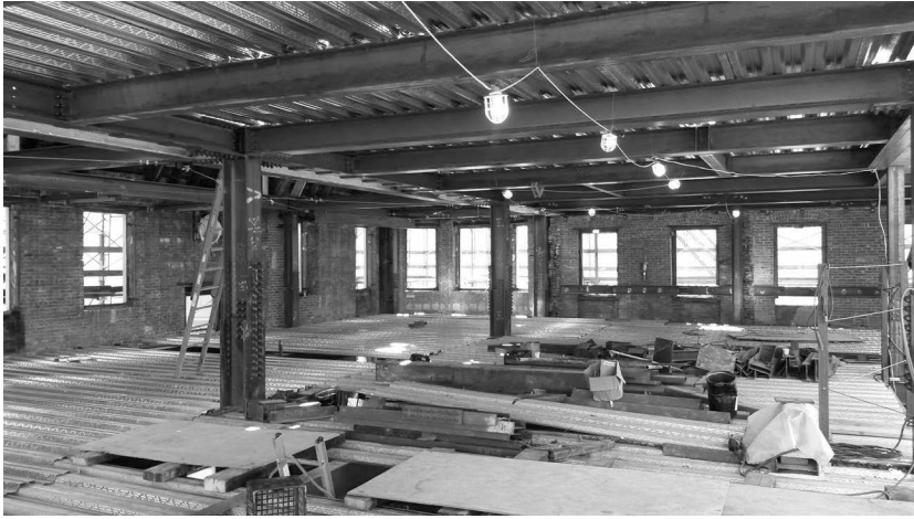
Figure 5.9 New steel and concrete building frame system being coupled with existing masonry bearing wall system.
