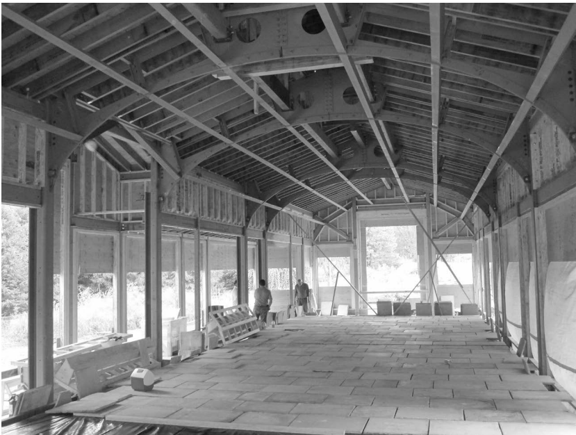
Figure 5.22 Single-story frame system integrated with wood framing.
