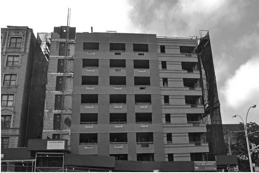
Figure 5.5 Masonry bearing wall and building frame system.
