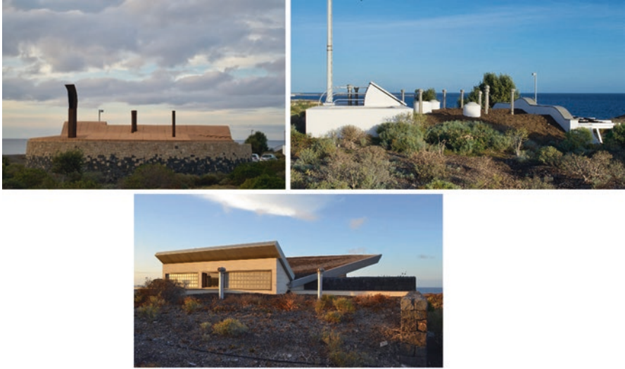
Fig. 9.11 Wind towers in the north façade of La Duna house; static chimney cowls for ventilation in Las Bóvedas and La Geoda houses
