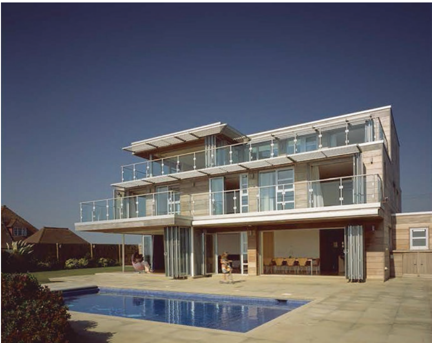
Fig. 2.14 Exterior view of south elevation showing deep eaves, cantilevered corner ceiling to ground floor living room and external pool and terracing
