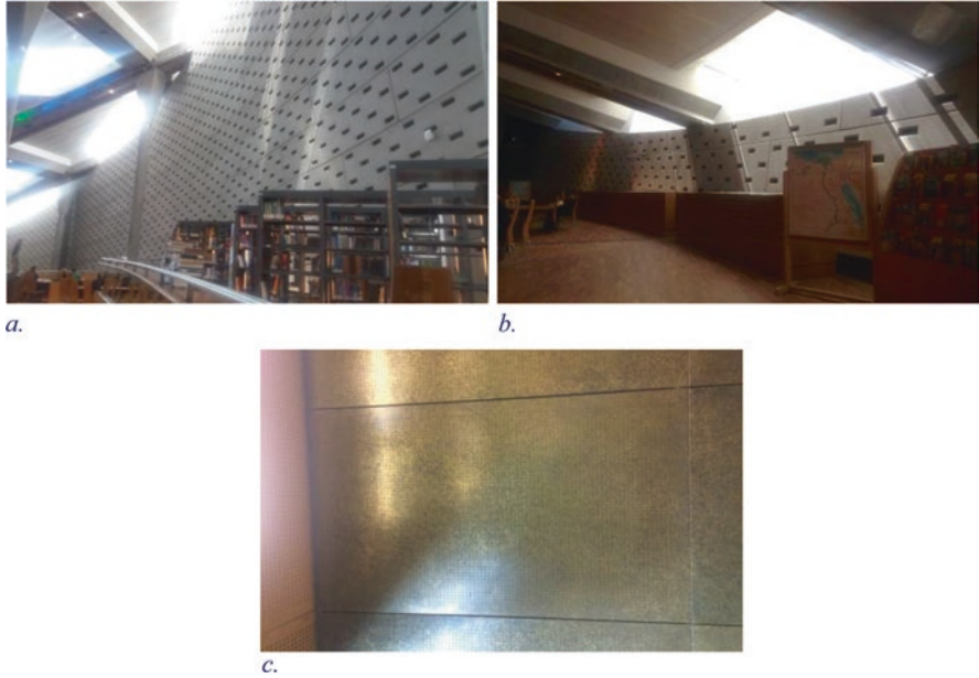
Fig. 5.27 Noise reduction using indoor acoustic materials. (a) Internal acoustic wall for sound absorption. (b) Part of the acoustic wall at the maps reading area. (c) Copper clad panels, circulation lobby (Images credit: Author)
