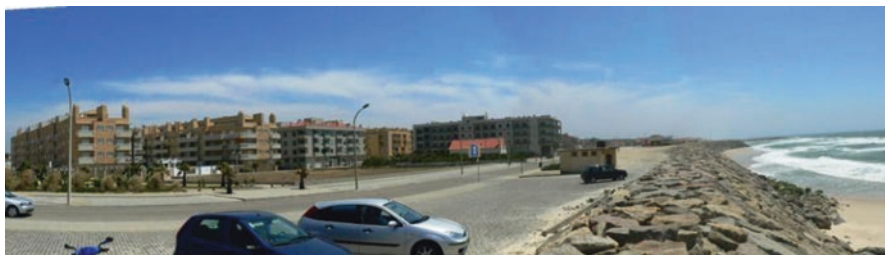
Fig. 6.12 Uncontrolled penetration of sea wind
