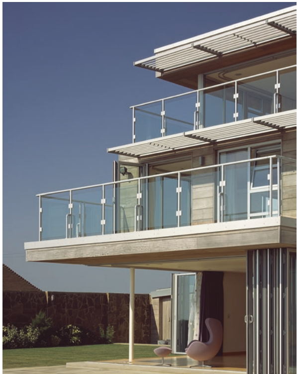
Fig. 2.12 View of south-west corner of house – illustrating the deep eaves, solar shading and materials
