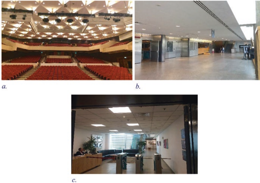
Fig. 5.32 Efficient lighting – LED lamps in the main building. (a) Conference centre with LED lamps. (b) LED lamps in the main entrance. (c) An office, in the main building with replaced LED (Images credit: BA)
