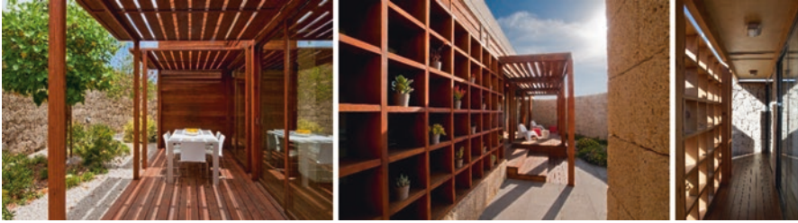
Fig. 9.15 Solar protection systems in the north courtyard and at south façade in La Geria house (Source: ITER)
