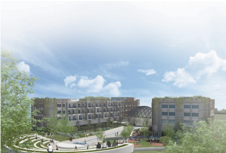
Fig. 10.9 The general view of the Eco Green Sea Site Hotel
