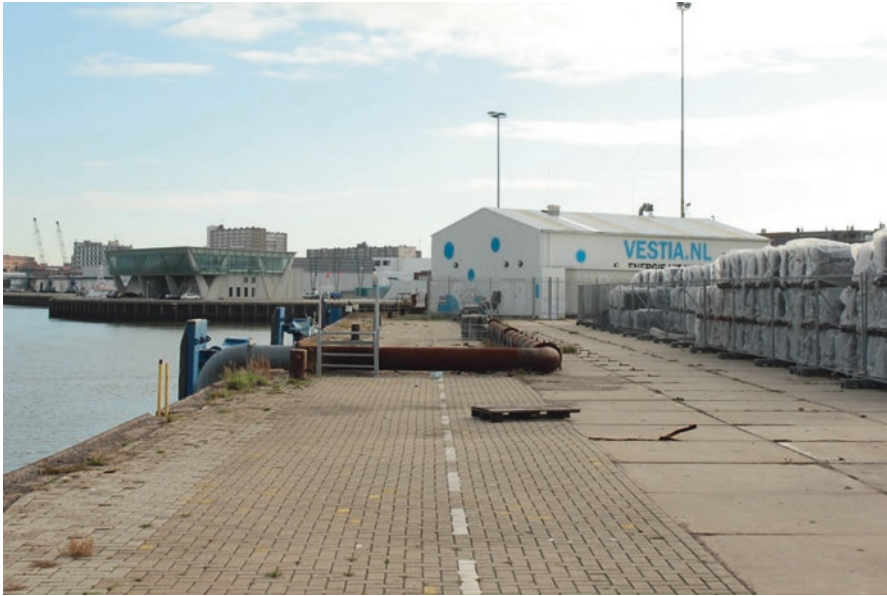
Fig. 4.16 Central heat pump using energy from the seawater to distribute it by underground pipes toward the houses
