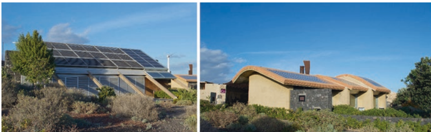
Fig. 9.12 Solar active systems in the roof of El Muro and La Duna houses
