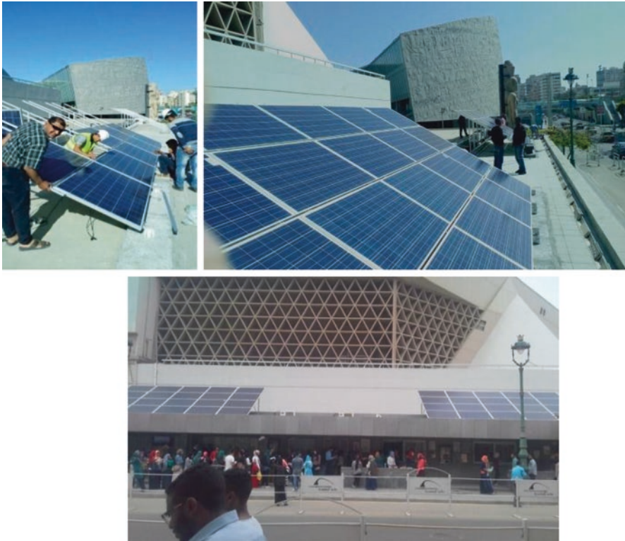
Fig. 5.33 Solar photovoltaic panels on the roof of the Library of Alexandria (Image source: BA)
