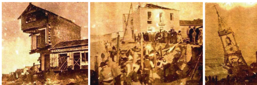
Fig. 6.9 Images from the early 1900s – collapse of buildings over sea waves
