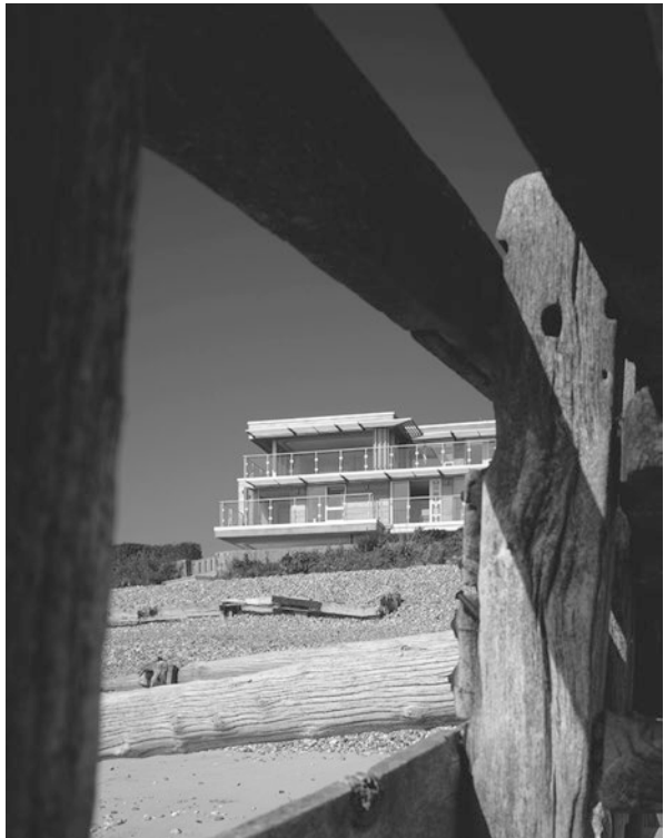
Fig. 2.11 The use of an external timber cladding system
