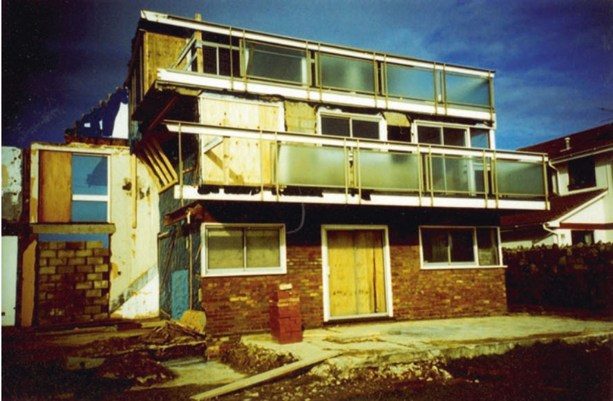
Fig. 2.8 View of the original house
