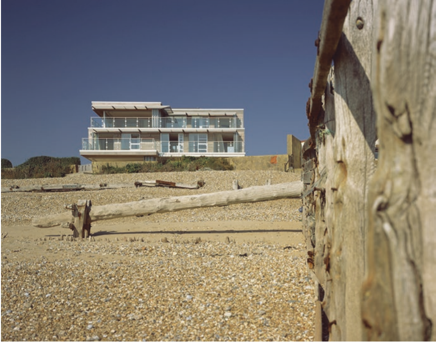
Fig. 2.1 Beach house at Bexhill
