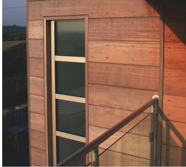
Fig. 2.24 Exterior detail – Iroko timber cladding
