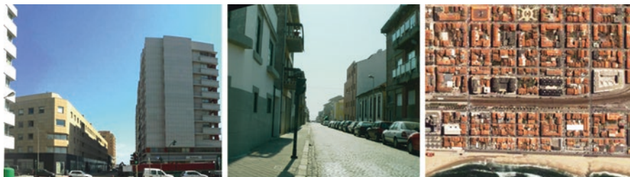
Fig. 6.11 Left , construction of concrete corridors as wind tunnels; centre , absence of trees in the streets; right , inadequate urban framing
