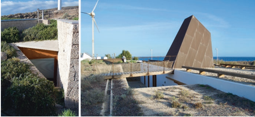
Fig. 9.10 Houses La Estrella and La Compacta , partially buried
