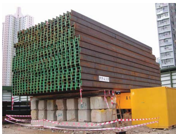
Figure 13.4 Example of use of kentledge for pile load test reaction.
