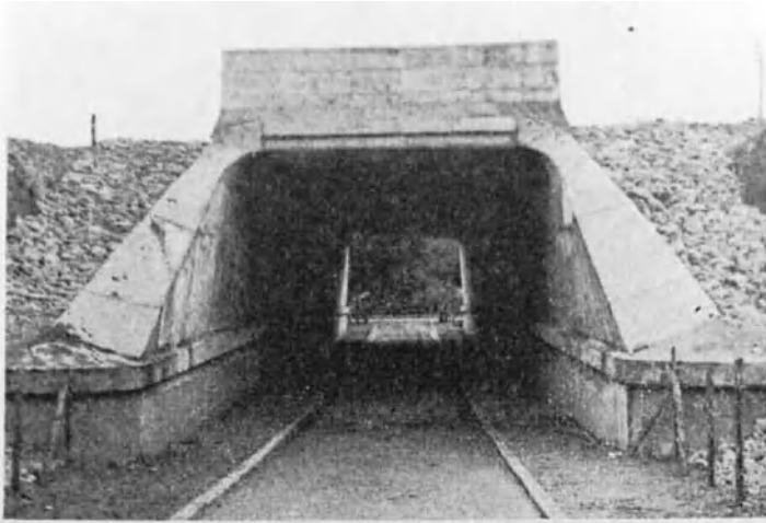
Fig. 8 (above). A square-topped underpass, marked by a solid, ornamented parapet, and with stone-pitching at the sides. Fig. 9 (below). A higher, arched concrete cattle creep, used where head-room permits, which fits in more happily and is not quite so gloomy.
