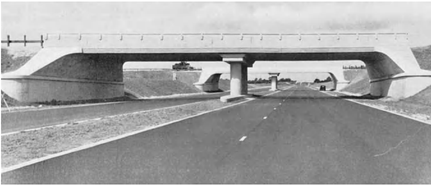
Figure 3.10 Two-span over-bridges spanning the M1 motorway. Reproduced by permission of Laing O'Rourke Plc.
