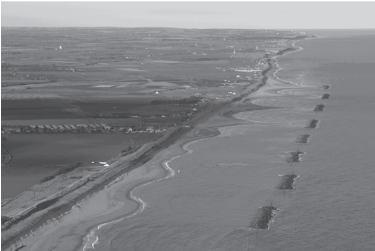
Figure 12.23 (a) Wave diffraction around the tips of two adjacent breakwaters. (b) After completion (Stages 1 and 2), showing wave diffraction and interference patterns as well as the sinuous evolution of the beach (courtesy of Mike Page)
