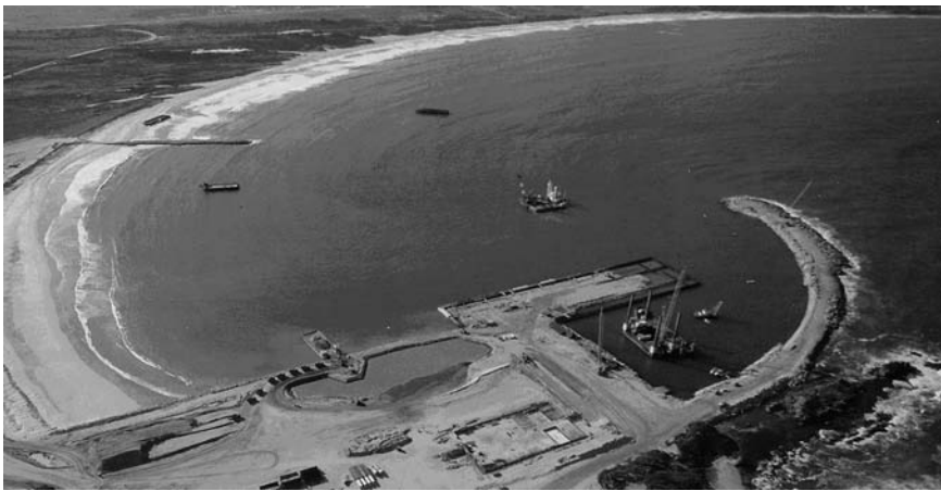
Figure 12.4 Port at Ehoala, Madagascar, showing wave diffraction, reflection and breaking near the breakwater head, and shoaling and breaking at the shore (courtesy of RTZ)
