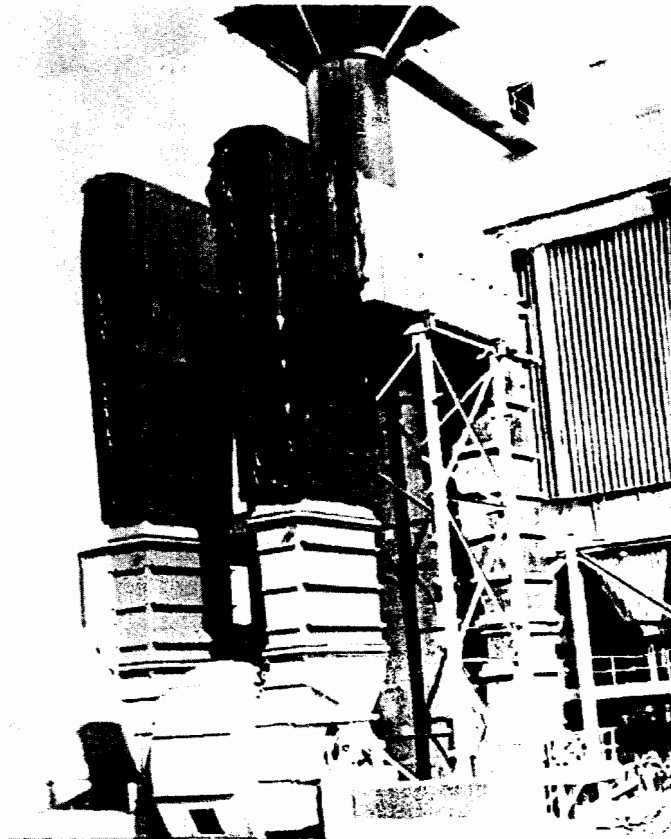
FIGURE 1.17 Fan installation in a power plant. (Barron Industries) (Note the dual-inlet ducts to supply flow to both sides of the DWDI Fan.)
