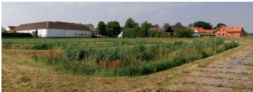
Fig. 16.1 Constructed wetland Břehov, Czech Republic (Photo author)
