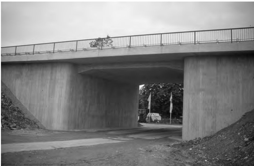
Figure 2.2 Portal frame bridge
