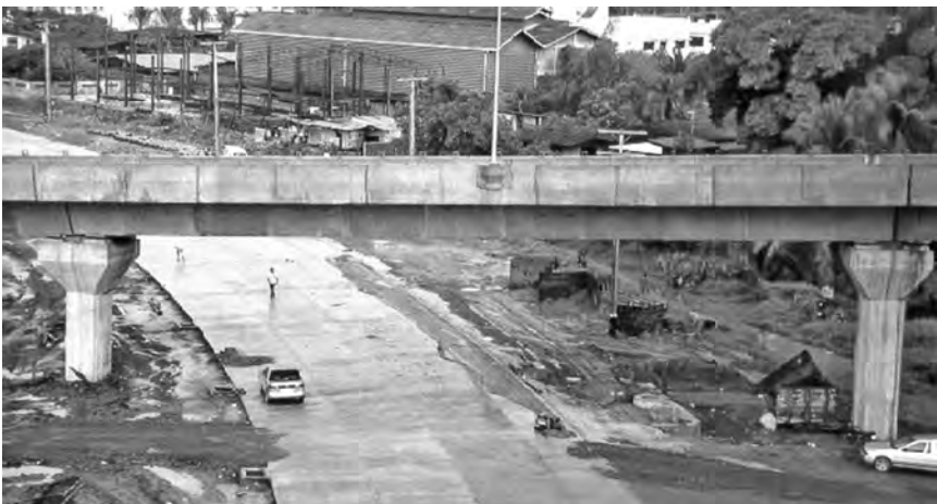
Figure 2.6 'Standard' span, Second Stage Expressway, Bangkok (Rombach, 1997)
