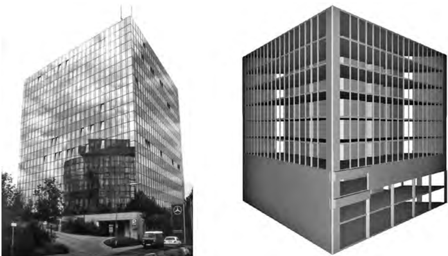
Figure 6.1 Real building and FE building models
