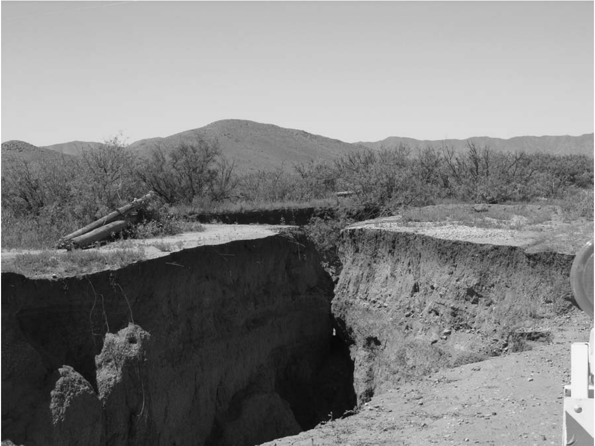
Fig. 8.2 Earth fissure due to groundwater withdrawal. This major tear in the ground (note the snapped telegraph pole for scale!) is attributed to shrinkage of the sedimentary fill of an intermontane basin near Tucson, Arizona (USA) as a consequence of heavy and sustained pumping of groundwater. (Photograph courtesy of John Callahan, United States Geological Survey.)
