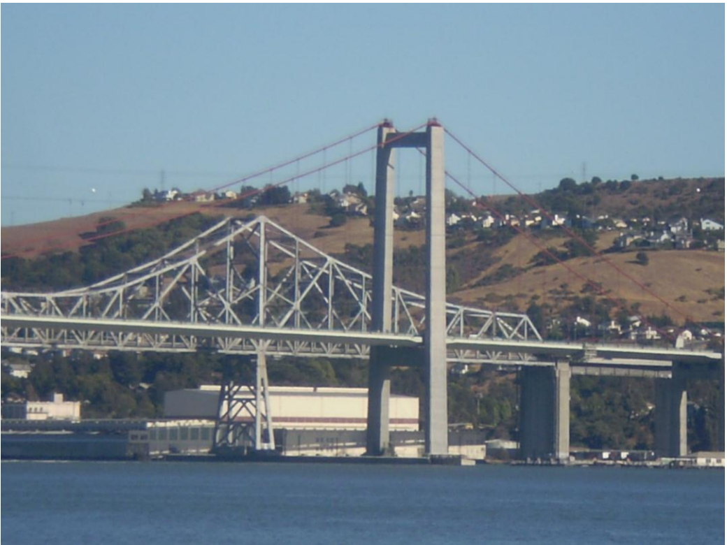
Figure B-30. Alfred Zampa Memorial Bridge (Source: Courtesy of Leon Bacud. http://en.wikipedia.org/wiki/File:Carquinez_Bridge_9-1-2007_From_Northeast.jpg )
