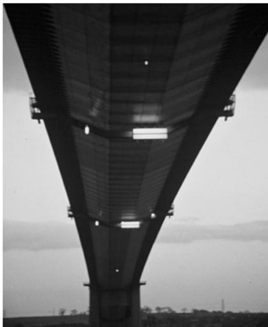
Figure 3-3. Optometer targets at Humber Bridge.
