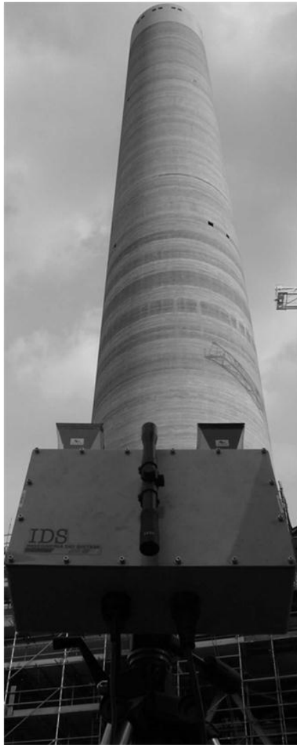
Figure 3-4. Radar system and 183m chimney
