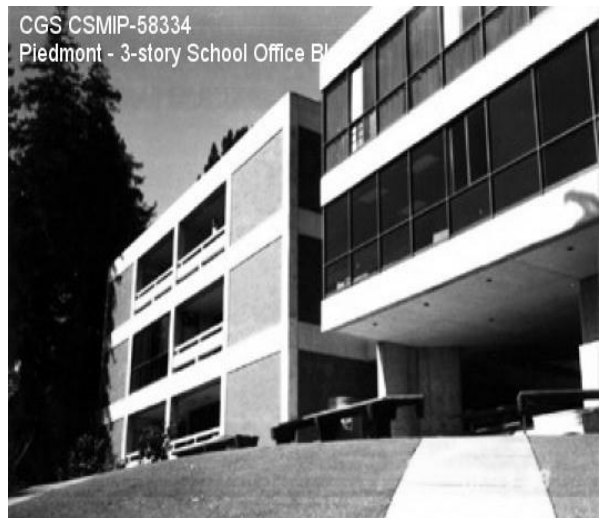
Figure A-8 Three-story Piedmont School Office Building (Source: Center for Engineering Strong Motion Data operated by CSMIP)
