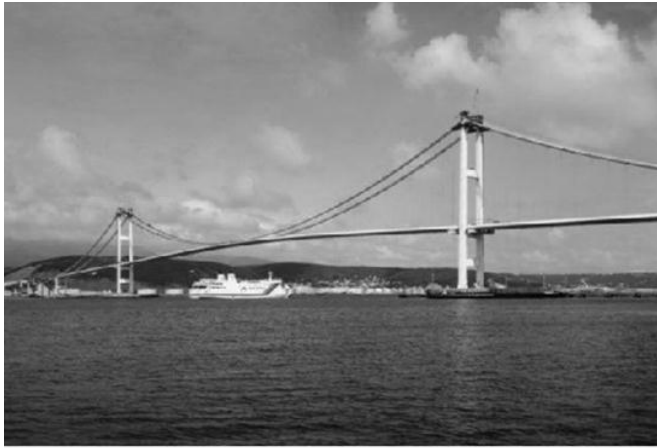
Figure B-23. Hakucho Suspension Bridge
