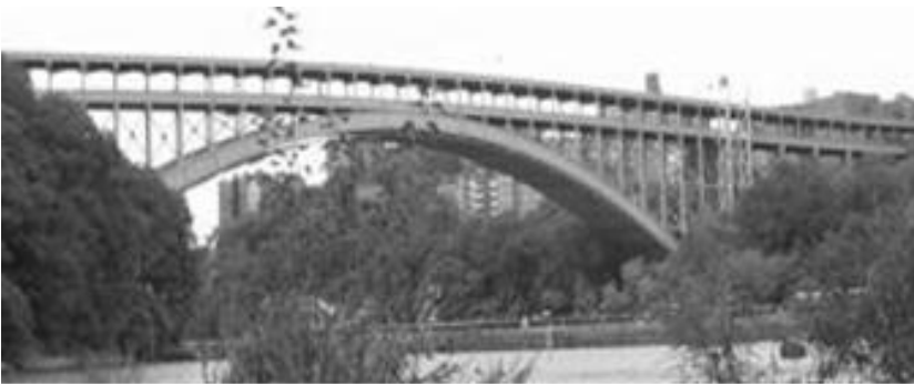
Figure B-1. Henry Hudson Bridge
