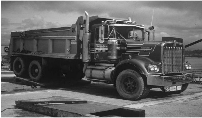
Figure 3-2. Vehicle impact (Annacis Bridge, Vancouver)
