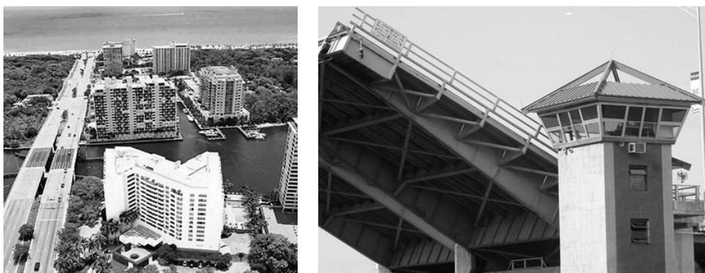
Figure B-40. Sunrise Boulevard Bridge in Florida
