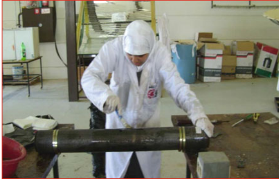
Fig. 3 Photograph of the beginning of the over-wrapping
