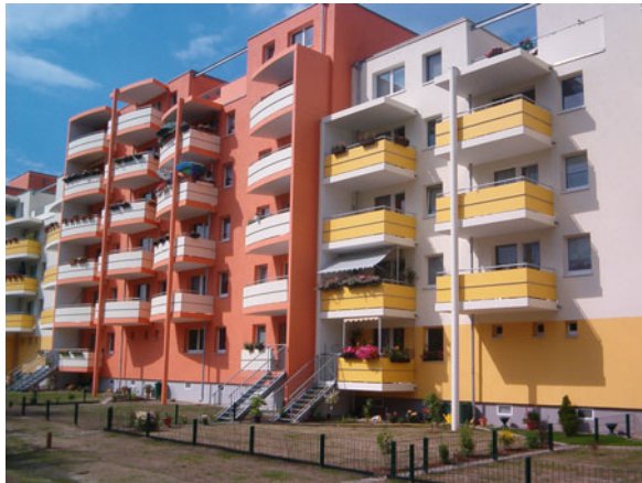
Fig. 9.2 Marzahn-Nord after reconstruction
