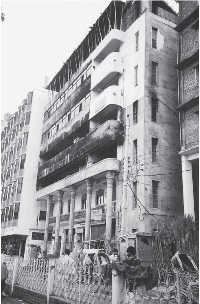
Figure 5. Outside the Tri Model/Suntex factory complex in Dhaka, three months after the fire. Jute cloths have been placed in the window frames in lieu of windows. Even though the floors are burned out, work continues inside.
