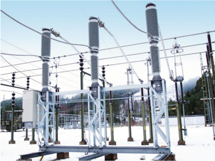
Fig. 6.13 Circuit-breaker filled with 10 bar CO 2 and rated for 72.5 kV. In this pilot installation, it operates in the 145 kV system (Courtesy of ABB)
