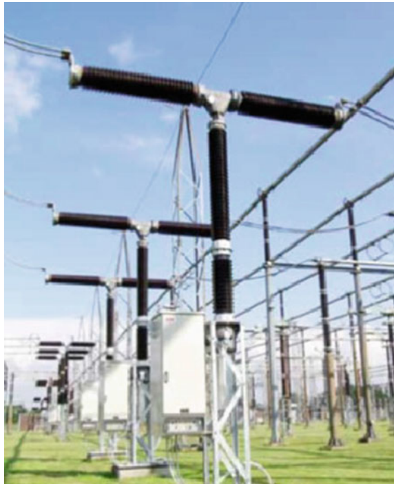
Fig. 4.23 Modern single pressure 420 kV SF 6 circuit breaker (Courtesy of ABB)
