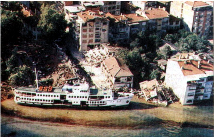
Fig. 1. Damage from the earthquake 1999, tectonic subsidence, ground liquification and the tsunami. The ship in the foreground thrown onshore by tsunami wave action. (Kandilli Observatory and Research Institute, www.drgeorgepc.com/Tsunami1999Turkey.html , accessed on 14.04.08)
