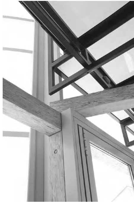
Figure A.14 Detail of the overlaying of elements in the main sunspace.
