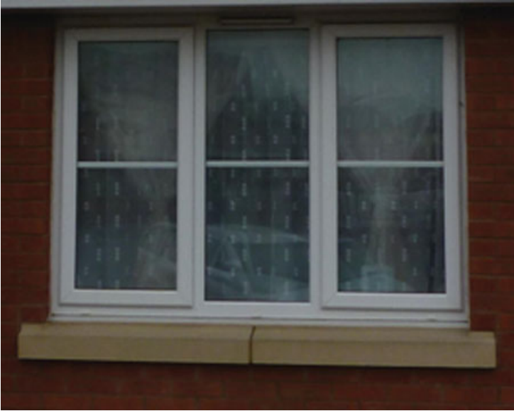
Figure 4.15 External view of window (iv).
