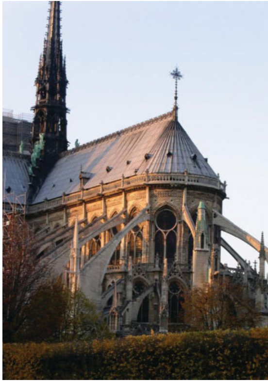
Figure 1.1 Notre Dame de Paris, illustrating the technical mastery, the depth of understanding and the pure technical design genius of the flying buttress.
