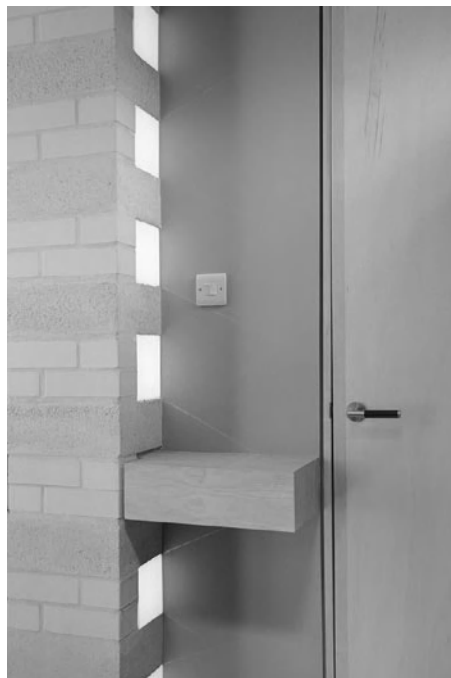
Figure A.13 Purpose made LED lighting to the larder entrance.
