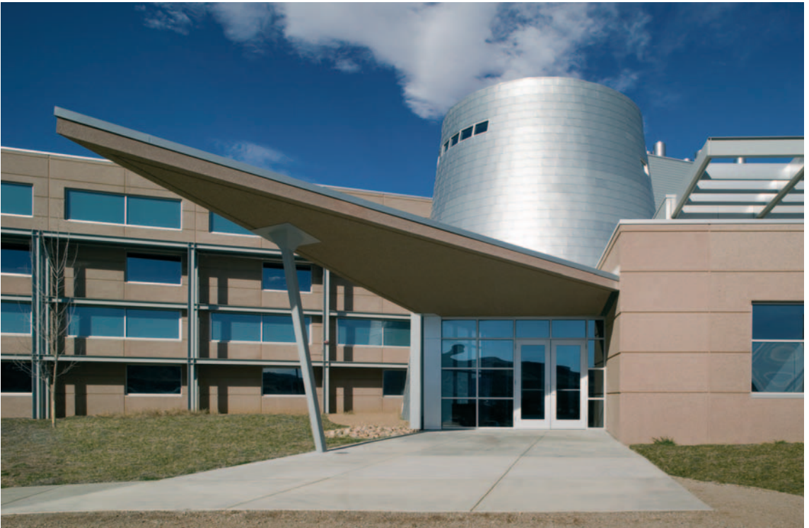
▲ 5.6 Designed by SmithGroup, the Science & Technology Facility at the US Department of Energy’s NREL is LEED-NC Platinum certified. Photography by Bill Timmerman. Courtesy of SmithGroup.
