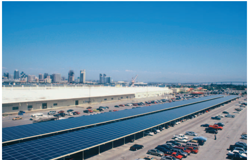
► 7.3 The 924-kilowatt PV system installed by PowerLight on the carport at the US Naval Base in Coronado, California generates enough energy during the day to power over 935 homes. Courtesy of SunPower Corporation.
