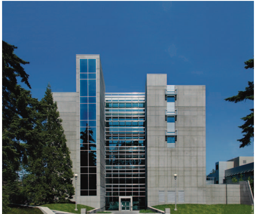
► 5.5 The ECS Building on the University of Victoria campus operates at 51 percent below Canada's National Energy Code. Courtesy of Busby Perkins+Will.
