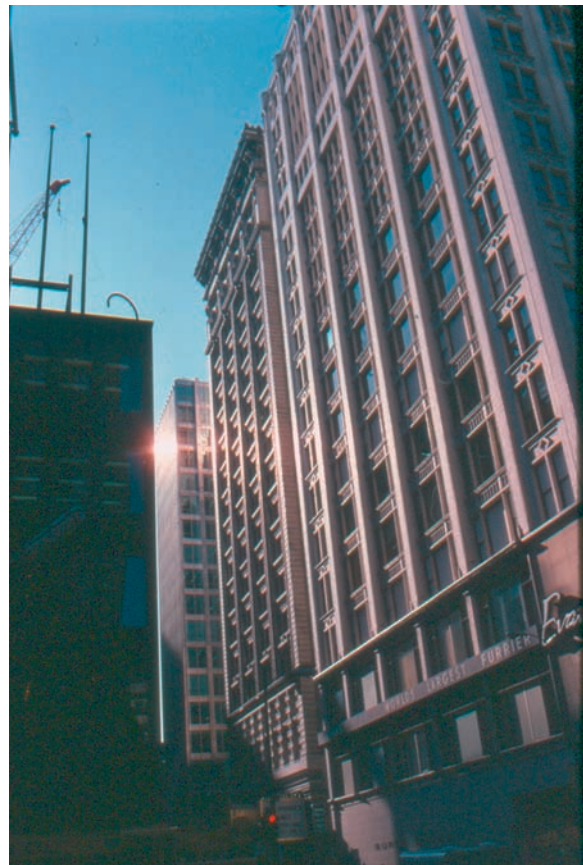
Figure 3 Steel-framed buildings in 'the Loop', Chicago.
