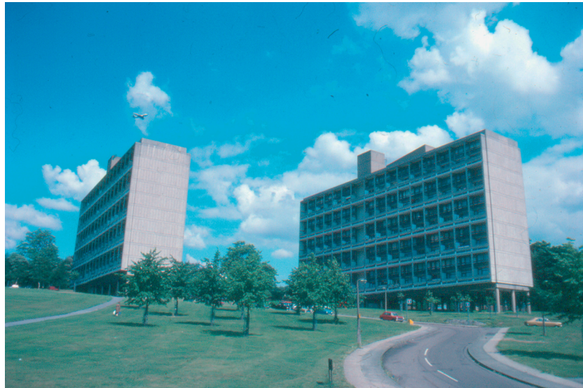
Figure 4 Flats at Alton West, Roehampton, London (LCC Architects Department, 1954–1958).
