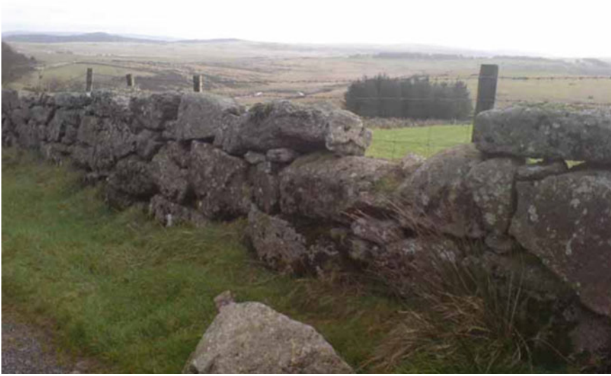
Fig. 6 Drystone wall, skipton Source Vaughan 2010
