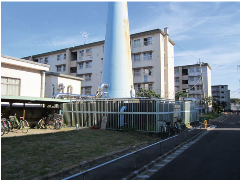
Fig. 7.2 Repaired main water pipe in Tatsumi apartments (Sep. 8, 2011)
