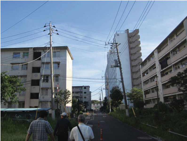
Fig. 7.4 Temporary repaired infrastructure, Tatsumi apartments (Sep. 8, 2011)
