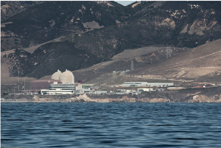
Fig. 11.1 The Diablo Canyon Power Plant, north of Avila Beach, in San Luis Obispo County, California (courtesy of ML Baird)
