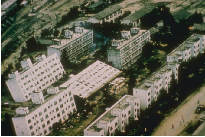
Fig. 7.6 Inclined apartment buildings at Kawagishi-cho in Niigata due to soil liquefaction, after the M_w 7.6 magnitude Niigata earthquake, Japan, 16 June 1964
