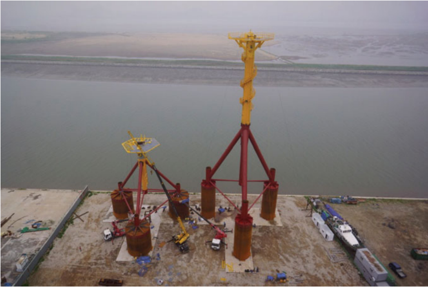
Fig. 26.1 Suction piles supporting tripod substructures [1112]
