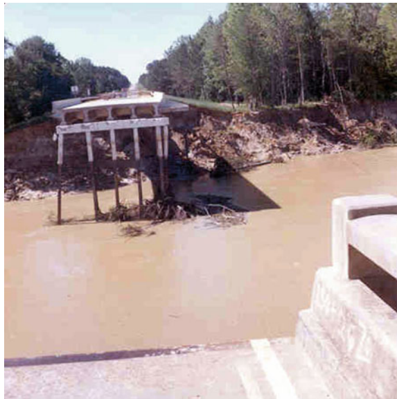
Fig. 20.5 Illustration of scour at the bottom of a bridge foundation
