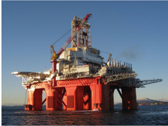
Fig. 9.3 A floating drilling platform Aker H6e (courtesy of Aker Solutions)
