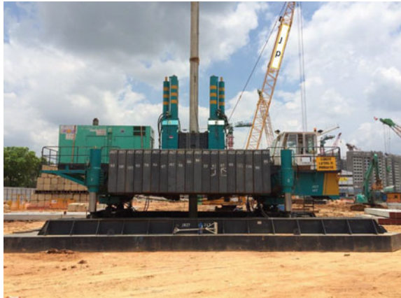
Fig. 14.5 Operation of pile jacking. (Courtesy of Geotechnical Society of Singapore)
