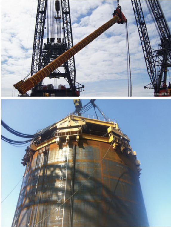
Fig. 14.4 Installation of steel piles at sea using large vibratory pile drivers, upper figure: CAPE Vibro 320 Vibro Lifting Tool—used for installing piles with a diameter of 2.1 m and a length of 45 m in the North Sea; lower figure: 8xAPE 600B for installing piles with a diameter of 22 m and a length of 50 m for Macau bridge. (Courtesy of L. de Neef, P. Middendorp and J. Bakker, Netherland, photo by L. de Neef, CAPE Holland)
