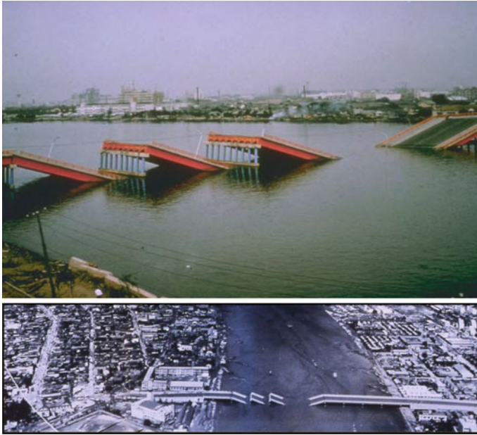
Fig. 7.7 Collapse of Showa Bridge during Niigata earthquake
