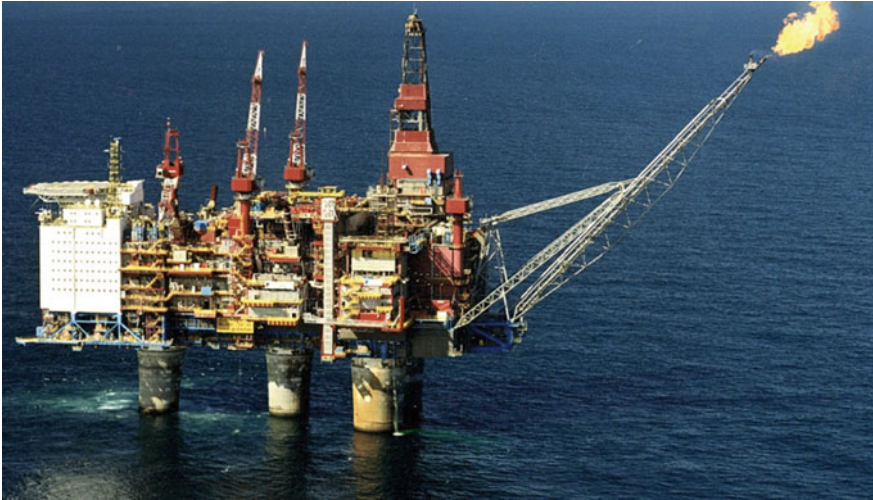
Fig. 1.31 Gullfaks C platform with a topside weight of 74,000 tons
