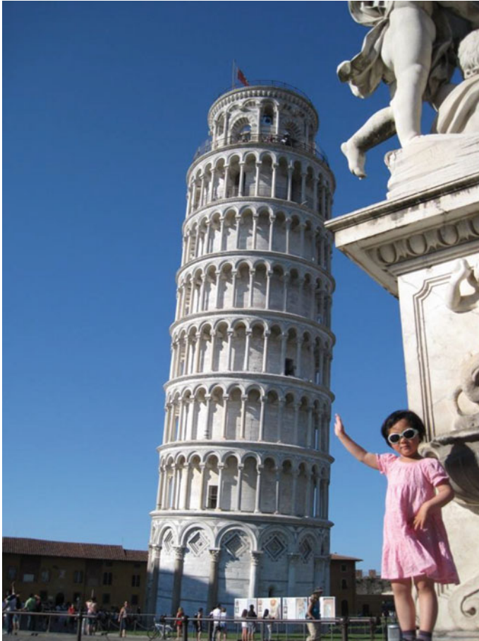
Fig. 1.1 Leaning Tower of Pisa, with a height of 55.86 m
