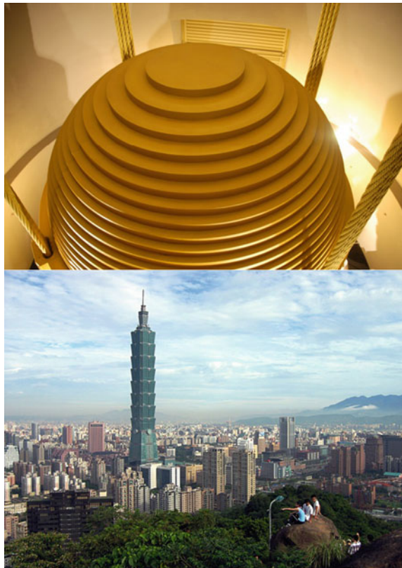
Fig. 9.32 A tuned mass damper (upper) suspended from the 92nd to the 87th floor at Taipei 101 (lower) (under licenses of CC BY-SA 3.0 by Guillom and Peellden)
