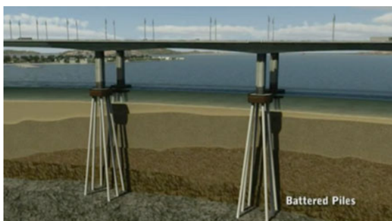
Fig. 14.7 Battered piles support a precast segmented skyway of the San Francisco-Oakland Bay Bridge where upper soil layers are weak muds
