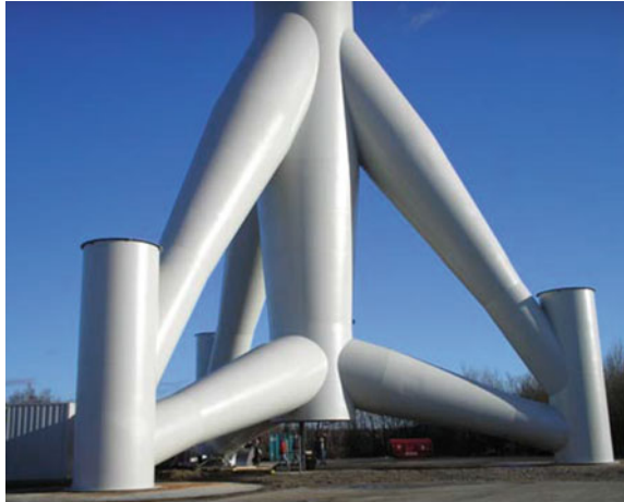
Fig. 9.17 A close look at a tripod used as a substructure for OWT (courtesy of Aker Solutions)
