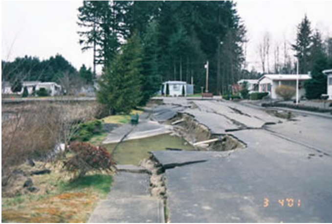
Fig. 7.5 Lateral spreading due to soil liquefaction (courtesy of USGS)
