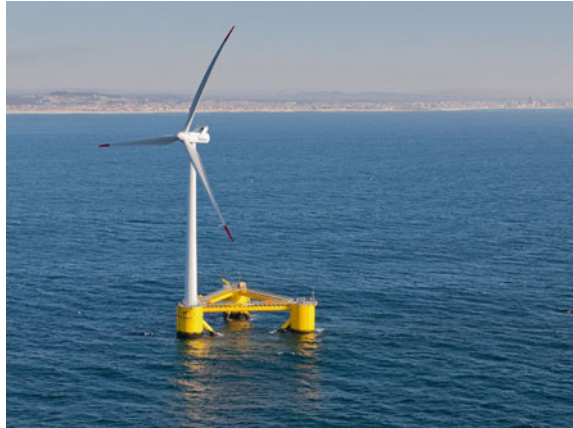
Fig. 9.16 WindFloat, which is a semi-submersible structure for an OWT operating at a rated capacity of 2 MW approximately 5 km offshore of Aguçadoura, Portugal (under license CC BY-SA 3.0 by untraktrover)
