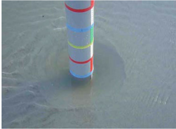
Fig. 20.3 Steep-sided local scour pits around a monopile foundation
