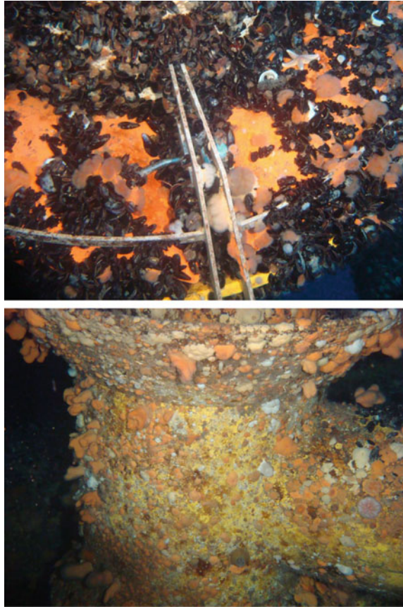
Fig. 9.41 Marine growth at water depths of 14 m (upper) and 41 m (lower) on an offshore jacket structure in the North Sea
