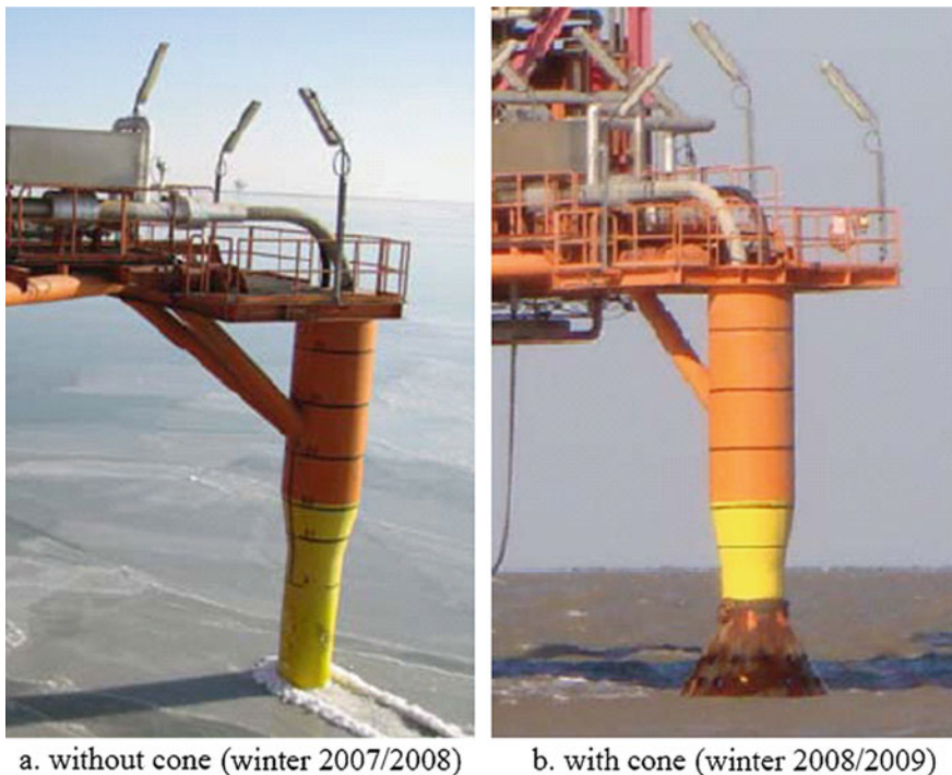
Fig. 10.1 A monopod structure with vertical leg structure (left) during the first winter, later modified with an ice-breaking cone (right) installed during the second winter [528]
