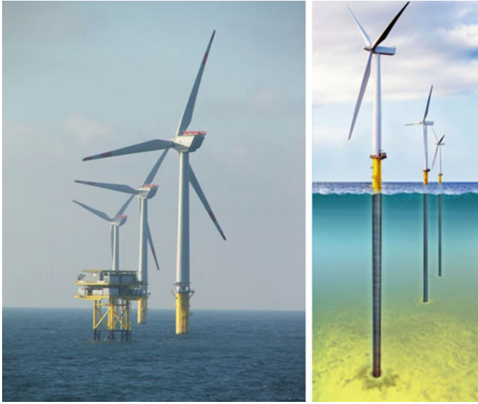
Fig. 15.9 Monopile structures supporting offshore wind turbines
