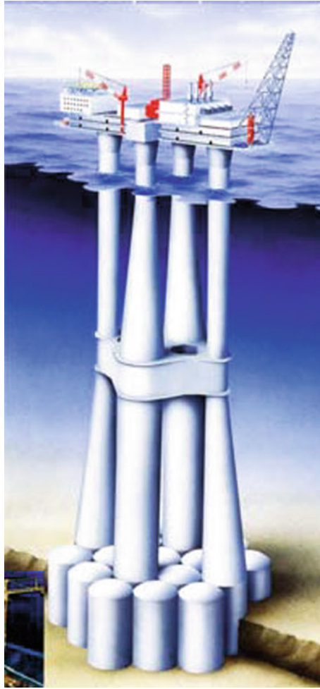
Fig. 26.7 Troll A platform (481 m high) with a skirt suction foundation
