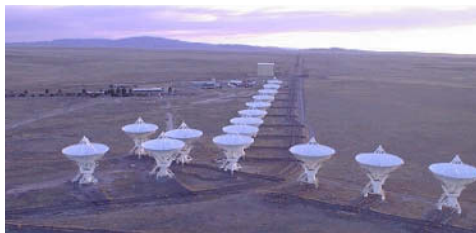
FIGURE 3-13 The Very Large Array. SOURCE: Photo by Dave Finley, NRAO/AUI.
