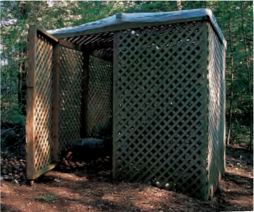
The author's shade house is an 8-foot (2.4-meter) square simply constructed structure using wood lath and 4- x 4-inch (10- x 10-cm) pressure treated wood posts.
