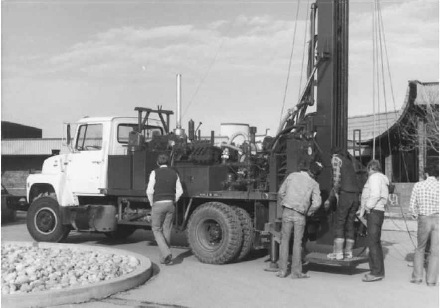
FIGURE 2.5 Truck-mounted drilling rig.
