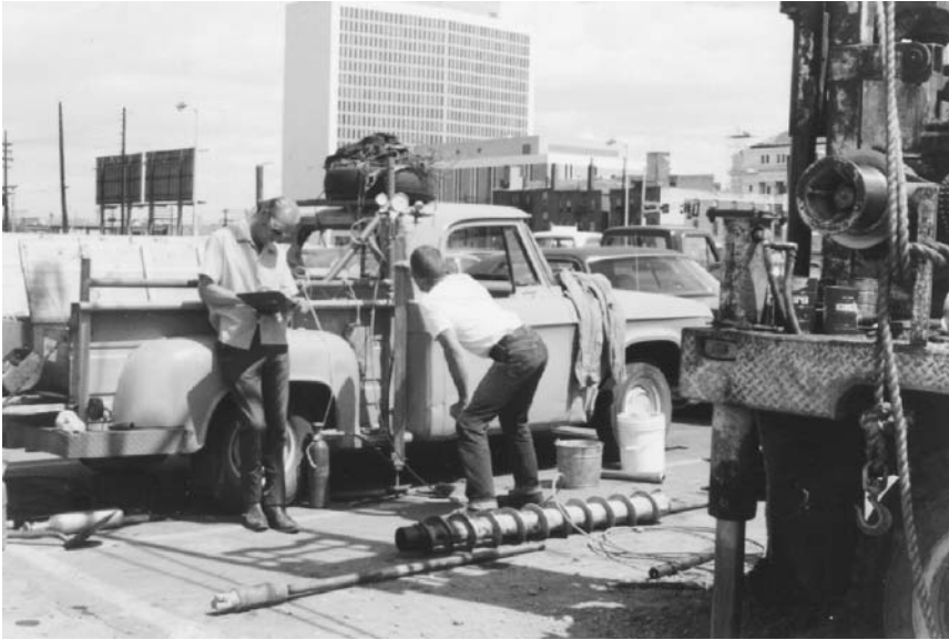
FIGURE 3.1 Drilling for pressuremeter test.
