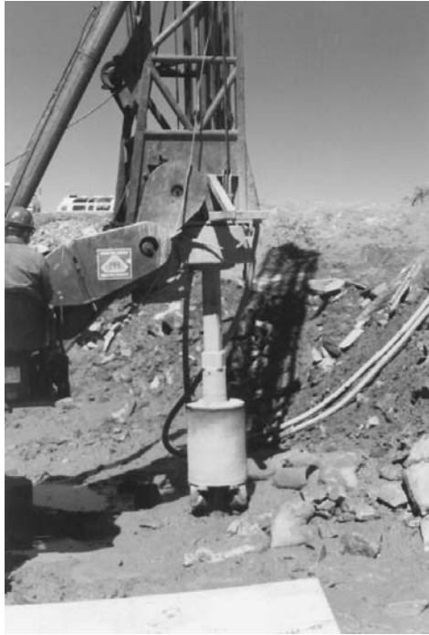
FIGURE 2.1 Caisson rig with a rock bit.
