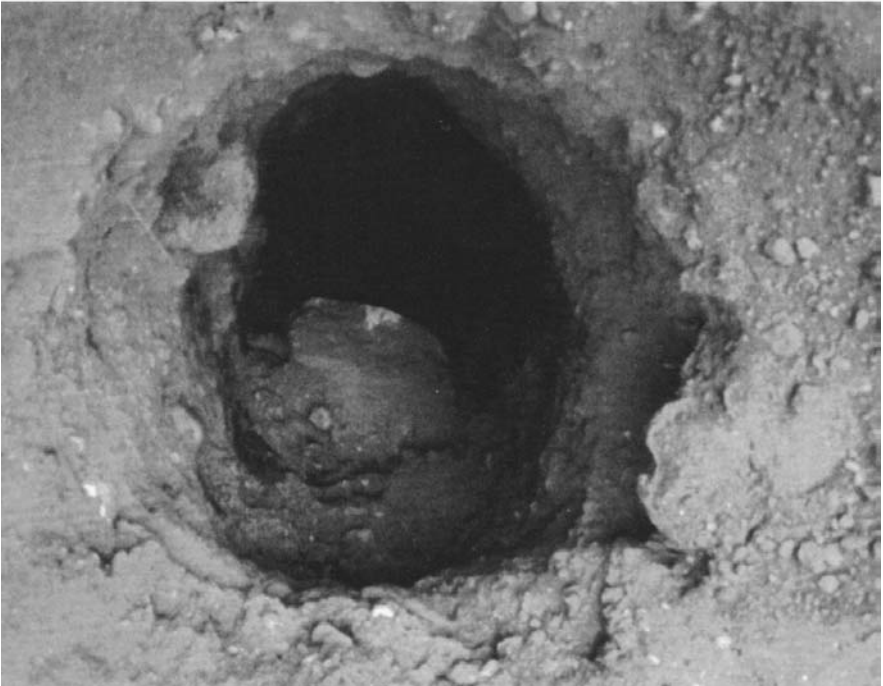
FIGURE 17.1 Boulder in the drilled pier hole.
