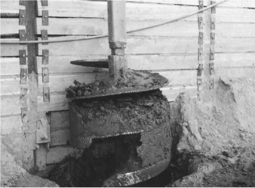
FIGURE 10.3 Large-diameter pier drilling for a high-rise building.
