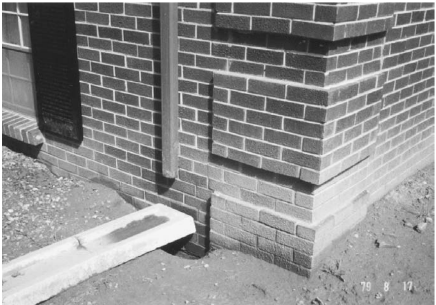
FIGURE 13.9 Down spout drain into backfill.
