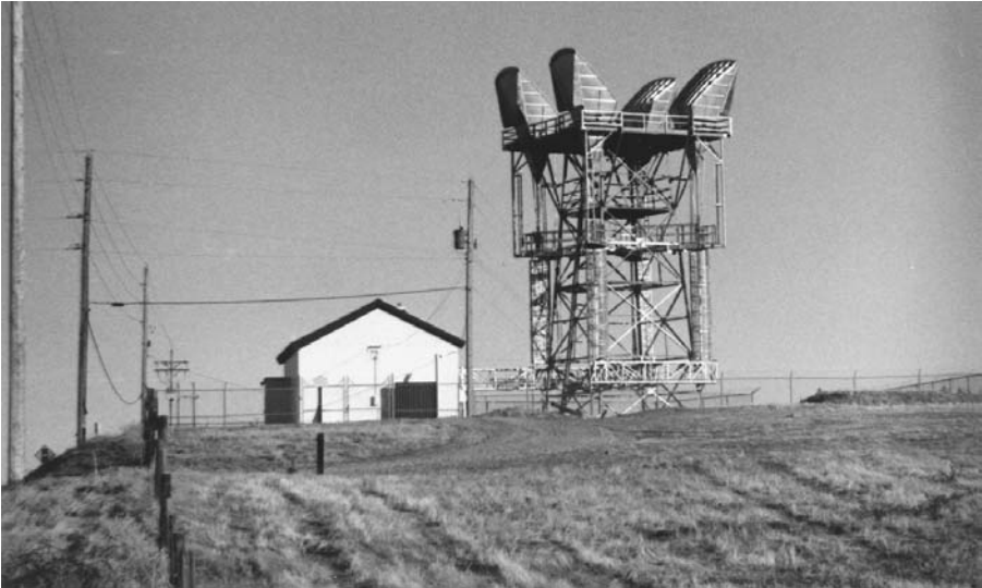
FIGURE 11.12 Microwave tower on piers subjected to lateral load.
