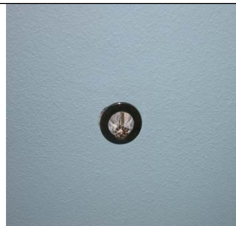
Sprinkler head finishing rings held in place by friction came off during the quake at Del Mar Elementary.
