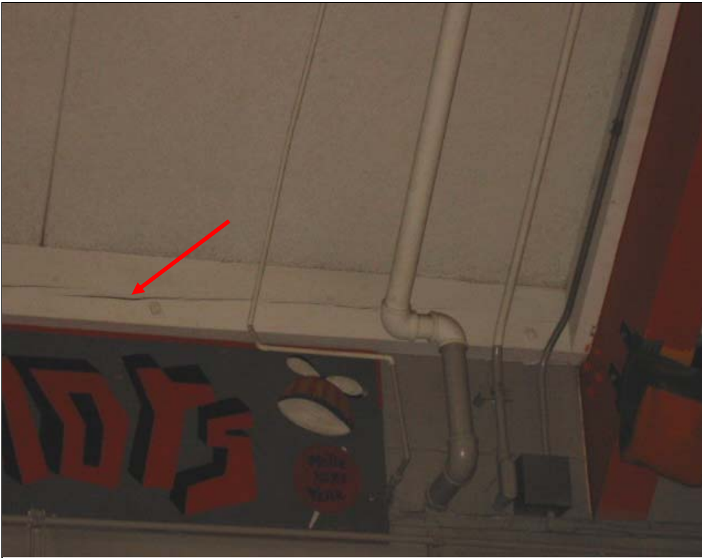
Ledger cracking was observed at the Atascadero High School gym building at the roof connections
