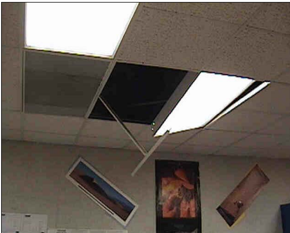
T-bar cross runner popped loose at Paso Robles High School.
