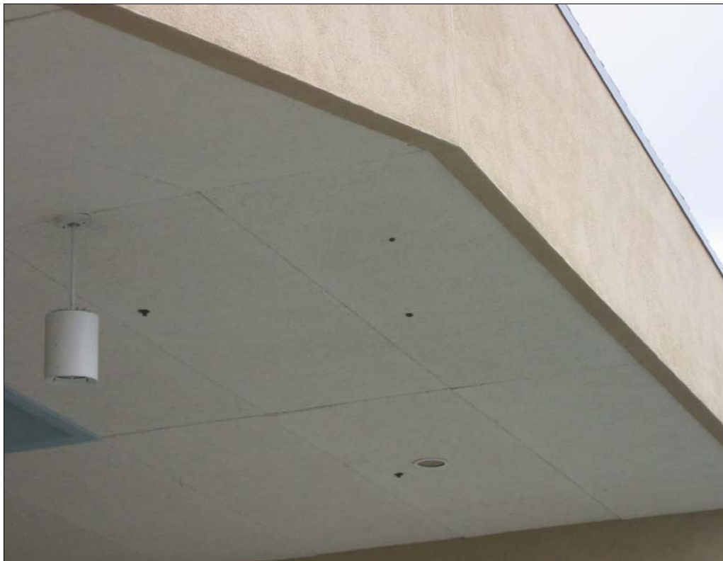
Tectum panels at Del Mar Elementary school in Morro Bay were observed to be coming loose under the soffit area.
