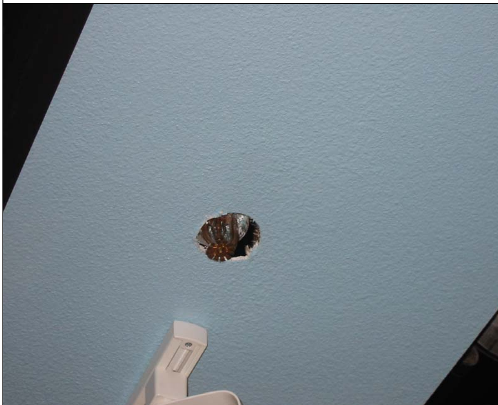
Sprinkler head finishing rings held in place by friction came off during the quake at Del Mar Elementary.
