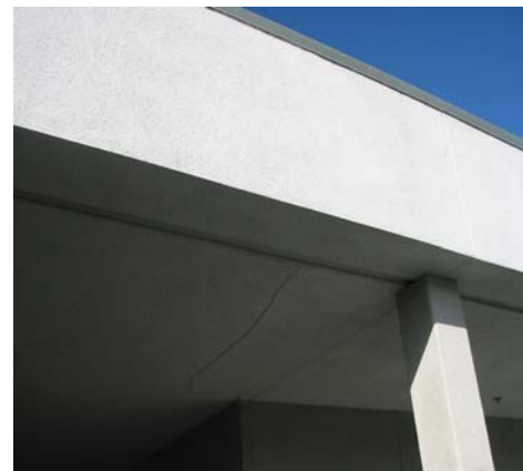
The joint at the addition to an existing building separated at San Luis Obispo High School. There was some evidence that this separation was pre-existing. The same building was observed to have loose roof tiles in need of repair.
