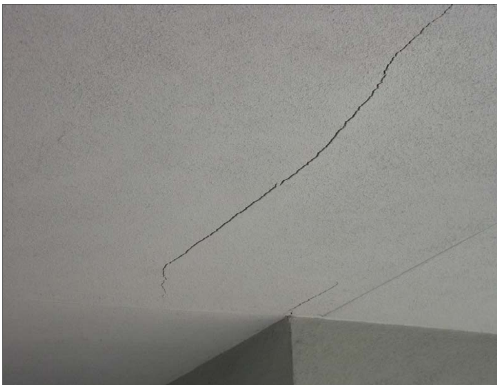
Plaster cracks at a re-entrant corner were observed at Los Ranchos Elementary School.
