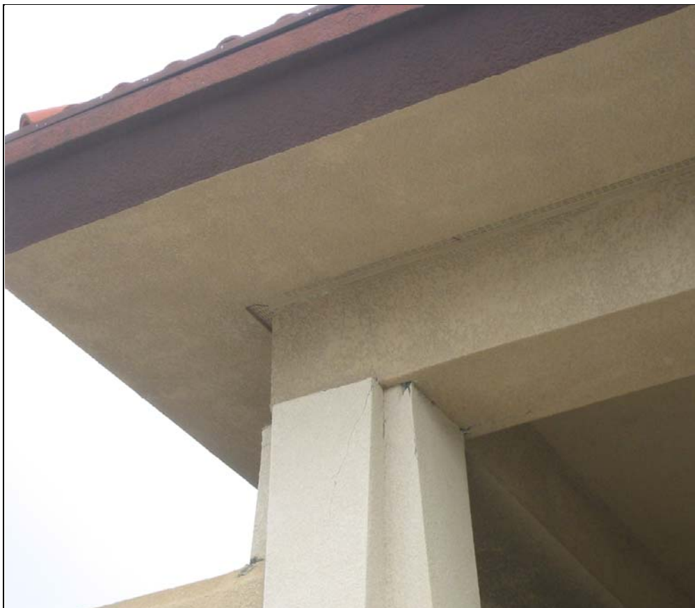
Cracking of the plaster assembly at the Paso Robles High School administration wing was observed
