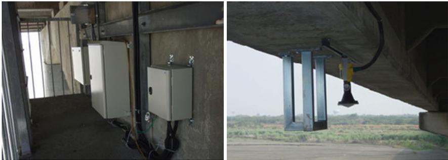
**Fig. 11.24** Completed installation of the CB box, power supply system, and the water level sensor
