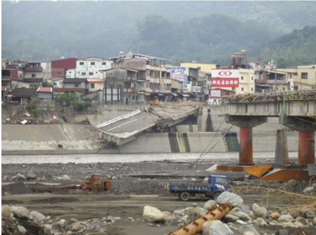
**Fig. 11.14** A bridge was failed by over-scale flood during Typhoon Morakot
