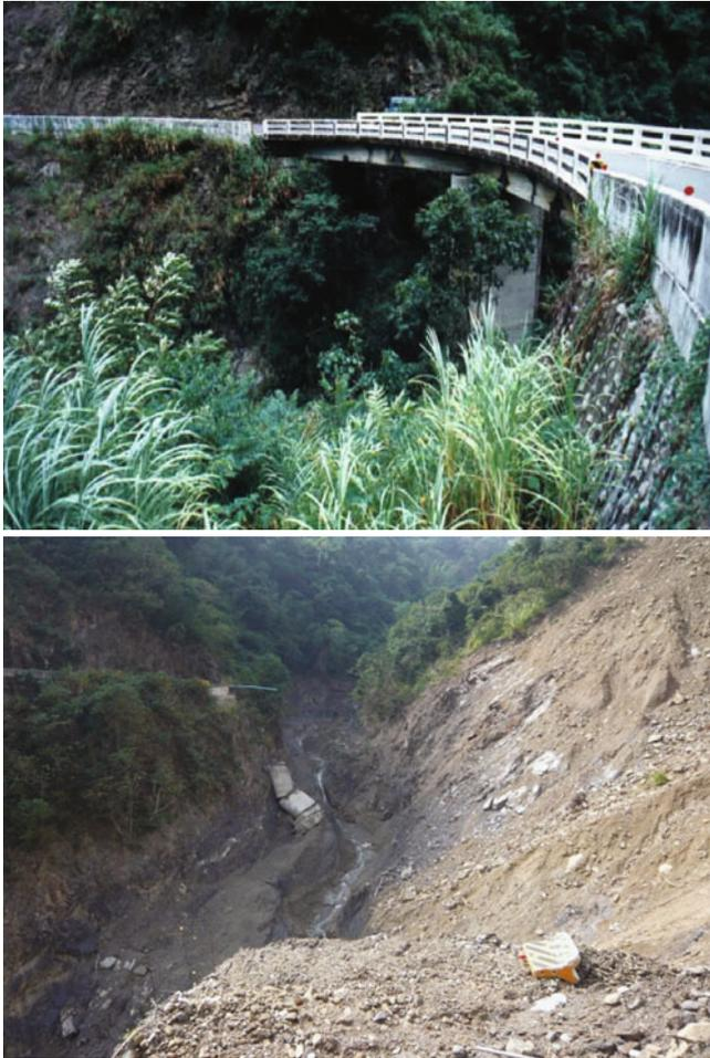
**Fig. 11.9** Before and after photo images of a bridge destroyed by Typhoon Morakot
