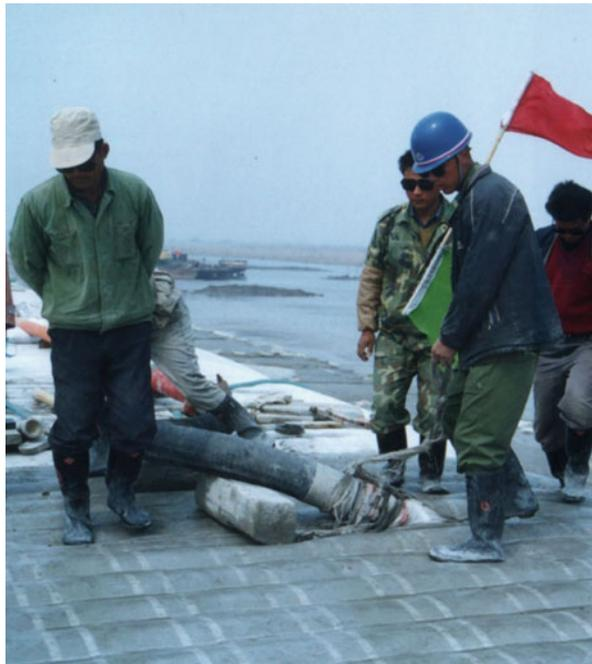
**Fig. 7.7** A concrete cover made of grouted geotextile mattress
