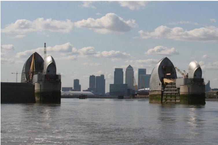
**Fig. 5.1** The Thames Barrier open to shipping, with one of the ten rotating gates closed (*on left hand side*), photograph © Scott Steedman
