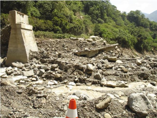
**Fig. 11.13** A bridge was failed by debris flow during Typhoon Morakot
