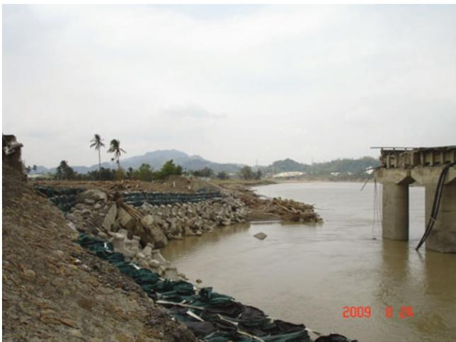
**Fig. 11.15** A bridge embankment and abutment were eroded away during Typhoon Morakot
