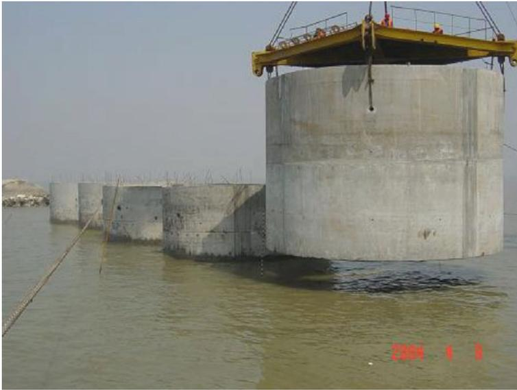
**Fig. 7.15** Installation of upper cylinders to form breakwater
