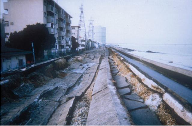
**Fig. 12.1** Liquefaction-induced subsidence of Yodo River Levee in Osaka after 1995 Kobe earthquake (Photo by Fudo Construction Company)
