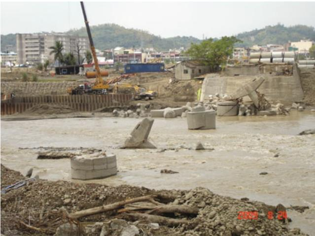
**Fig. 11.17** A bridge was failed by scour during Typhoon Morakot
