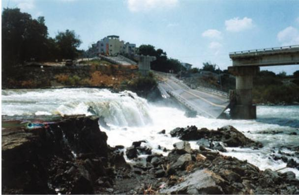
**Fig. 11.1** A bridge was damaged by fault rupture during Chi-Chi earthquake (provided by Professor Chen, Cheng-Hsin)
