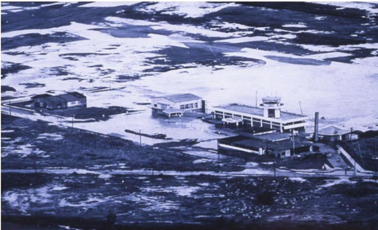
Fig. 12.15 Boiled water around Niigata Airport (air photograph taken by Mr. Yuminamochi immediately after the quake)
