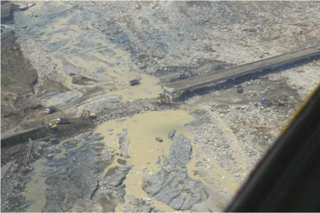
**Fig. 11.16** A bridge was failed by deep erosion of river flood during Typhoon Morakot
