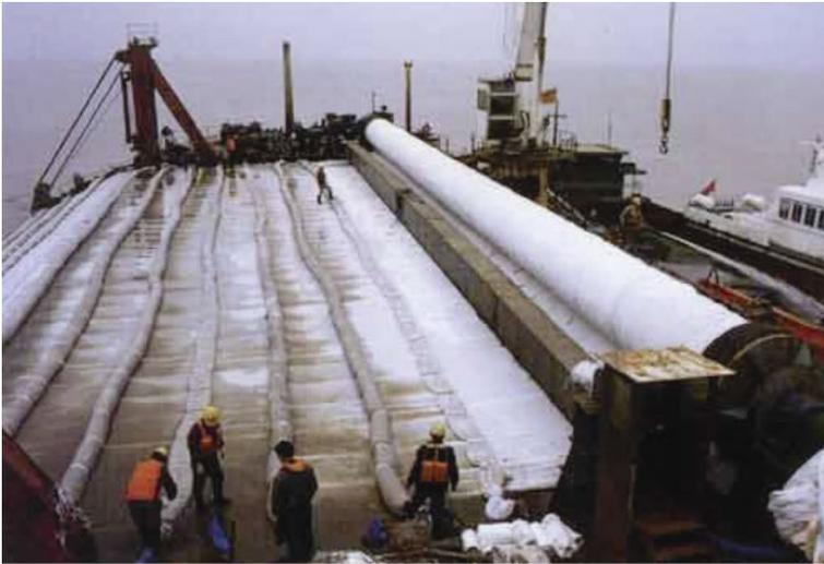
**Fig. 7.11** Placement of geotextile with sand filled geotextile tubes (after Yan et al., 2009)
