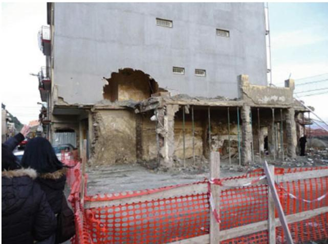
**Fig. 10.9** Scaletta Zanclea Village: a building damaged by the debris flow flowing in the Racinazzi stream
