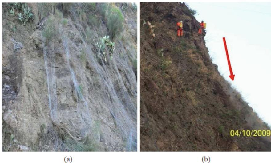
**Fig. 10.29** Stabilization of the slope reported in Fig. 10.26: (a) old stabilization works; (b) new stabilization works
