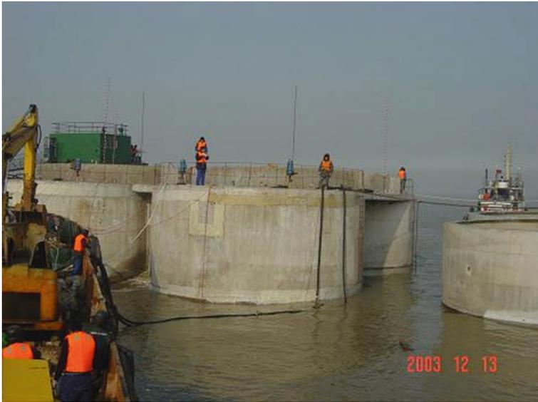
**Fig. 7.14** Installation of concrete suction caissons
