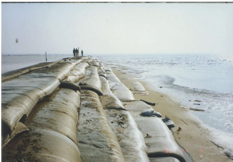
Fig. 7.6 A picture showing the formation of a dike using clay slurry filled geotextile bags
