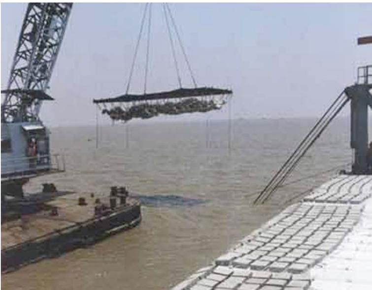
**Fig. 7.12** Installation of the geotextile and concrete block composite (after Yan et al., 2009)
