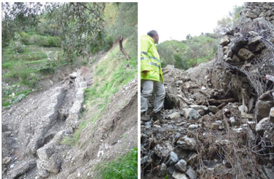
**Fig. 10.17** The damage occurred to gabions along the Sopra Urno stream
