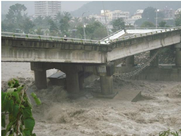
**Fig. 11.2** A bridge was damaged by progressive scour during 2009 Typhoon Sinlock
