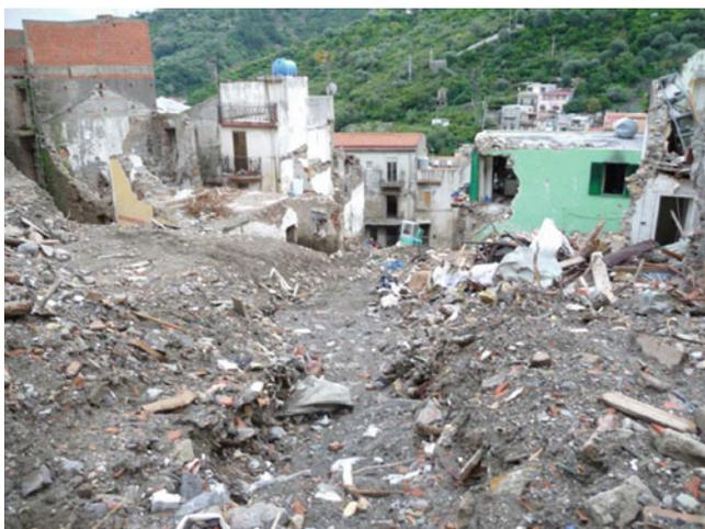
**Fig. 10.15** Damaged houses due to the landslide occurred at Puntale stream. The debris flow reached the third floor of the house in front of the stream
