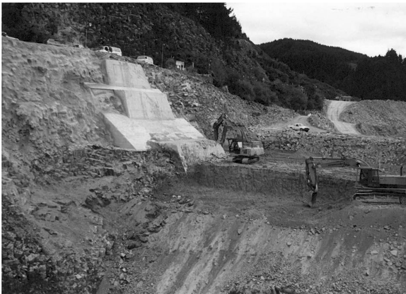
(b) Photograph of abutment showing slope correction concrete
