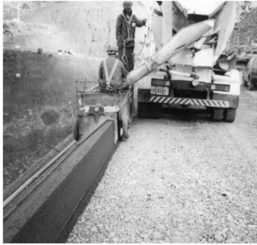
Figure 15.31 Extruded kerb construction for the upstream face (Cruz et al. , 2009).
