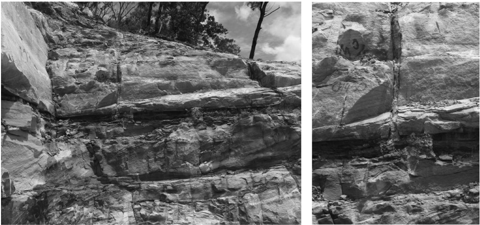
Figure 3.22b Photographs of the abutment of Shannon Creek Dam, showing in-filled stress relief joints. The joints are up to 80 mm wide and terminate on shale beds. Photographs courtesy of L McDonald and Clarence Valley Council.
