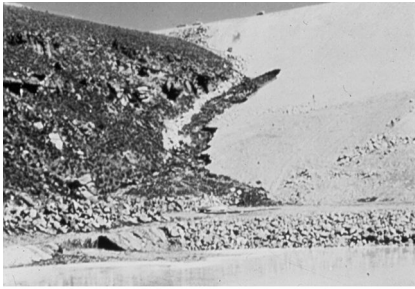
(a) Concentrated leak and pipe at 10:45 am
