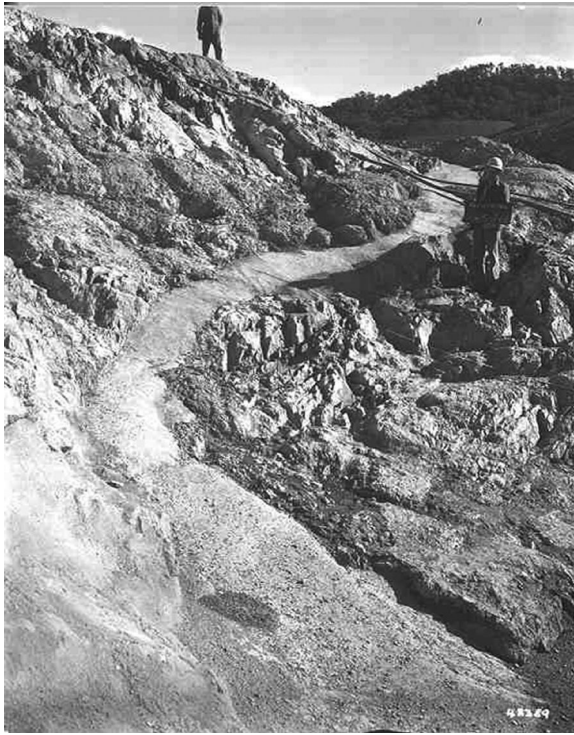
Figure 17.8 Left abutment of Blowering Dam after treatment of large fault zone and weathered seam (courtesy of Snowy Hydro).
