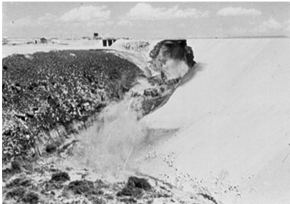
(c) Breach nearly developed at 11:55 am
