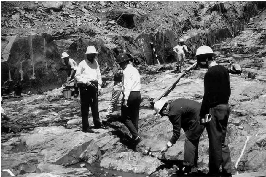
Figure 17.19 Middle River Dam – foundation cleanup in progress.
