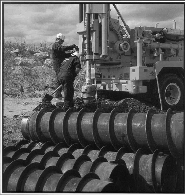
Figure 5.13 Large diameter hollow auger drill rig (courtesy CMEC).
