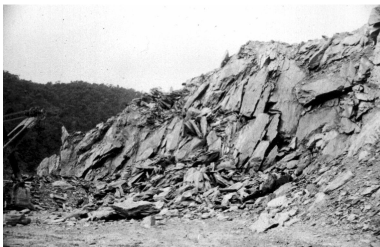
Figure 3.14 Schist being quarried in the spillway excavation at Kangaroo Creek Dam. Note the platy shapes of the rock fragments.
