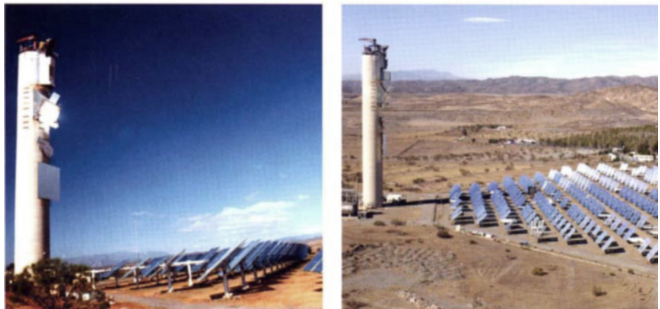
Figure 6.12. Solar tower test installations in Almería, southern Spain. Source: Stefan Franzen, CIEMAT
