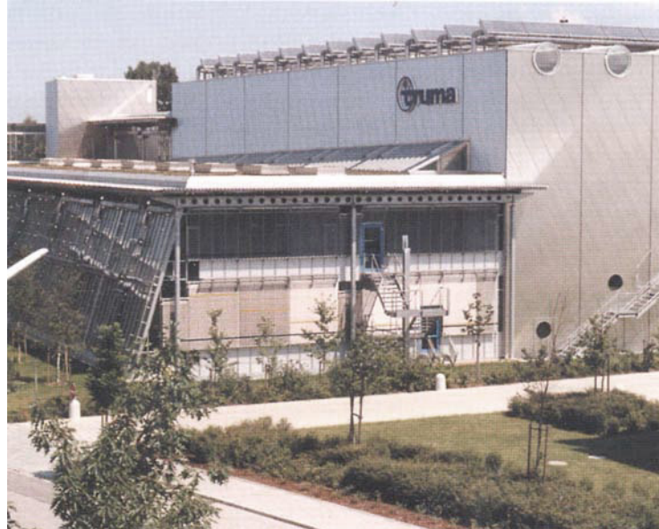
Figure 8.4. Air collectors placed on stands on the roof of a factory building. Source: Grammer, Amberg
