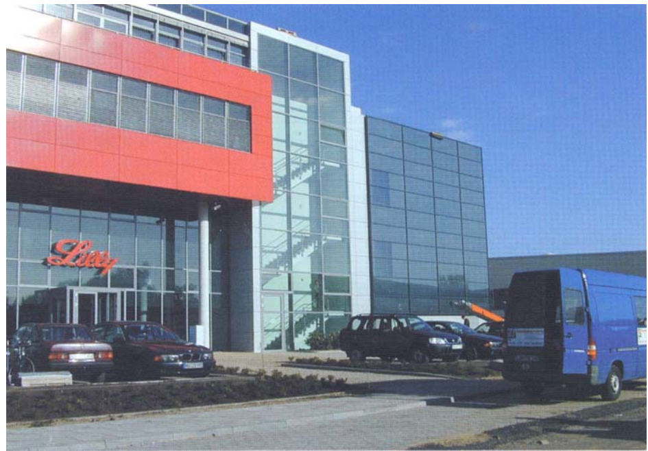
Figure 8.10. Solar air collector on the façade. Source: Grammer, Amberg
