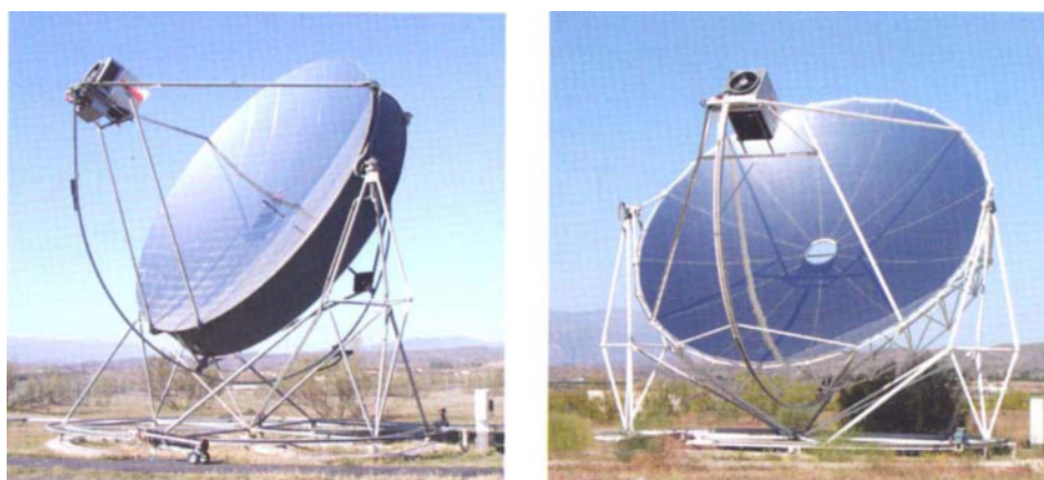
Figure 6.15. Dish/Stirling demonstration systems in Almeria, Southern Spain. Source: Volker Quaschnig
