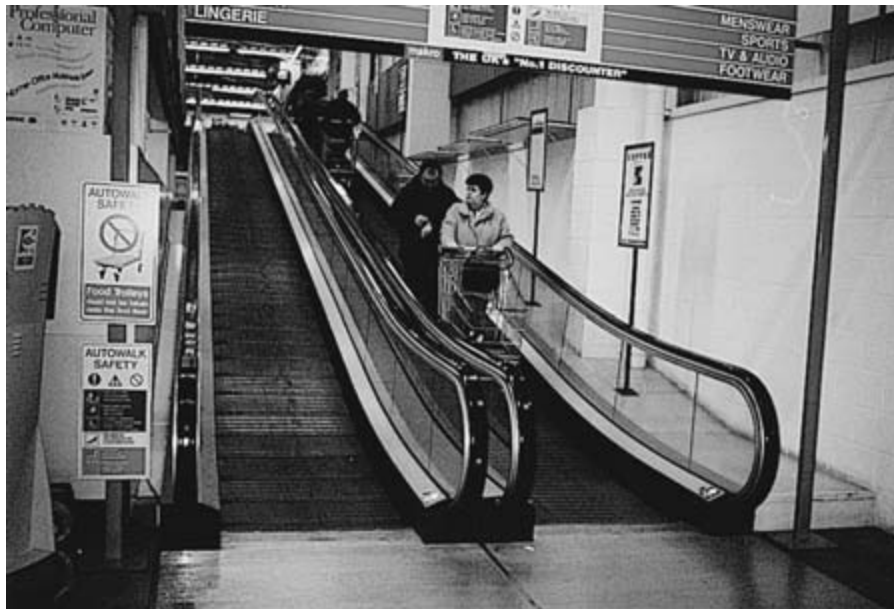
Figure 4.39 Where a travelator is inclined the gradient should be low to allow easy and safe access.
