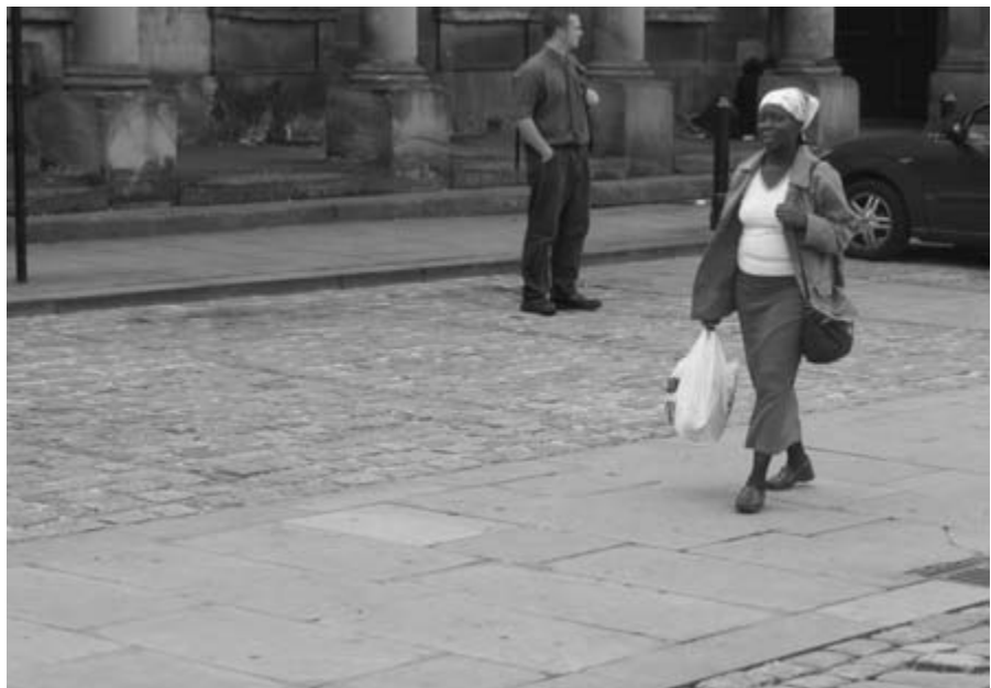
Figure 4.8 A smooth path can be laid across an uneven surface to provide an accessible route.
