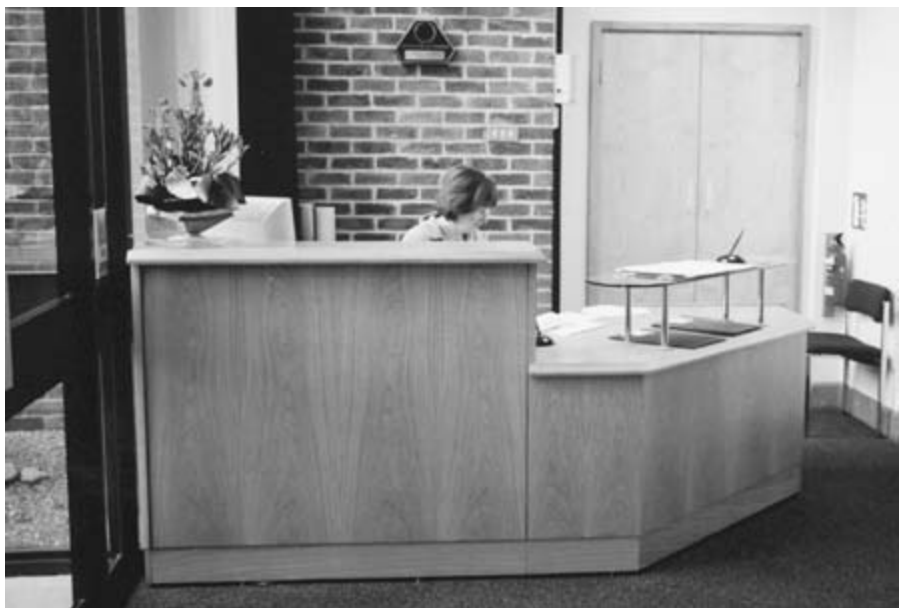
Figure 4.27 This desk has a low section – but the writing shelf and the lack of knee space would prevent easy use by a wheelchair user.
