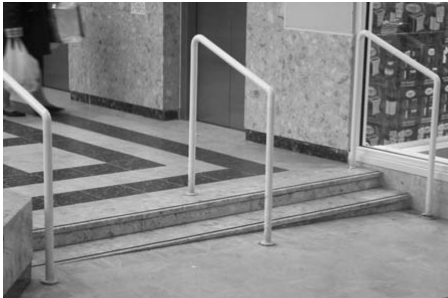
Figure 4.19 Tapered risers can present a serious tripping hazard and should be avoided.
