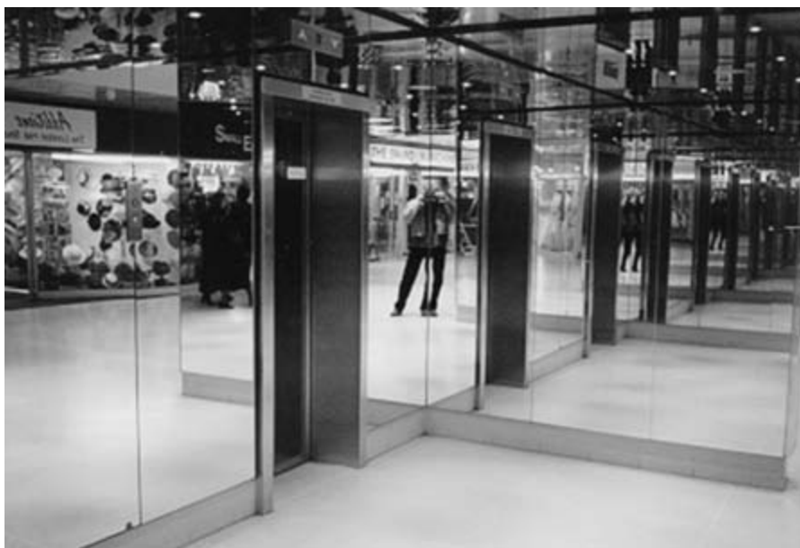
Figure 4.29 How many doors are there? Reflective finishes can be very confusing for someone with poor vision.
