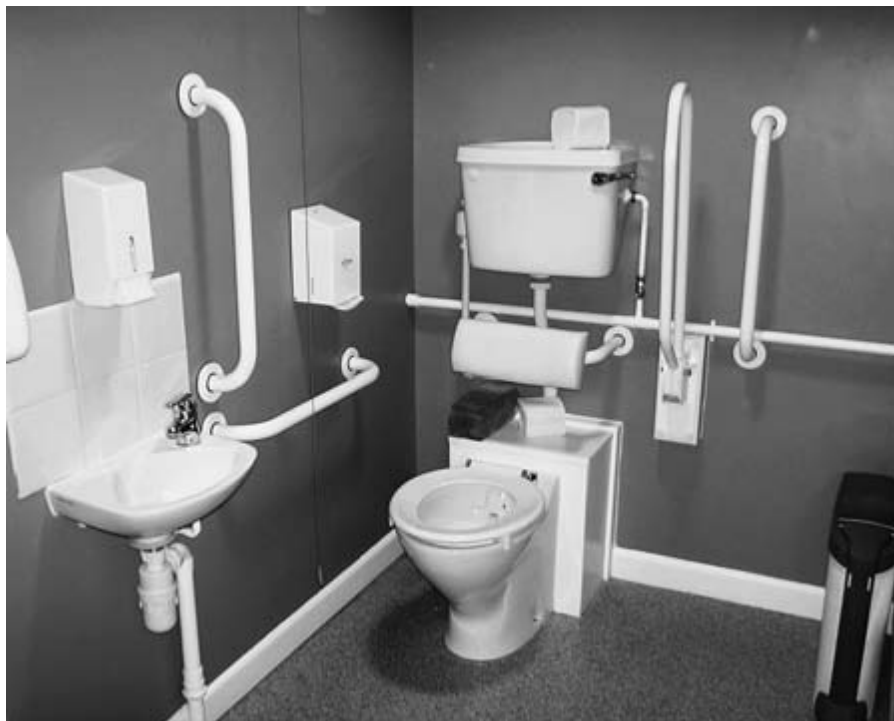
Figure 4.44 Good use of contrast ensures that fittings are visible, though position of bin reduces area available for side transfer.
