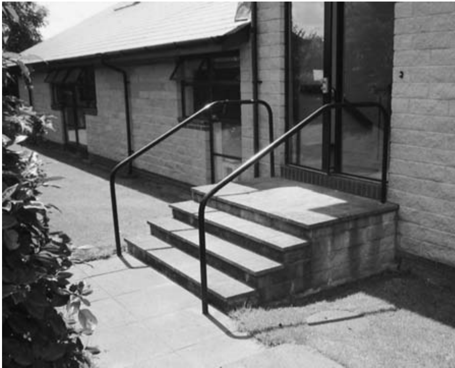
Figure 4.66 Assisting disabled people out of the building using a fire exit with external steps presents management issues that simply cannot be addressed by an ad hoc escape policy.
