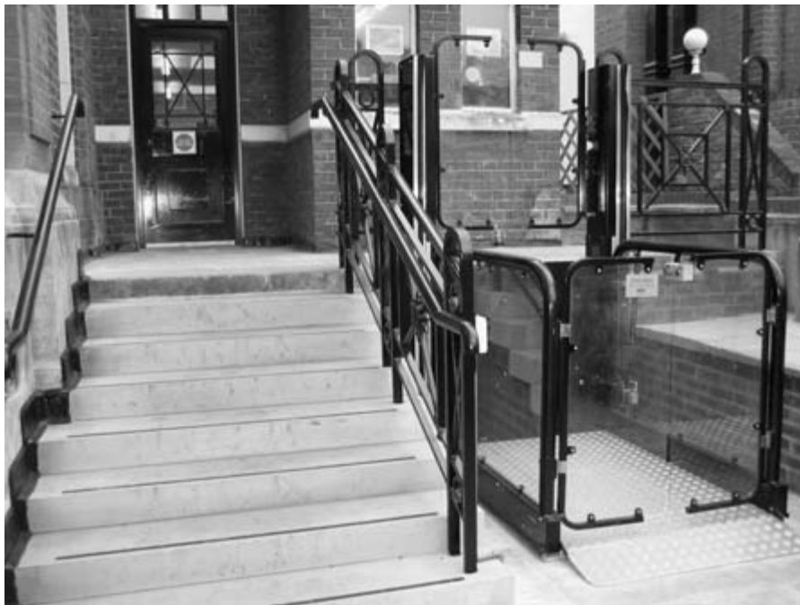
Figure 4.41 A vertical platform lift can be added to an existing building to help provide equal access to services.
