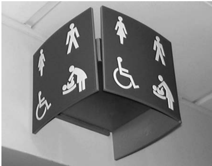
Figure 4.45 Projecting signage allows people to identify the position of a toilet from a distance, important for people who experience incontinence. This sign shows good use of colour contrast and symbols and, importantly, all the facilities are located in the same area.
