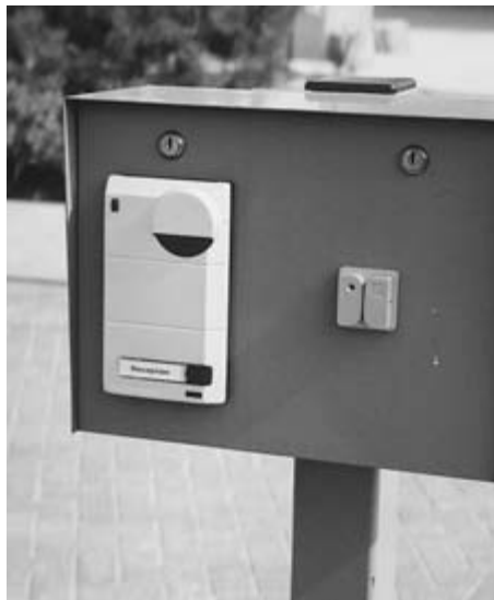
Figure 4.26 This car park control requires reach, dexterity, speech, hearing, and a right arm. It is possible to hold a driver's licence without one or more of the above but you need all of them if you wish to enter this car park. Is this reasonable provision?
