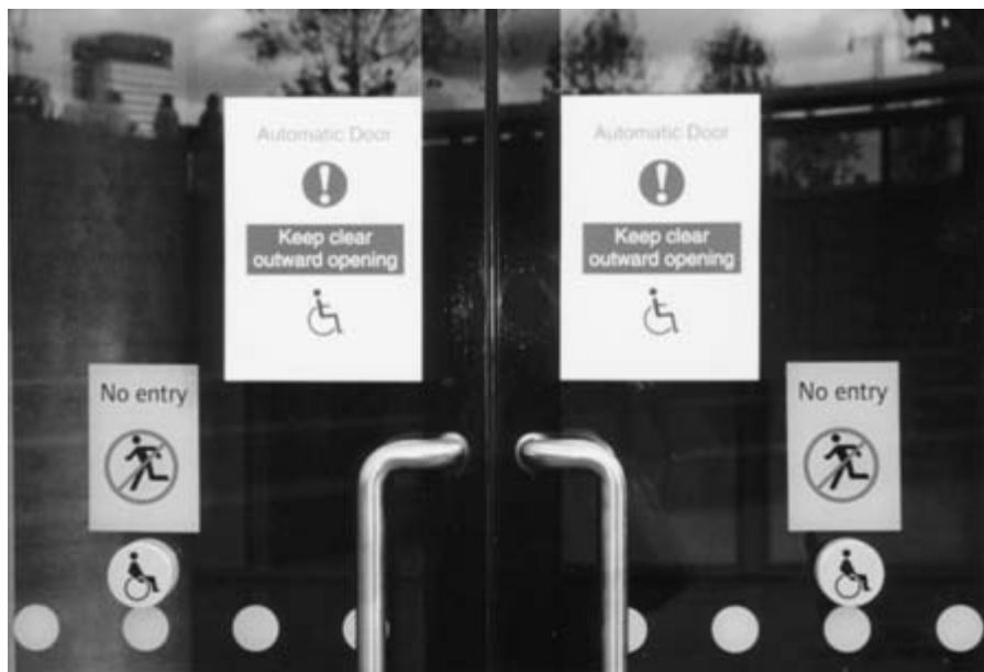
Figure 4.56 Signs should be clear and easy to understand. Too many signs can cause confusion. Effective, ongoing management of signage is essential.
