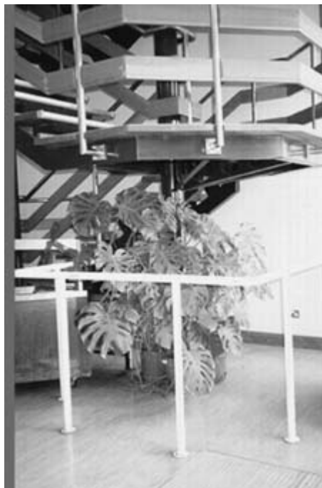
Figure 4.36 The area below overhanging stairs should be guarded.
