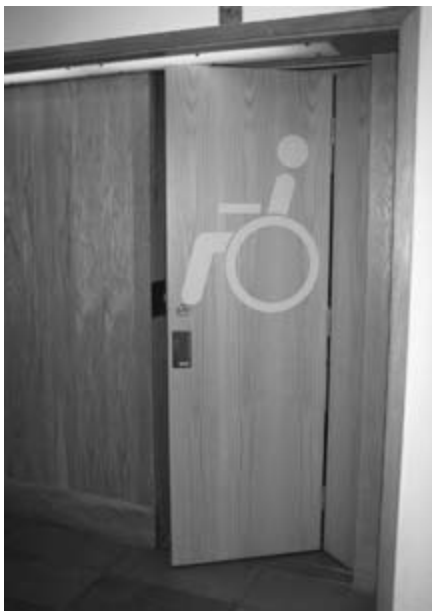
Figure 4.51 Bi-fold doors can be used to avoid obstructing corridors.
