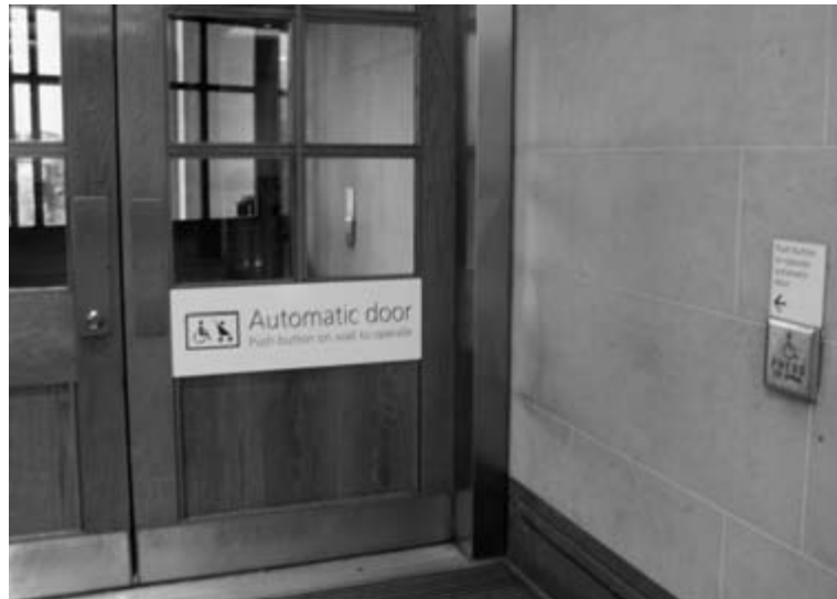
Figure 3.4 Adding automatic opening to doors can make access more convenient and help a service provider fulfil their duties under the DDA.
