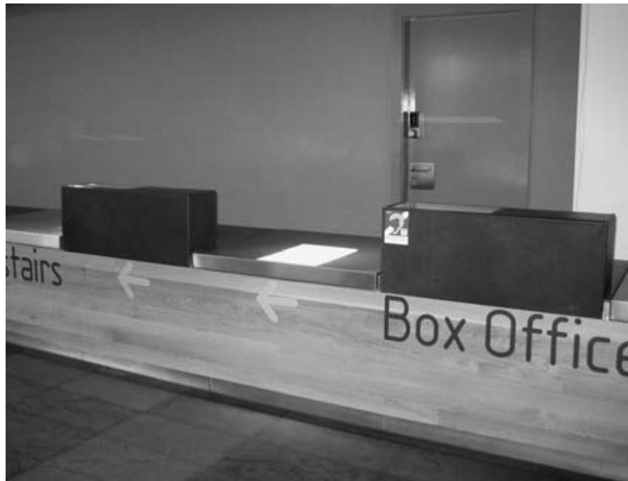
Figure 4.53 A low counter, fitted with an induction loop, can help provide easy access.
