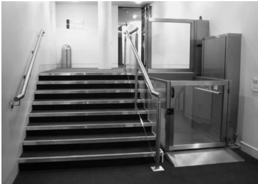
Figure 2.2 Refurbishment can offer opportunities for improving access, such as adding a lift to a change of level.
