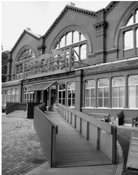
Figure 1.4 A ramp may be provided as a short-term solution while awaiting a major refurbishment of the building.
