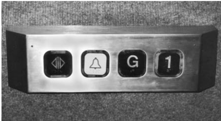
Figure 4.42 Lift buttons located horizontally can be easier to reach.
