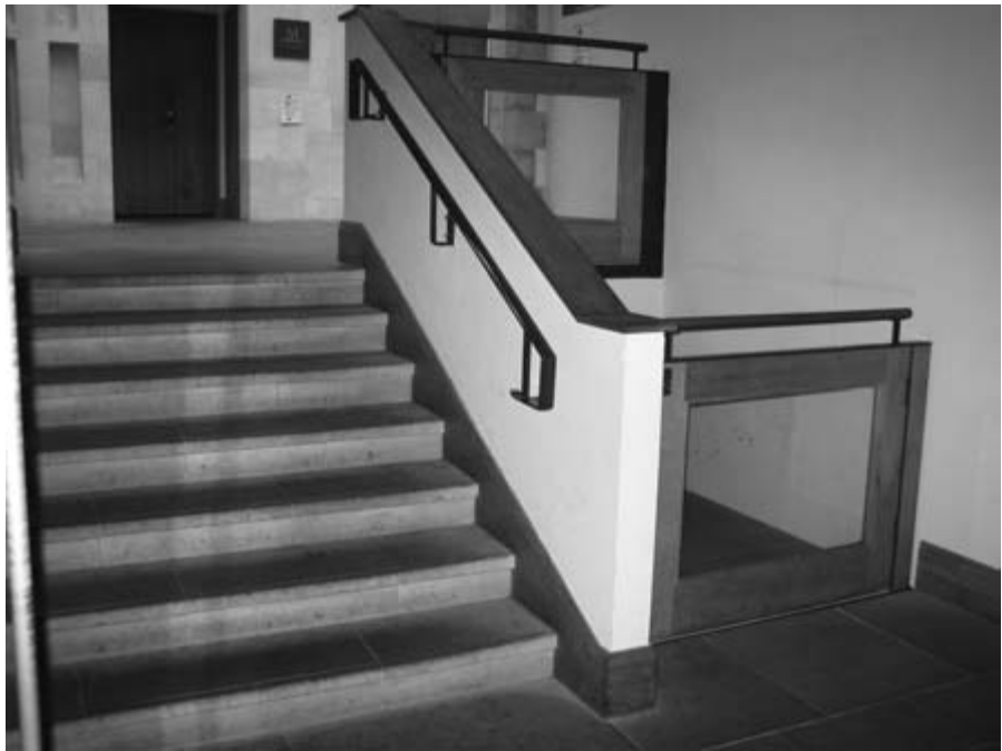
Figure 4.40 When a vertical platform lift is provided it should be adjacent to the stair with which it is associated.
