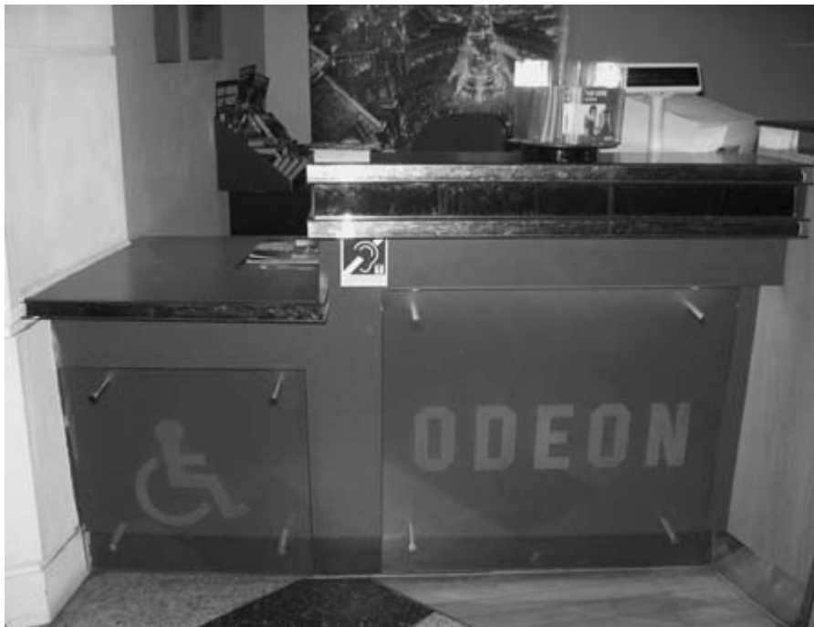
Figure 3.1 A low ticket desk can help a service provider fulfil their duties under the DDA.
