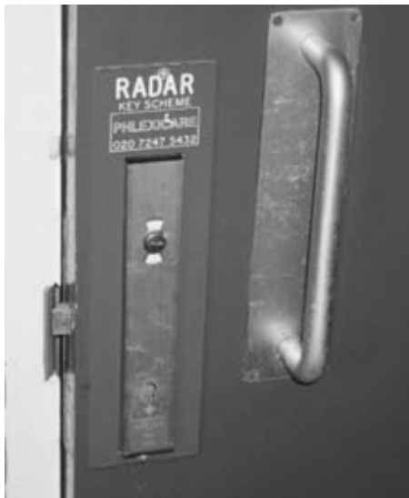
Figure 4.47 The RADAR KEY SCHEME is used to prevent the use of accessible WC facilities by non-disabled people.
