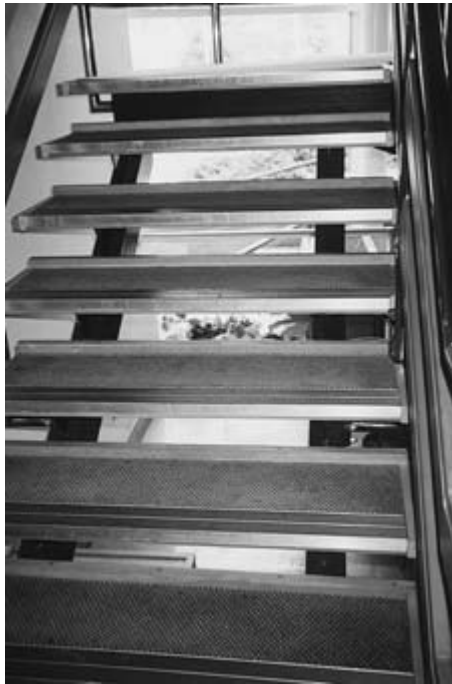
Figure 4.34 Open risers should always be avoided; they can be visually confusing and catch toes, sticks, callipers, etc.
