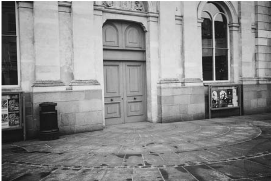
Figure 4.18 Gently ramping a section of pavement can overcome a change of level at an entrance.
