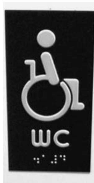
Figure 4.60 The use of the letters WC indicates this is an accessible toilet. Using the symbol without the letters may suggest to some people that this an area related to disability, but not necessarily a toilet.
