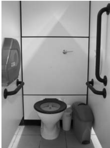
Figure 4.43 WC compartments fitted for use by ambulant disabled people should always be provided.
