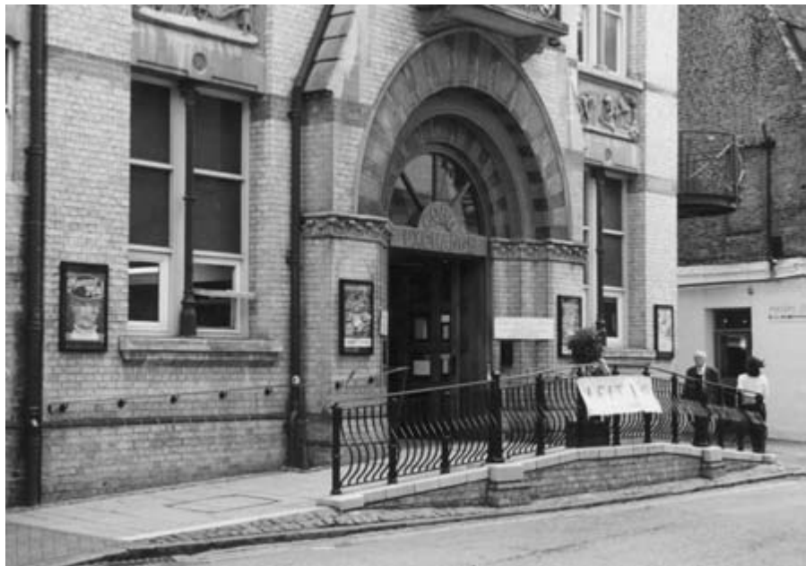
Figure 3.8 A change of level at the entrance to a building can be overcome by ramping the pavement.
