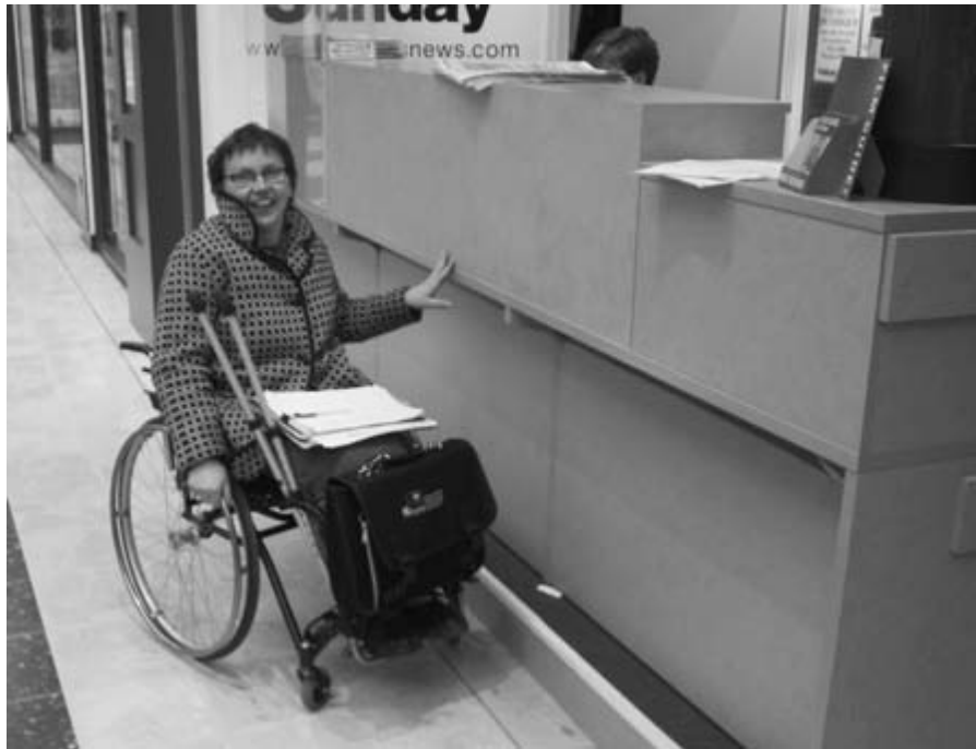
Figure 4.52 Counters should allow communication at seated and standing heights. A low counter or low section will allow wheelchair users to communicate with staff or customers. Seats should be provided to both staff and customer side.
