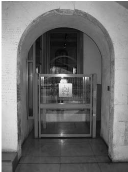
Figure 4.21 A platform lift added beside a stepped change of level at the entrance of a historic building can improve access.
