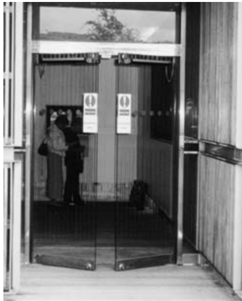
Figure 4.23 Automatic swing doors should be clearly signed and the swing area protected.
