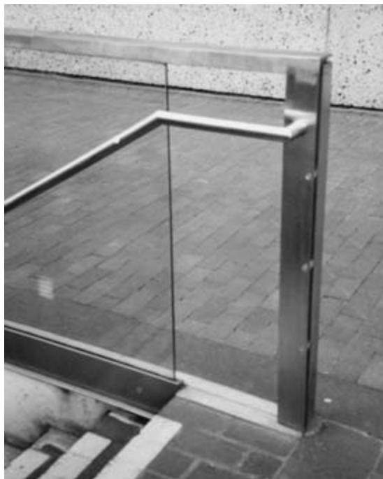
Figure 4.20 The horizontal extension of a handrail can provide support and also information on the start and finish of the flight of stairs.
