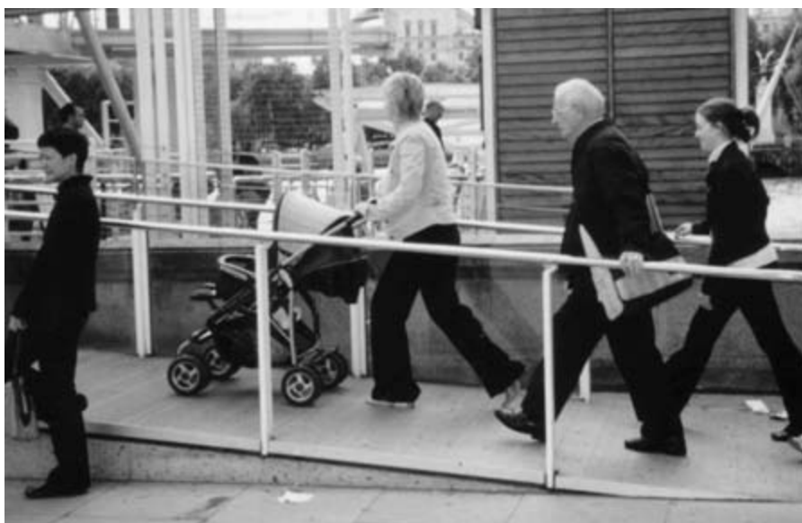
Figure 4.17 All ramps should have appropriately designed handrails.
