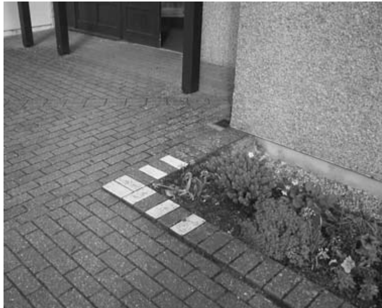
Figure 4.11 Potential tripping hazards should be highlighted using visual contrast.
