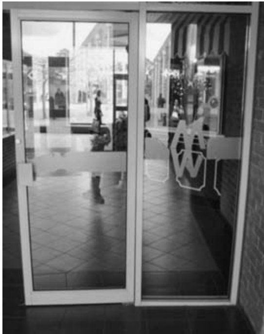
Figure 4.33 Is the manifestation adequately contrasted against its background at all times?
