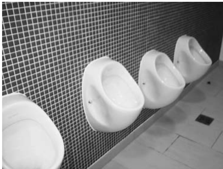
Figure 4.50 Not all disabled people use accessible toilets; some will use the standard toilet accommodation. The need for good design, colour contrast and appropriate fittings is also important here. Children should also be considered.
