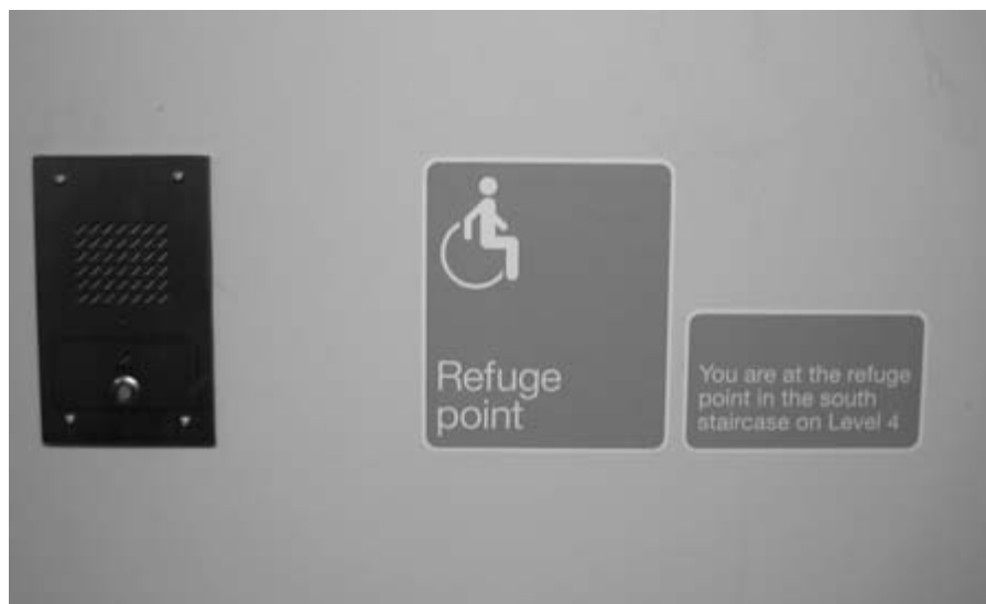
Figure 4.63 Refuges should be clearly identified and a system of communication provided.
