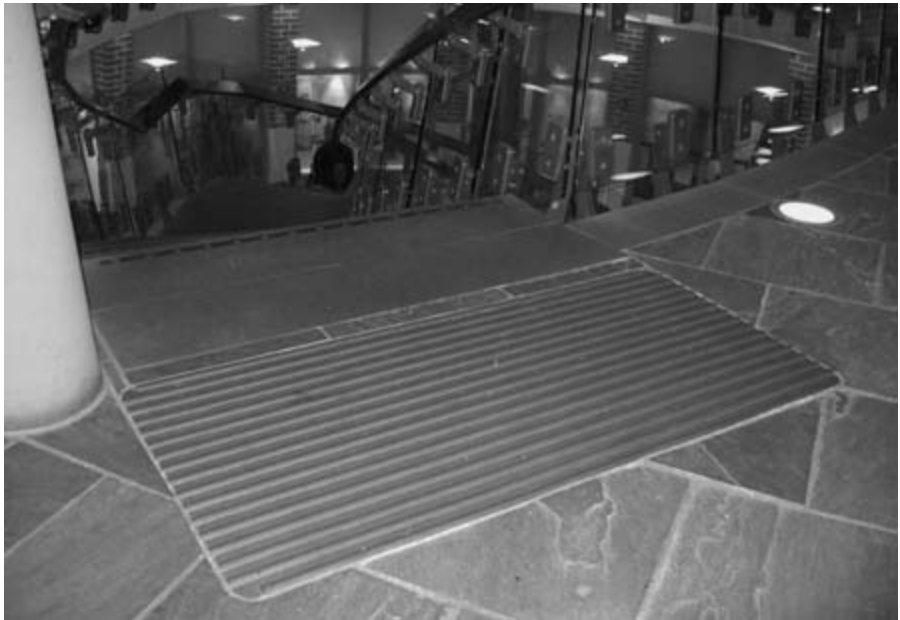
Figure 4.38 Tactile hazard warning can alert people to the presence of a stair.
