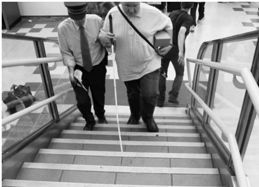
Figure 4.35 Each step nosing should contrast visually with the remainder of the tread and should be clearly visible when ascending and descending stairs.
