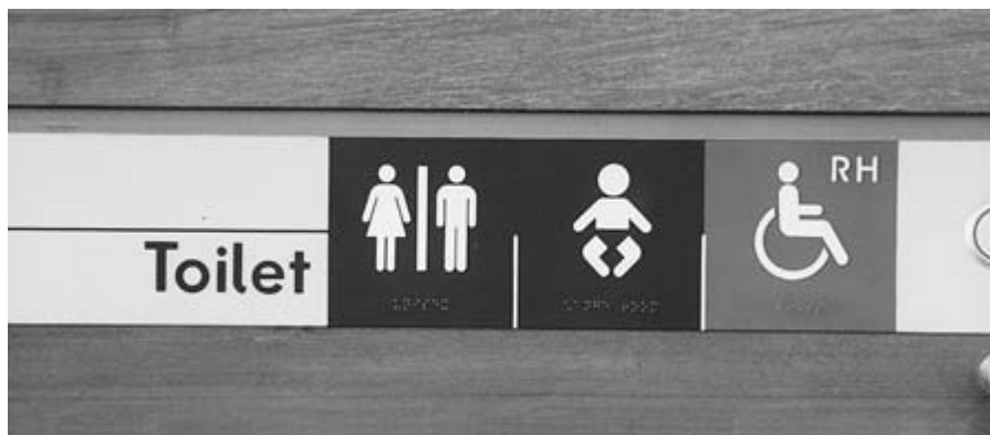
Figure 4.46 A clear sign with good use of colour, symbols and text. The RH identifies to a disabled person that this is a right-hand transfer toilet. This is very useful information, easily provided.
