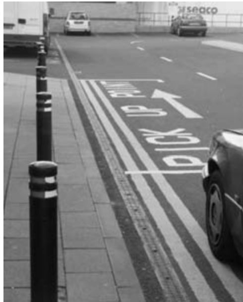
Figure 4.5 Setting down and pick-up points should be clearly marked with dropped kerbs. Care should be taken to ensure bollards do not obstruct routes.
