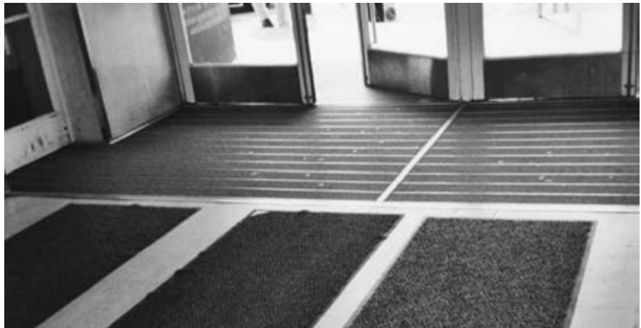
Figure 4.24 Good use of fixed mats – but loose mats represent a serious tripping hazard.
