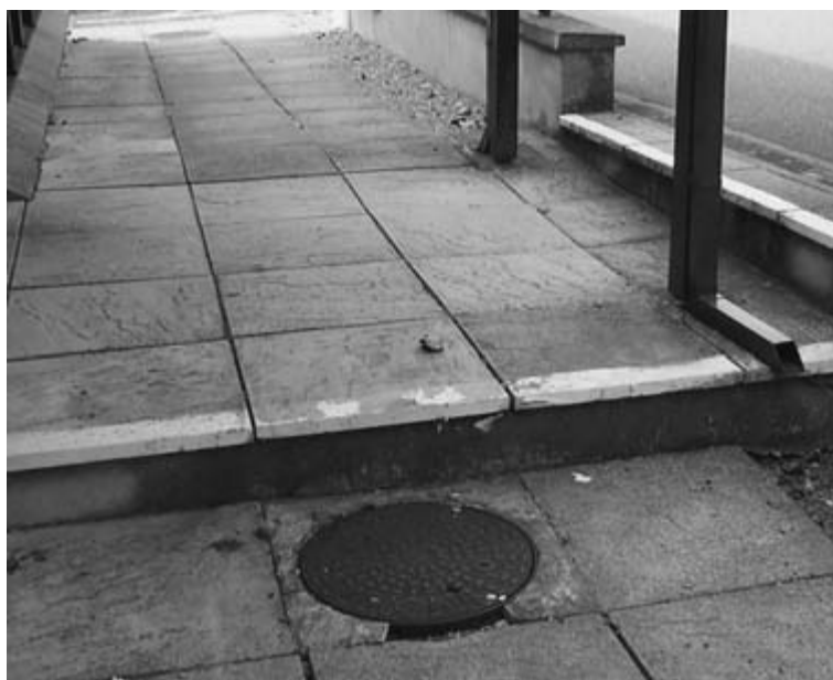
Figure 2.3 Once a nosing is painted, a commitment is made to re-inspection, repair or redecoration/replacement. The implications in terms of duties and obligations under the DDA should be considered for all access issues.
