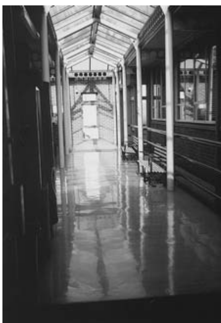
Figure 4.30 Many people would find this floor finish disconcerting, but especially those with poor vision, older people and people using mobility aids such as crutches. It may not be the selection of the floor covering that is the problem, but the way it is being cleaned and the impact of daylight and artificial lighting.
