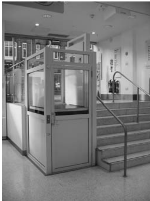
Figure 3.2 A platform lift can be used to overcome a physical feature such as a stepped change of level.
