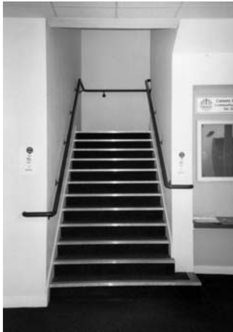
Figure 4.37 Contrasting nosings and well-designed handrails can help people use stairs.
