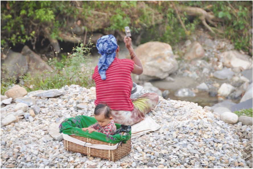
Photo 1 A mother with child making gravel for road construction by hammering larger rocks to make smaller rocks along the Marsyangdi Highway. This is a common sight along many road construction alignments in Nepal (R.E. Beazley 2019).
