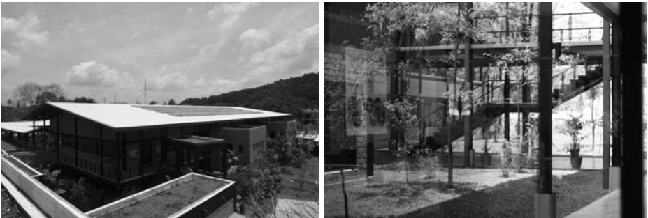
Figure 5.8 An LEED Platinum certified building in warm, humid climates, with cool and green roofs and shading by vegetation
